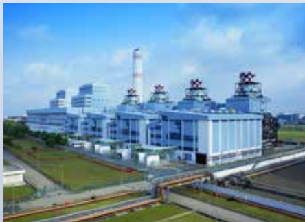
Fabric material replacement for an expansion joint on a MHI 701F gas turbine exhaust at a Combined Cycle Power Plant in Singapore.
