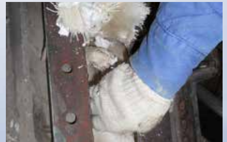
1. Removal of A-style expansion joint including external and internal insulation, wire mesh, back-up flanges and pre-bolster.
