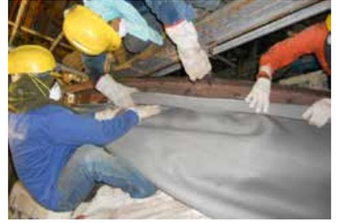
Fabric material replacement for an expansion joint on a MHI 701F gas turbine exhaust at a Combined Cycle Power Plant in China. These durable fabric replacements have lasted 6 years in service with 1 200 cycles on 9 units.
