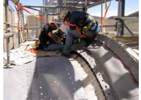
Replacement of fabric belt on a Siemens 501F series gas turbine. EagleBurgmann offers complete turnkey installation, inspection, and emergency services for fabric, metal and rubber expansion joints.
