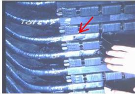
Photo 7. Huge 2-5/8" separation after 19 months operation, 11 mils/load cycle. Separation is inside the core due to high power factor load.
