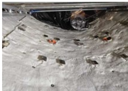
4. Inner insulation at the exhaust diffuser consists of a 4 × 1 in. layer of needed silicate fiber mats held in place securely with washers on the pins
