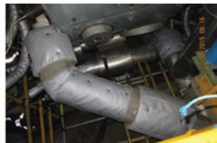
3. Old-design piping insulation with sheet-metal cover is at left; new flexible insulation design is at right. Time for dismantling/reassembly for the old design was about seven hours, with flexible insulation only 20 minutes
