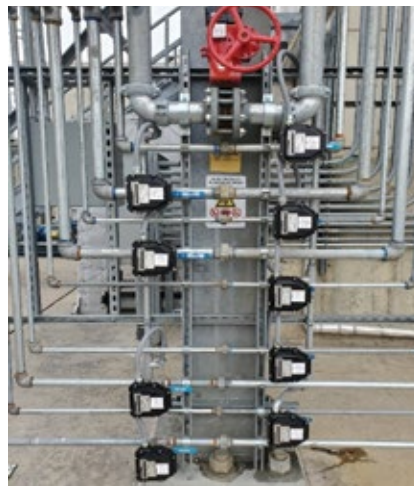
5. Automatic solenoid zone valves were not easily disabled or isolated (left)
