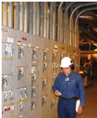
480-V switchgear—150 amps one side; 200 amps other side
