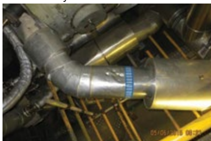
3. Old-design piping insulation with sheet-metal cover is at left; new flexible insulation design is at right. Time for dismantling/reassembly for the old design was about seven hours, with flexible insulation only 20 minutes
