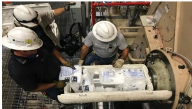
2. Specialty tooling required to replace the exciter field was made in-house (left)
