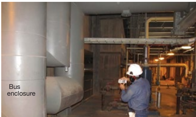
Isolated phase bus—21 kV, 8k amps
