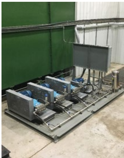
1. Wet compression skid includes high-pressure pumps, PLC panel, and tubing for delivering water to the gas-turbine air inlet duct
