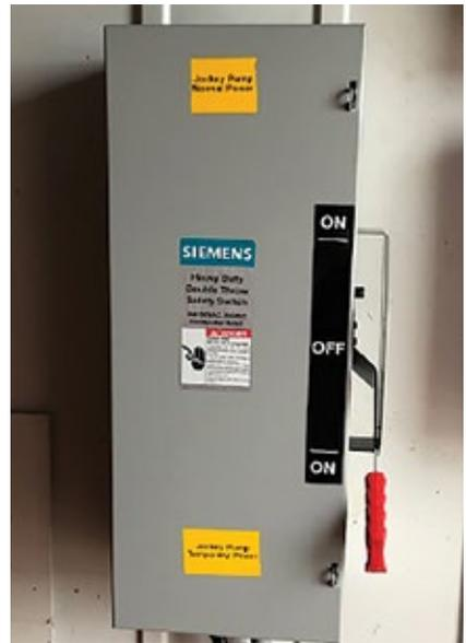
2. Selector switch transfers electric supply for the jockey pump from station service to an alternative source connected to the welding receptacle
