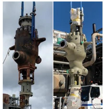
**9. Digital valve replacement** at right eliminates the need for upgrades to internal parts and the valve casing at left made necessary by solid particle erosion
