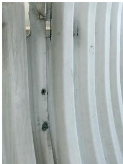
**1. Original stacks** were made of molded fiberglass, with sections bolted together on the inside
