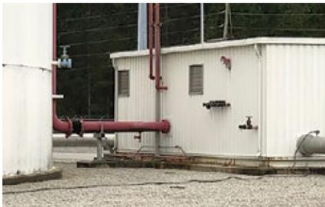
3. Jumper cable supplies a secondary source of power to the jockey pump when station service is not available
