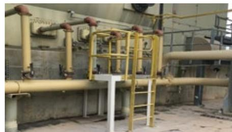
**2. Staff-designed platform** provides access to level switch without need for a ladder
