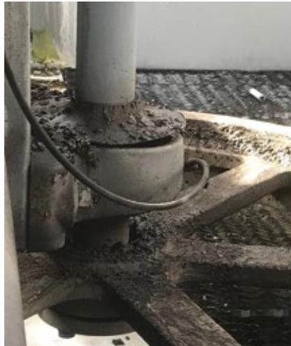
7. Grease is supplied to the bearings (lower at left, upper at right) via flexible hose
