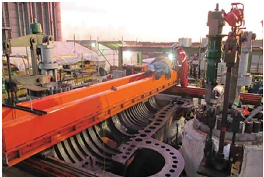
**3. Portable mill set-up** on the horizontal joint helped to correct casing distortion
