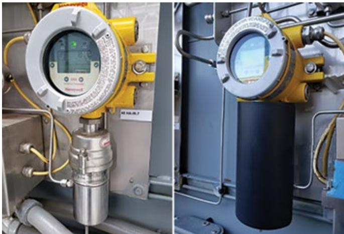
5. Sensor with factory-supplied stainless-steel cover is at left; with plastic shield over the steel cover at right
