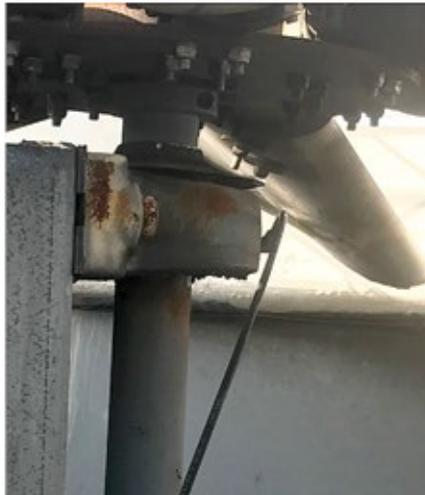
OEM's single-piece bearings and opted for using slightly more expensive split bearings of the same rating, which would not require fan removal. Another benefit of the split design: Less time to replace a bearing by a factor of four—4 hours versus 16 for the original.
