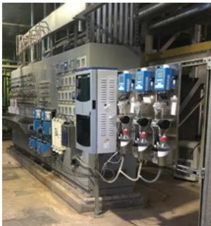
**1. Upgraded and expanded panel/ instrumentation underpins the KPI index developed for tighter control of water chemistry**
