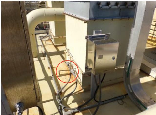
**2. Haz-gas detectors** (left photo) can be accessed from the compartment roof (circle in photo at right) where the analysis equipment is located
