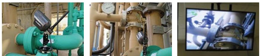
**Wireless camera**, magnetically attached to piping (left) points to lube-oil flange guards (center). Screen view is at right
