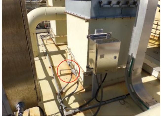
**2. Haz-gas detectors** (left photo) can be accessed from the compartment roof (circle in photo at right) where the analysis equipment is located
