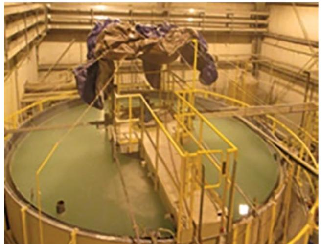
4. Access provided by the catwalk is in evidence here. The tarp is used to cover the clarifier during annual high-pressure cleanings to capture fugitive dust and debris
