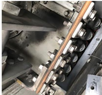
**1. The busbar location** where the power cables to the brush rigging are bolted is directly above the intake filters
