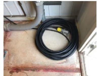
4. Jumper cable is ready for rapid-deployment in the event of a sudden loss in station service power
