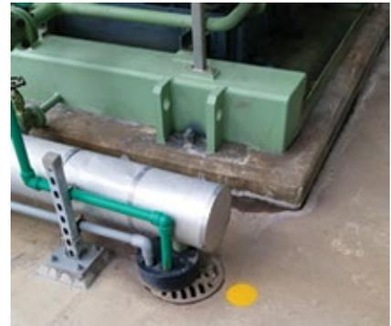
**8. Drains have color circle to identify the sump to which is connected**
