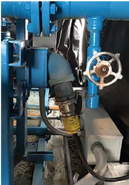
1. When the station-service transformer is out of service, power is supplied to the jockey pump from an alternative source via the welding receptacle
