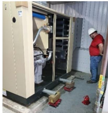
**8. The new compressor, 89 × 54 × 76 in. high and weighing nearly 5500 lb, is lifted (left) to allow the placement of four caster rollers (right) for maneuverability**
