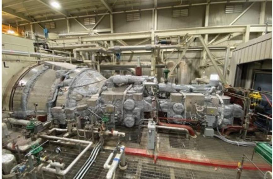
**10. Upgraded insulation system** mitigates the thermal fatigue of steam turbine’s critical parts and enables longer intervals between maintenance outages
