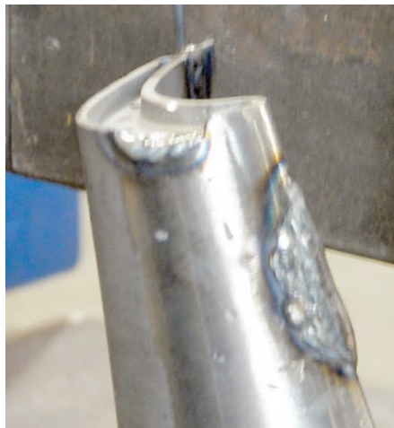
5-2. Temperature control of the repair process is critical for achieving desired results
