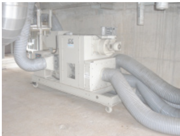
9, 10. Steam turbine has a separate dehumidifier (left) which is located external to the unit (right)
