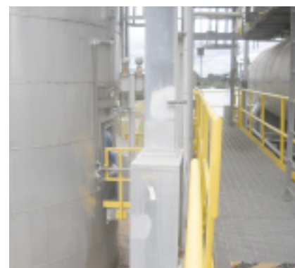
6. Duct balloon is simple to install through manhole accessible from catwalk
