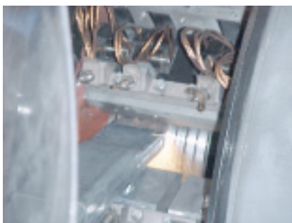
8. Online truing , also known as ston-ing, essentially “grinds out” brush vibration
