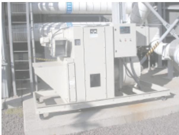
7, 8. Dehumidifier located outside the HRSG casing (left) works as illustrated at right
