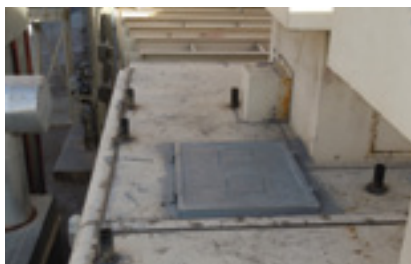
12. Roof hatch facilitates confined-space rescue
