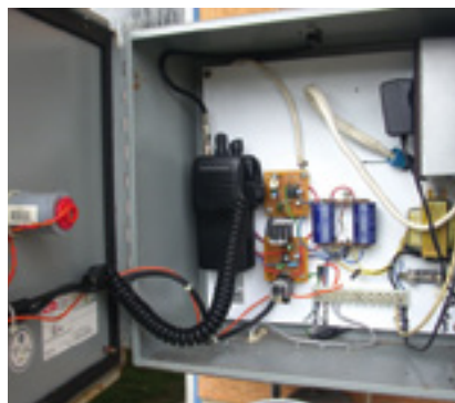
5, 6. Plant employees can allow visitors to enter the plant using their radios. A radio with tone receiver module in the gate control panel activates a relay to open the gate
