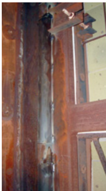
5. Steel baffles were installed to prevent exhaust gas from bypassing around the catalyst grid
