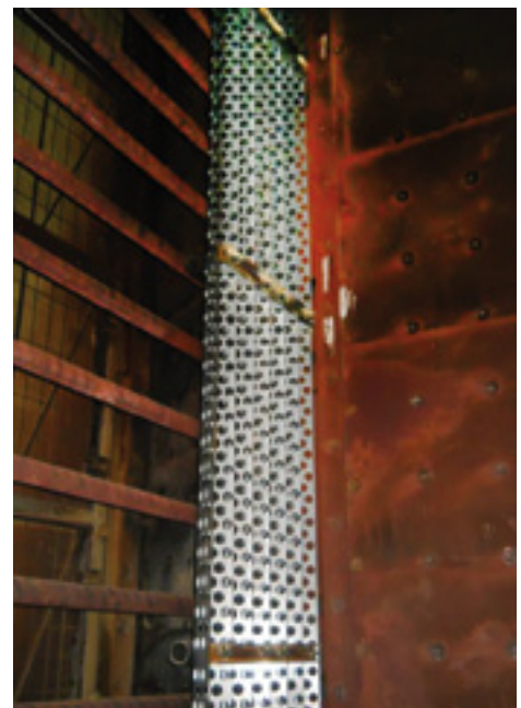
6. Perforated flow restrictor reduces exhaust-gas velocity close to the side wall, with minimal impact on backpressure
