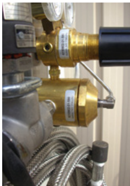
12. Key components in the Fig 9 system are the high-flow dome-type regulator and 0.75-in.-diam, high-pressure, stainless steel piping and hose. Piping is Schedule 80 (left)
