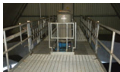
4. Gearbox for each ACC fan contains about 8 gal of oil
