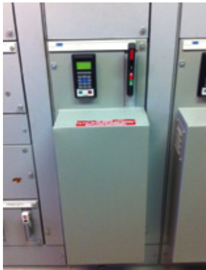
18. MCC modifications were required to accommodate the replacement drives
