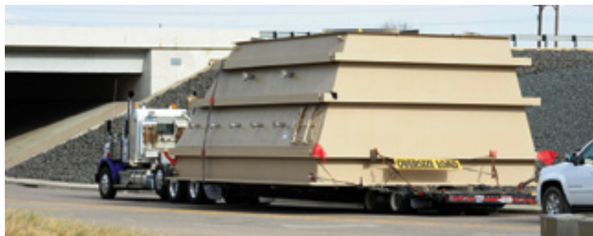
9. Very large subassemblies were prefabricated and shipped to Pueblo
