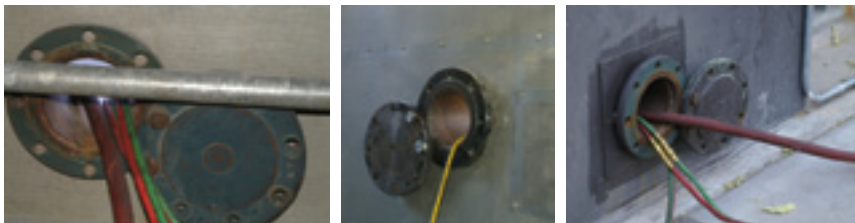
6-8. Penetrations on enclosures eliminate the need to run lines, cords, and leads through doorways
