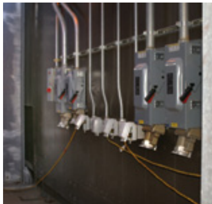
9. Plug-ins eliminate need for portable power stations
