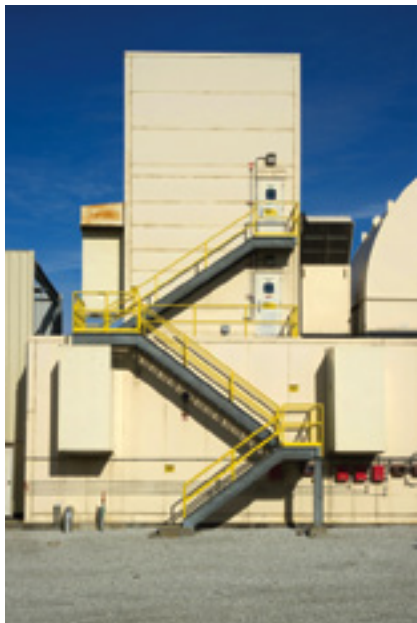
13. Steps and landings are much easier to navigate than ladders to access combustor
