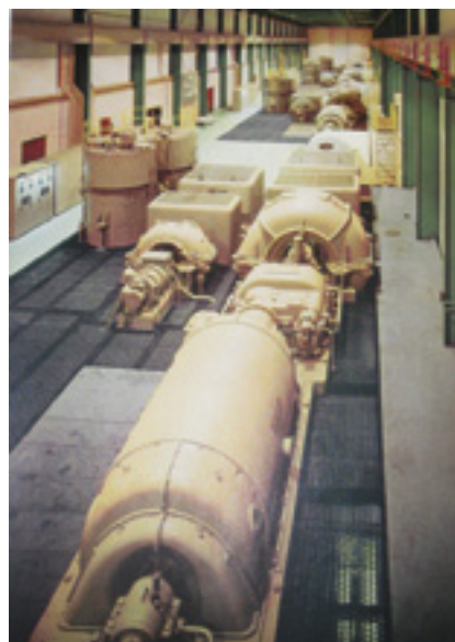
1, 2. Port Mann gas turbines had an intercooler between the LP and HP shafts to reduce the temperature of air leaving the LP compressor before it entered the HP combustor. Each shaft had a starting motor that disengaged after startup. Note that the combustion chambers are located along the left-hand wall in the photo
