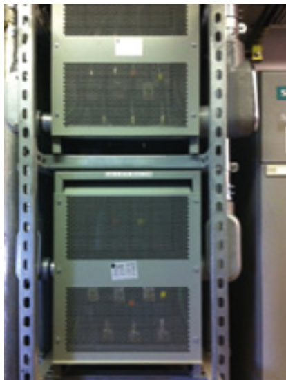
19. Load-side line reactors for each drive were installed in NEMA 1 enclosures
