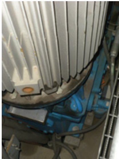
6, 7. Drip pans catch any leaking oil
