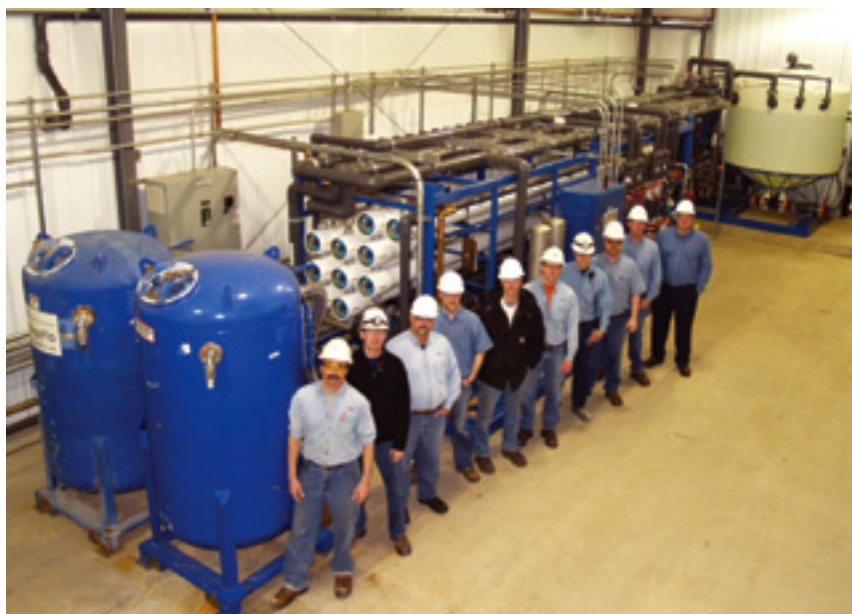
2. An ultrafiltration/RO system provides makeup both for the cooling tower and mixed-bed demineralizers
