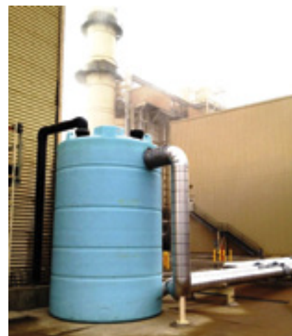
2. Residual chlorine and pH are monitored at the discharge of the 5500-gal retention tank to adjust treatment of water entering the tank
