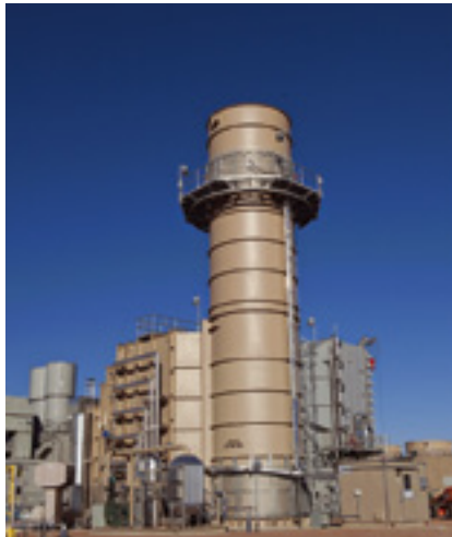
5, 6. Exhaust section for Pueblo LMS100 features redundant equipment (PLC connections to the plant DCS, tempering-air fans, ammonia vaporizers) to maintain NO x and CO emissions within permit limits
