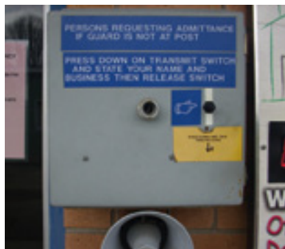
5, 6. Plant employees can allow visitors to enter the plant using their radios. A radio with tone receiver module in the gate control panel activates a relay to open the gate
