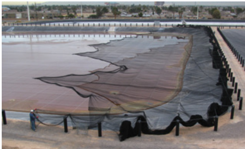
5. Netting is installed over evap ponds at NV Energy's Clark Station to protect migrating birds
