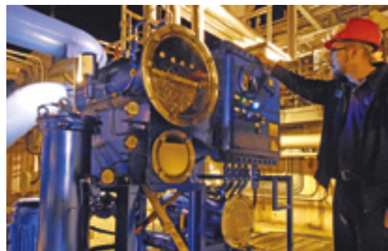
2. Vacuum dehydrator oil purification system extracts water and particulates from contaminated turbine oil
