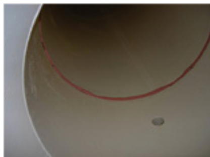
6. Chemical decontamination of the riser in Fig 4 with a low-pressure water wash prepared it for re-coating. After three years in service, the coating still was pristine. Decontamination before coating was the key
