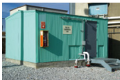
8. Fuel forwarding skid is protected from the elements
