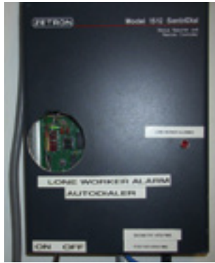
2, 3. "Lone worker" alarm is activated by an employee when working alone (above). If the alarm is not reset an automatic call for assistance is made (right)
