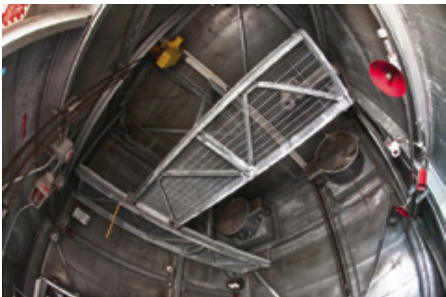
14, 15. Maintenance platform with movable sections facilitate maintenance
