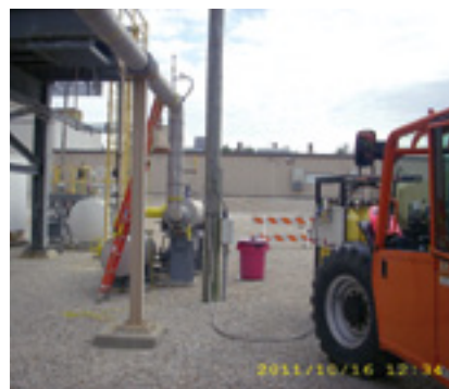
12. Key components in the Fig 9 system are the high-flow dome-type regulator and 0.75-in.-diam, high-pressure, stainless steel piping and hose. Piping is Schedule 80 (left)
