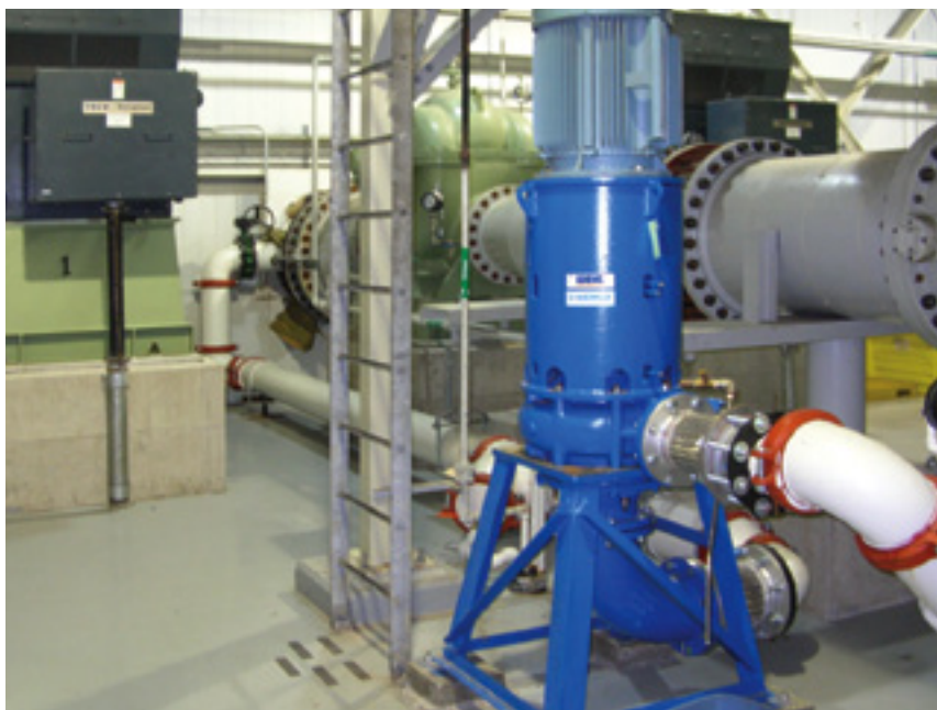
17. VFD-equipped bypass pump maintains water chemistry and system condition at much less cost than the main circ-water pump when plant is on standby
