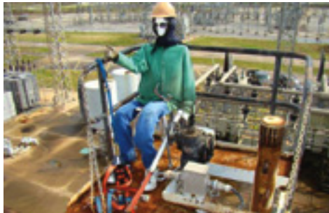
Meet Hogan! Lanyard tied off to handrail, not wearing fall protection, using a cheater bar, no safety toe shoes, pipe wrench handle bent
