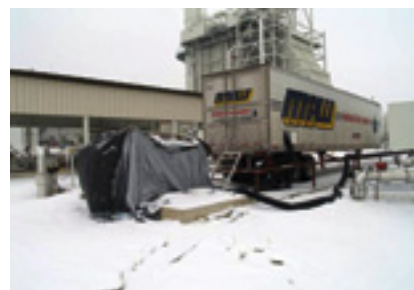
1. Cold weather adversely impacted the operation of trailer-mounted mixed-bed demineralizers and created safety issues
