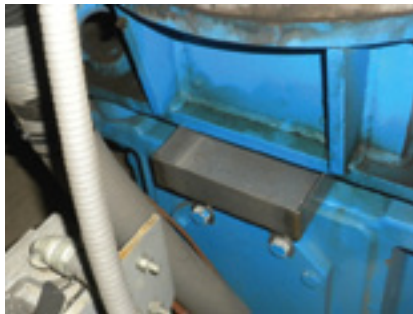
6, 7. Drip pans catch any leaking oil
