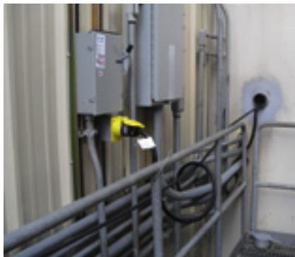
27. 480/240-V transformers were installed in each turbine's electrical control building
