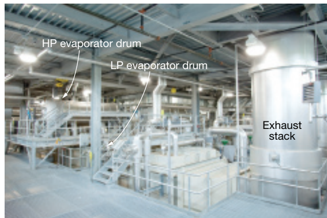
9. Balcony facilitates access to steam drums and their appurtenances
