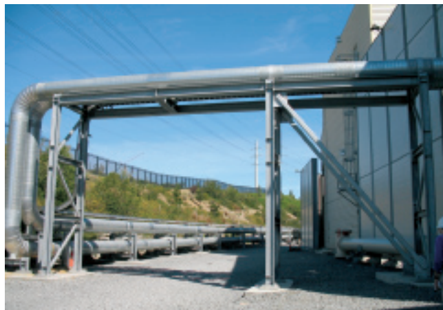
38. Chilled-water sendout/return pipes exit/enter the chiller house. Pipe returning water from the chiller coils in the air inlet house is closest to the reader
