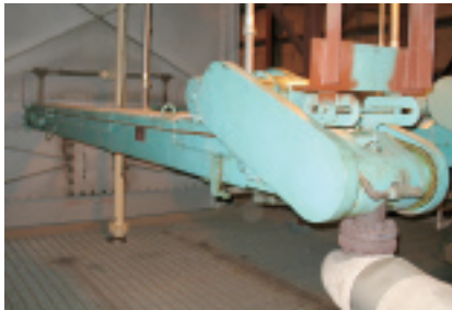
7. Sootblowers were standard on GE HRSGs burning liquid fuel
