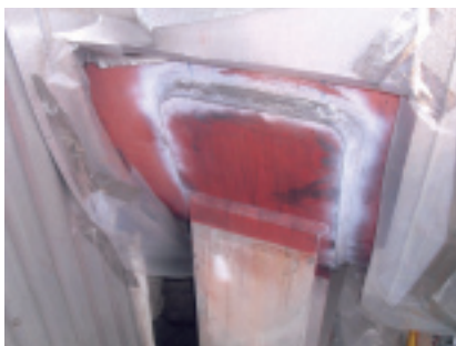
7. Crack in support saddle for HP drum was repaired during outage
