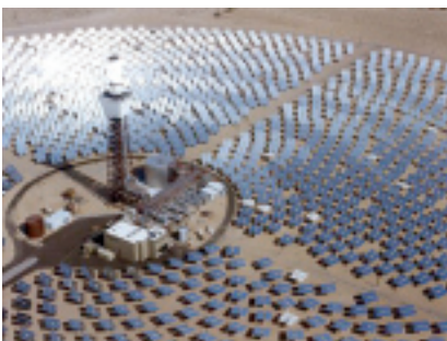
C. Solar power tower delivers steam at the highest temperature, but requires scale-up and more experience before being considered a viable candidate for integration with a combined cycle
