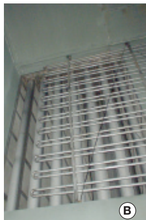
18. Heat exchanger (horizontal piping) cools compressor discharge air for pulsing service (A, B). Air leaving the coil is blended with compressor bleed air to maintain pulse air above 40F (C)
