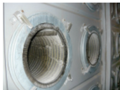
14. Pleated prefilter protects HEPA from large particles
