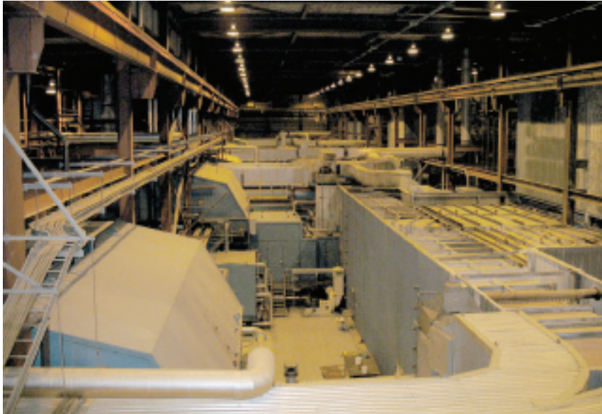
3. Gas turbines as they look leaning over the turbine-deck rail. The heat-recovery steam generator serving the first GT in the picture is to the right
