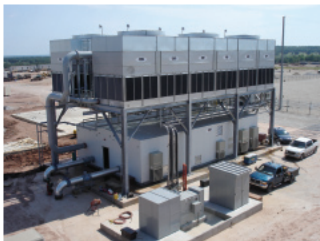
25. Chiller package located below the six-cell cooling tower came in two modules and set on a concrete pad
