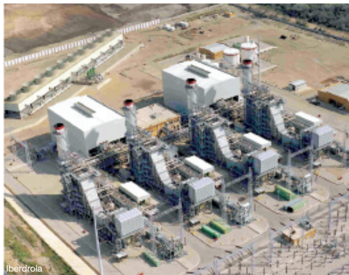
Mexico, Altamira III and IV. Each a gas-only, 518-MW, 2 × 1, GE 7FA-powered combined cycle
