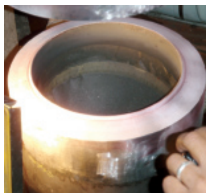
4, 5. Off-spec weld was removed with a clamshell pipe cutter (left) and the joint prepped for rewelding after verifying that no cracks were present in the material (right)
