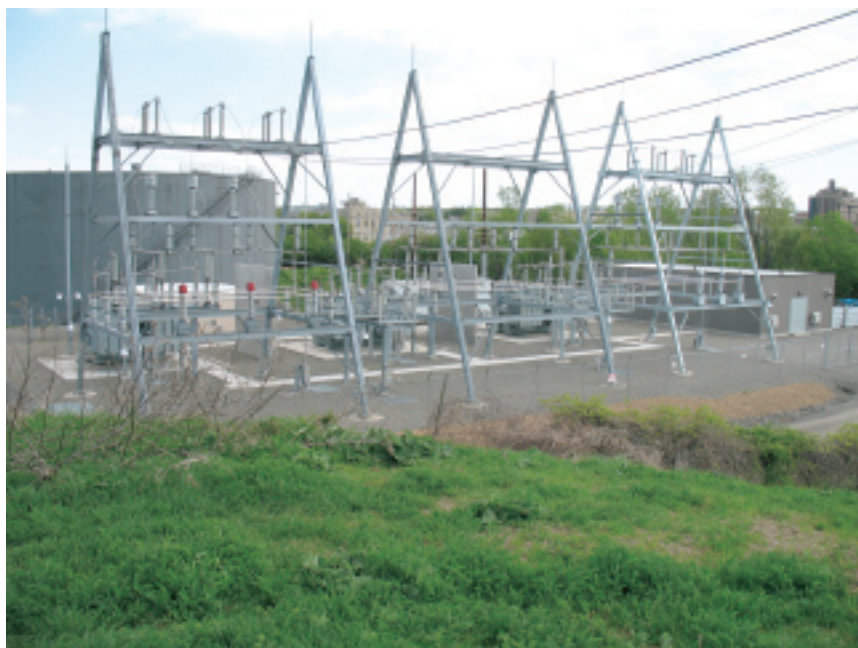
15. New substation with three 20-MVA transformers brings in 115-kV power from the utility system, provides 13.2 kV for the campus distribution system
