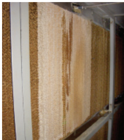
8. Microbiological fouling reduces efficiency and media life, can produce objectionable odors downstream, and can promote corrosion of framing
