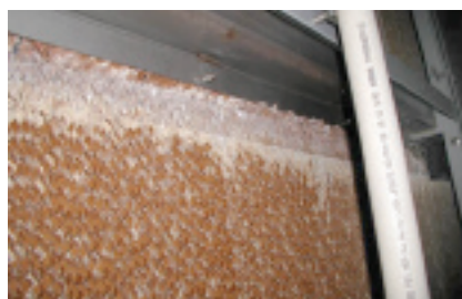
7. Scaling at the top of the media (frosty deposit) impedes proper operation of an evap cooler
