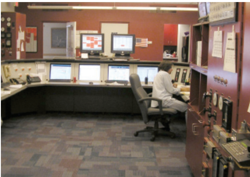
1. A well-programmed DCS can provide plant operators valuable guidance regarding corrective actions in the event of an alarm or other abnormal output from available instrumentation
