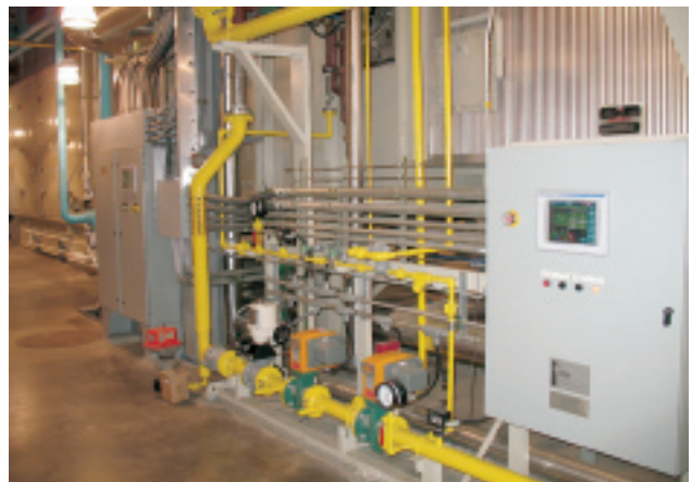
6. Duct-burner gas skid sits alongside the HRSG that it serves
