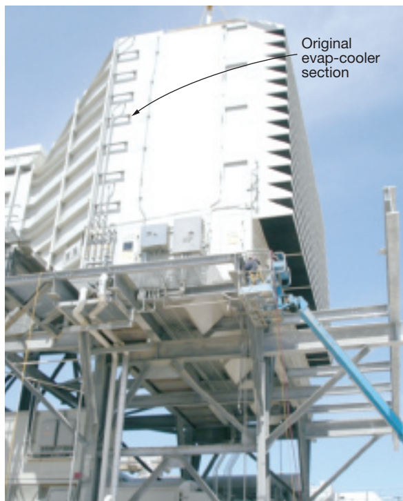
27, 28. Air inlet house as originally installed is at the left, after removal at the right
