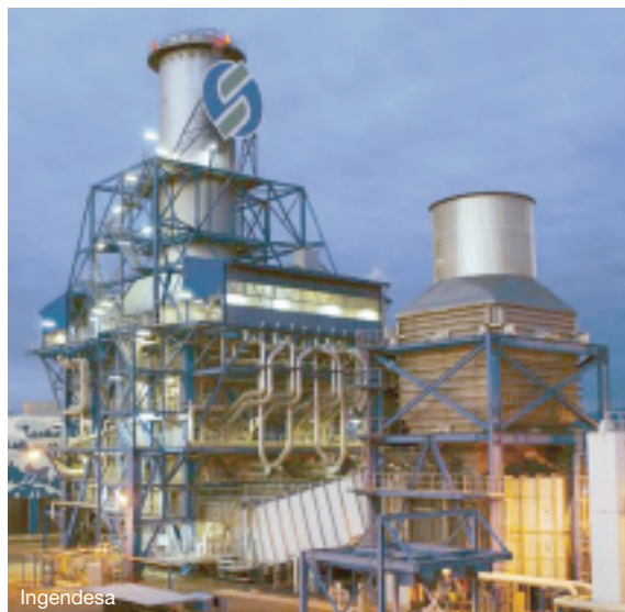
Chile, San Isidro 1. A dual-fuel, 379-MW, 1 × 1 combined cycle powered by a Mitsubishi 501F
