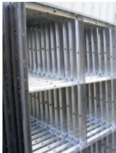
4. Framing for new static (barrier)-type filters is of stainless steel to minimize corrosion potential
