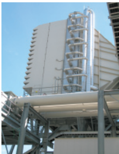
40. Vertical manifold pipe serving the six chiller coils in each air inlet house is furthest from that structure. Chilled water enters each coil at the bottom, returns out the top via the inside manifold
