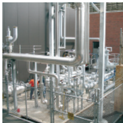
10. Permanent walkway facilitates access to GT prefilters—an important safety best practice (left)
