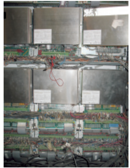
16-18. New control cabinet for peaker 2A is at left. It exactly fits in the space remaining after removal of the Mark II cabinet. Note the touch-screen operator interface. Down the aisle is the control cabinet for GT 1A with no screen. Photo in middle shows how efficient PLC-based control systems are in terms of electronic hardware and wiring. At right, the bottom of the Mark V cabinet for the DLN-1 equipped GT 1B reveals considerable clutter compared to the PLC-based control system
