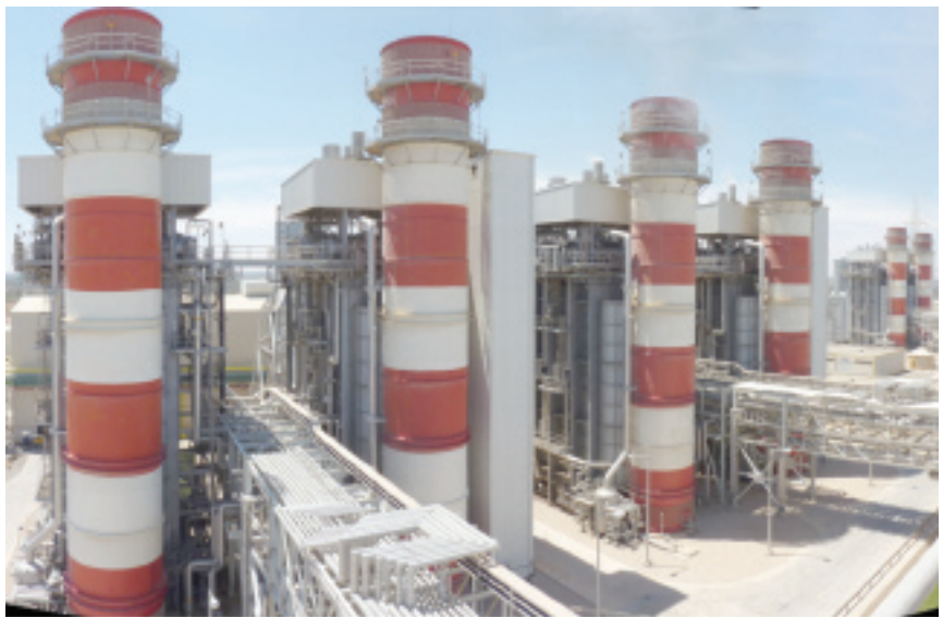
1. Libyan combined-cycle plant has three 2 \times 1 power blocks. First four Alstom 13E2 gas turbines were installed in 2001, the third block five years later
