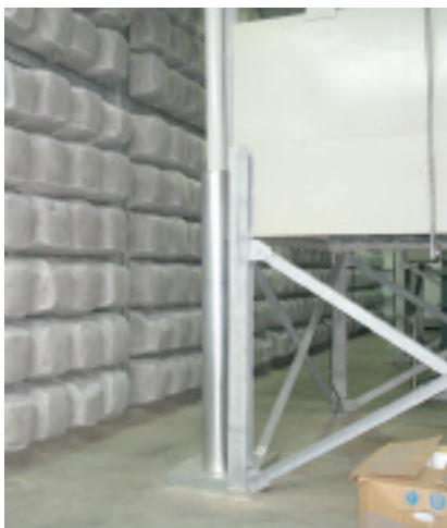
11. Gas turbine air inlet and its pulse-type inlet filters is to the right of the prefilters, shown from the back side
