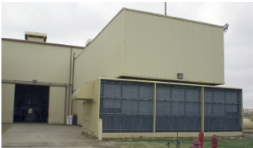
15. Ground-level air inlet supplied with Greenwood Energy Center's four 7B peakers were rudimentary by today's standards
