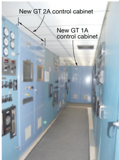
16-18. New control cabinet for peaker 2A is at left. It exactly fits in the space remaining after removal of the Mark II cabinet. Note the touch-screen operator interface. Down the aisle is the control cabinet for GT 1A with no screen. Photo in middle shows how efficient PLC-based control systems are in terms of electronic hardware and wiring. At right, the bottom of the Mark V cabinet for the DLN-1 equipped GT 1B reveals considerable clutter compared to the PLC-based control system
