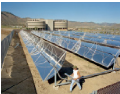
A. Parabolic trough is the most popular solar-thermal technology today and the one selected for all the ISCC plants entering service this year
