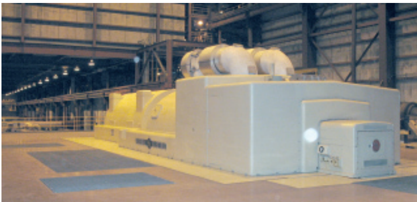
2. Nominal 100-MW steam turbine guards one end of the building and looks down on the gas-turbine "alley"
