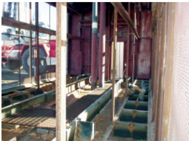
16. Evap coolers were disintegrating and demolished
