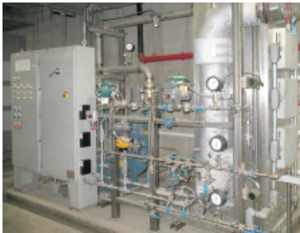
7. Ammonia skid receives reagent for the SCR from a 12,000-gal storage tank located a couple of hundred feet from the CHP building (left)
