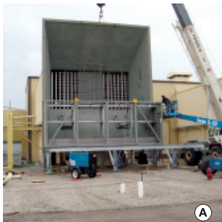
18. Heat exchanger (horizontal piping) cools compressor discharge air for pulsing service (A, B). Air leaving the coil is blended with compressor bleed air to maintain pulse air above 40F (C)
