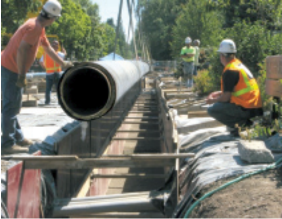
8. Preinsulated steam pipe connects the cogeneration plant to the existing steam network five blocks away
