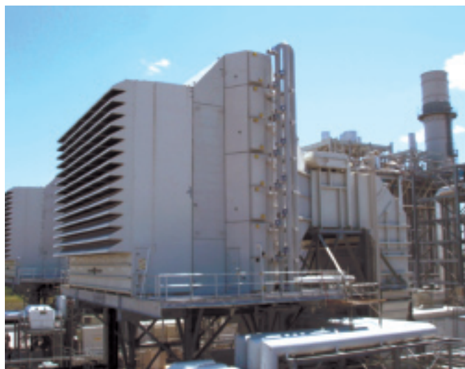
30, 31. New air inlet house, in drawing at left, photo at right, extends 17 ft beyond where the original inlet house ended
