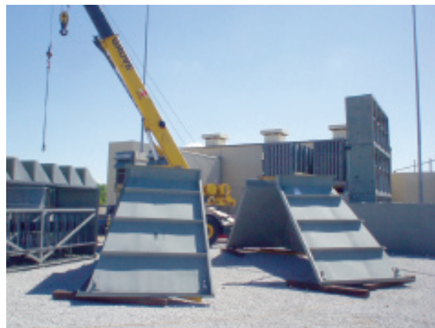
17. Transition-piece halves for the new air inlet system await installation
