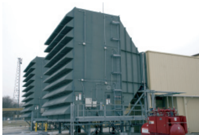
19, 20. Filter module is prepared for a pick (left), fully assembled replacement air inlet is at right
