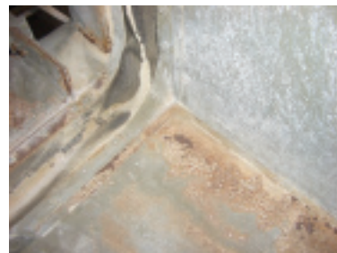
5. Corrosion of air-inlet floor must be addressed to prevent metal from flaking off and being ingested by the gas turbine
