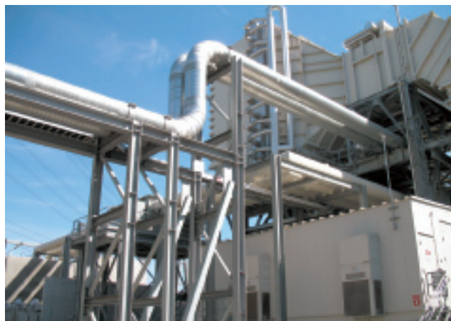
39. Chilled-water supply pipe is closest to the reader
