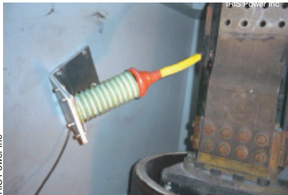
6. Partial-discharge sensor can provide considerable information on generator condition
