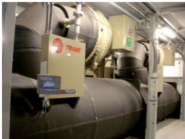
26. Chillers were installed inside the modules prior to delivery onsite
