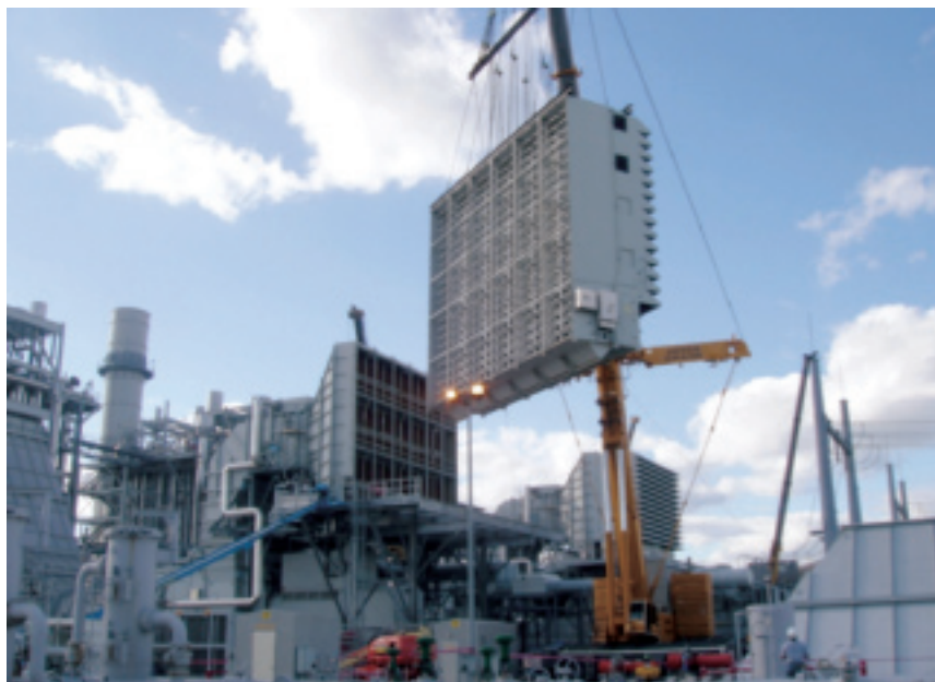
29. Original filter module is lifted into place after installation of the new chiller section and transition duct
