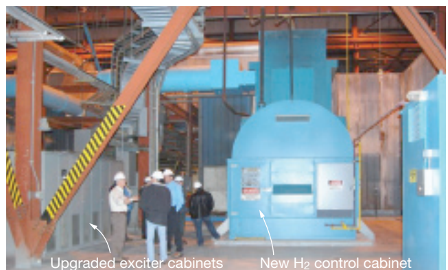
20. Exciter controls for the gas turbine generators were replaced by ICS as part of its workscope; plant staff installed new hydrogen control cabinets
