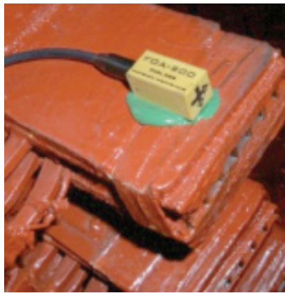
2. Stator end-winding vibration sensor pickup, relatively easy to install, helps prevent generator forced outages
