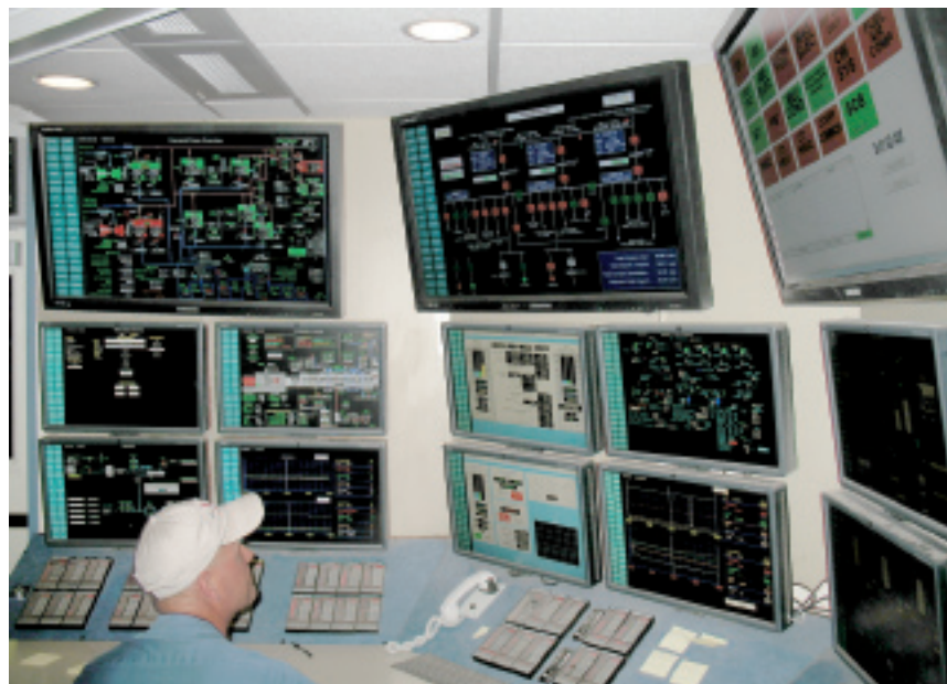
13. Operator Tom Brown is within easy reach of punch button to both stop gas flow and vent the line in an emergency. Two operators run the CHP facility and the existing infrastructure in the central steam plant. Total energy complex has a union staff of 22, including four I/C technicians (below)
