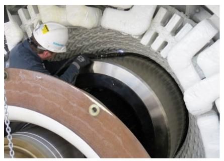
**Limited clearance** can make it challenging to get a robot into a generator. For some machines, the gap is too small for any robot to gain access
