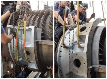
7. Rollers are bolted to the lower half of the compressor case to guide and support its removal
