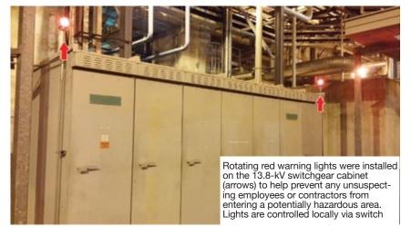
12. Rotating red lights (arrows) warn when an arc-flash hazard is present
