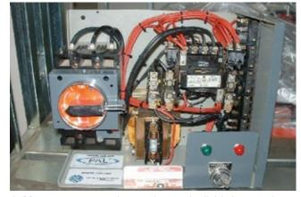
**6. Motor starters** are heavy-duty and reliable but need regular servicing. Shown here is a reconditioned starter with LED lighting and new contacts
