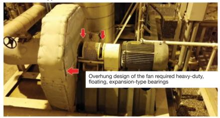
4. A tighter balancing requirement limited the radial loading on the couplingend bearing
