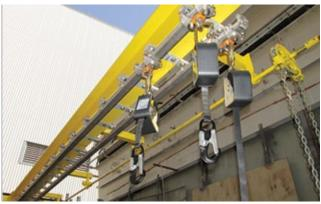
3. Alliant Energy's enclosure safety solution consists of retractable lanyards underneath an engineered rail
