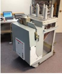
17. Remove and service the main power circuit breaker (device 52G)
