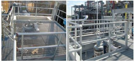
**1. Large motor-operated isolation valve** originally was installed in an obstructed location (left); corrected arrangement is at right
