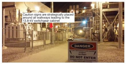
**13. Highly visible, durable signage** warns of hazardous operations. Arrow points to 13.8-kV switchgear
