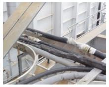
5. Leaking sample lines and heattracing failures were relatively common
