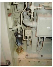
**15. Test solenoid valve** (black) to verify the stop/ratio valve will close on loss of trip-oil pressure
