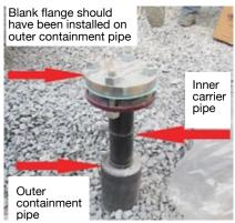
2. Aqueous ammonia piping with improperly installed flange could have led to a serious safety and environmental event
