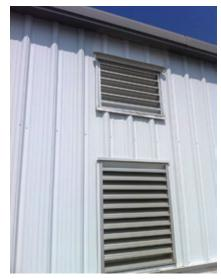
**11. Inlet and outlet air ducts** are separated by only 2 ft and the louvers serving the upper hot-air ducts were angled downward, allowing recirculation of hot air to the inlet
