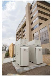
**1. Micro-turbine/generators,** gasfired, have recuperators to capture exhaust heat for improving engine efficiency and heating water
