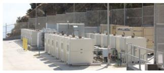
**2. Microturbines** supplied by Capstone Turbine Corp provide the flexible generating capability required on Catalina Island
