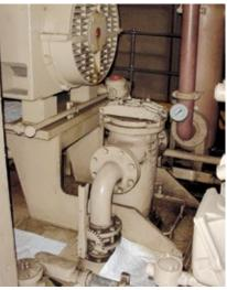
**16. Actuate the liquid-fuel stop valve** (center) with trip oil after verifying that the spring is in good condition
