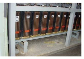
7. Individual battery cells comprising a 125-V DC system are numbered
