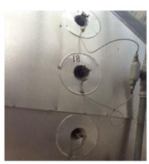
**10. New flashing design** protects T/ Cs and cable against excessive temperatures
