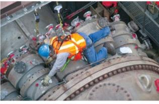
2. Tethered technician works atop the gas turbine with freedom of movement
