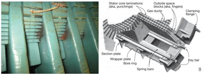
5. In high-speed generators with indirect-cooled stators, the large set-back and step-back of core iron at the ends of 6. The magnetic core, and frame, are a complex structhe core protects against the condition shown in Fig 4
