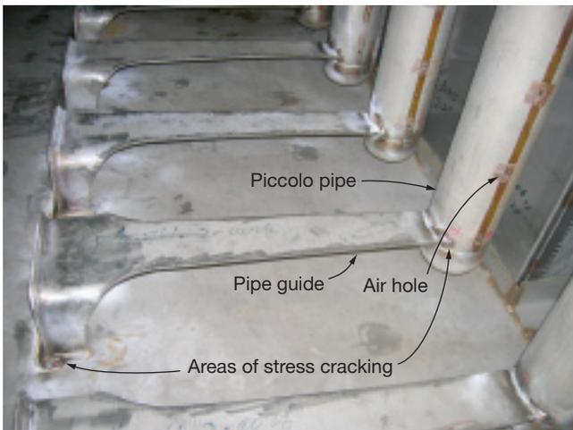
**9. Stress cracking** is relatively common on piccolo pipes where they attach to their respective pipe guides and in the areas where pipe guides attach to the floor. Stress cracks also may be found in the duct floor and in the pipe guides themselves
