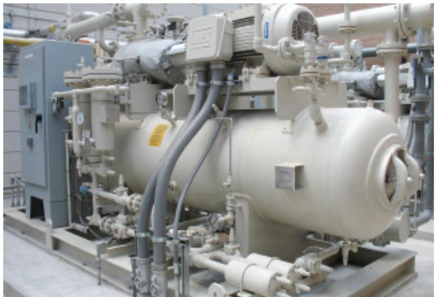
**3. Compression skid** boosts gas pressure from 40 psig as received to the 265 psig required by the Taurus™ 60's combustion system. Three skids are installed (one a spare) to remove liquids, particulate
