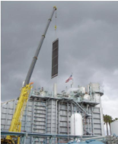
**5. New HP evaporator module,** located immediately downstream of the ammonia injection grid (refer to Fig 4), is lowered into place. The single HP superheater module also was replaced (left)
