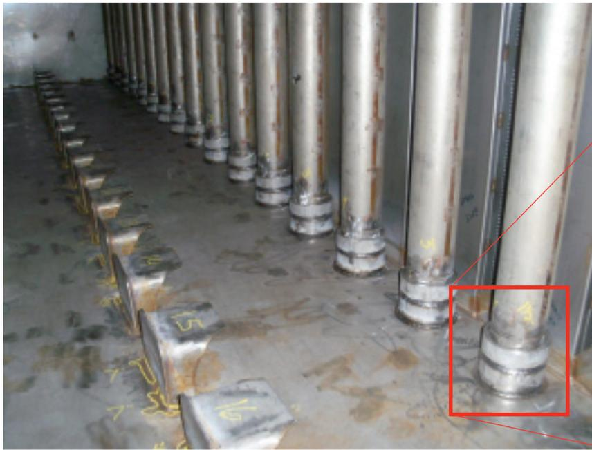
**11. Installation of the new guide sleeves went according to plan and has eliminated the need for annual crack repair**
