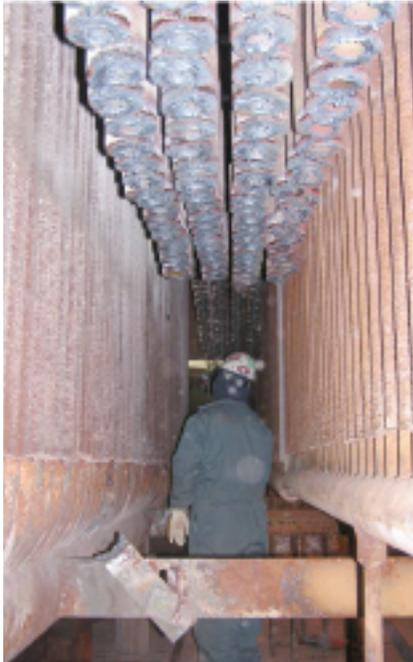
**8. Tube rows were removed (left) by cutting tubes in nominal 10-ft segments and lowering them one by one to the floor. Each segment weighed just under 100 lb (with foulant)**
