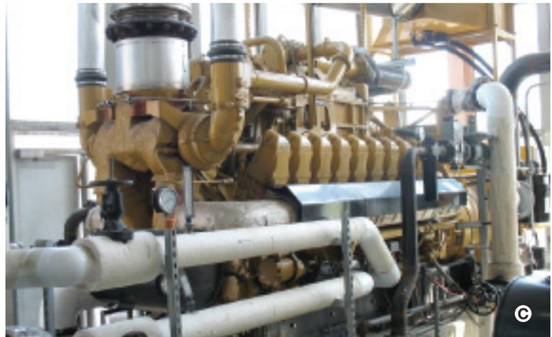
**2. The new cogen plant** is integrated into an especially flexible and reliable electrical supply system that includes a 69-kV line from Toledo Edison Co and seven engine generators with multiple fuels capabilities (A). Three aeration blowers (B) for wastewater treatment share building numbered 17 on site layout with the engine generators (C)
