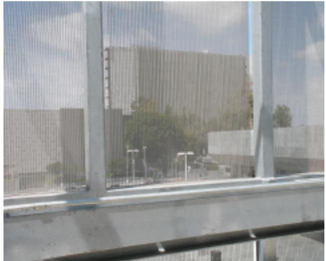
**8.** Architectural curtains obscure from view all rooftop equipment—including gas-turbine air inlets and dump condensers
