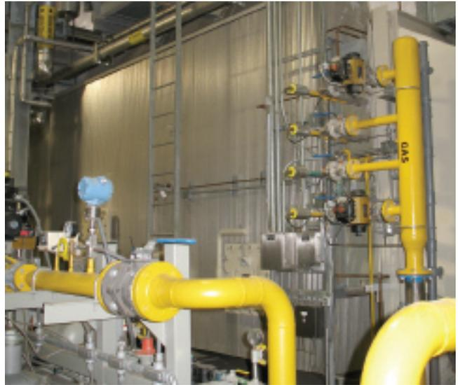
**5, 6.** Waterwall surface for HRSG is in the foreground of photo at left looking down at the Taurus 60 package. At right, duct burner and fuel skid are visible looking toward the rear of the waterwall section. Such tight spacing required locating catalyst beds and economizer in the vertical section shown clearly in Fig 4 but not here
