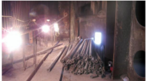
**9. Tube segments await removal through stack door (right)**
