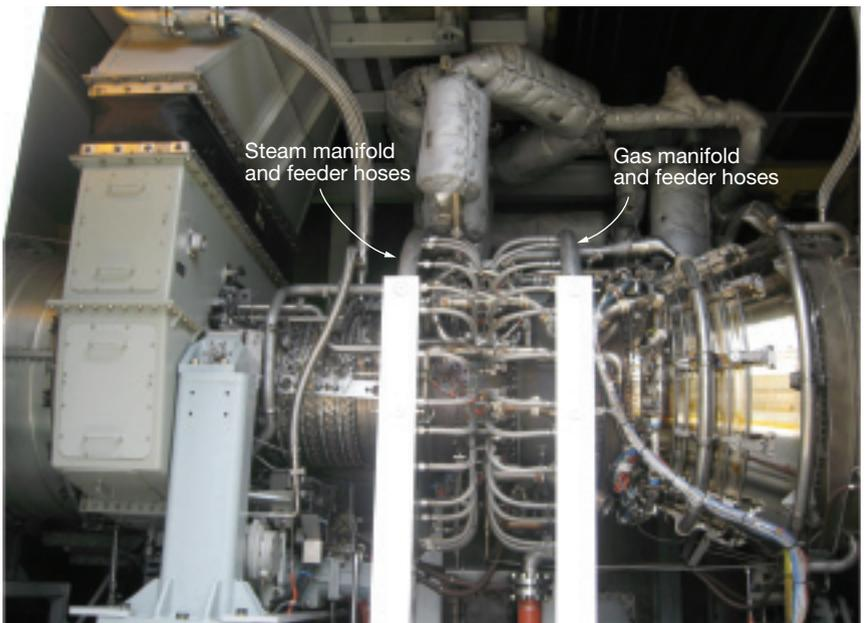
**2. Combustor arrangement** reveals one steam and one gas manifold. Steam here is for NO<sub>x</sub> control
