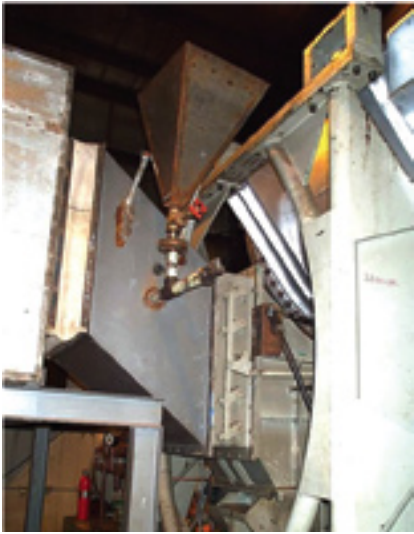
3. Hopper feeds solid cleaning agents (rice hulls, walnut shells) into compressor. Emergency stop lever closes the inlet damper valve to starve the GT of air flow
