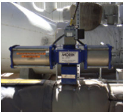
5. Plant valve mods eliminated shaft/bushing binding and resultant automatic unloads
