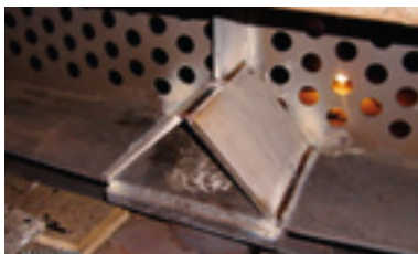
2. Reinforcement plates were installed on the inside face of the perf plate
