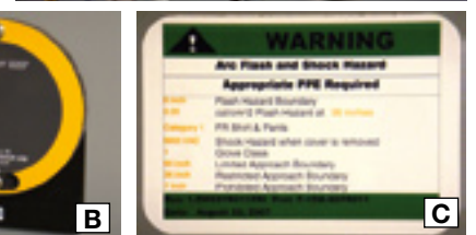
7. Arc-flash safety practices for medium-voltage switchgear (A) include use of infrared windows for thermography surveys (B) and clear instructions to protect personnel (C)
