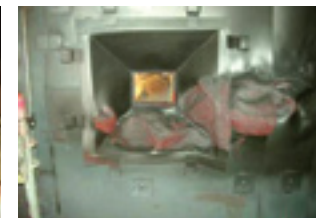
8. Wall around view window was damaged by heat from the duct burner
