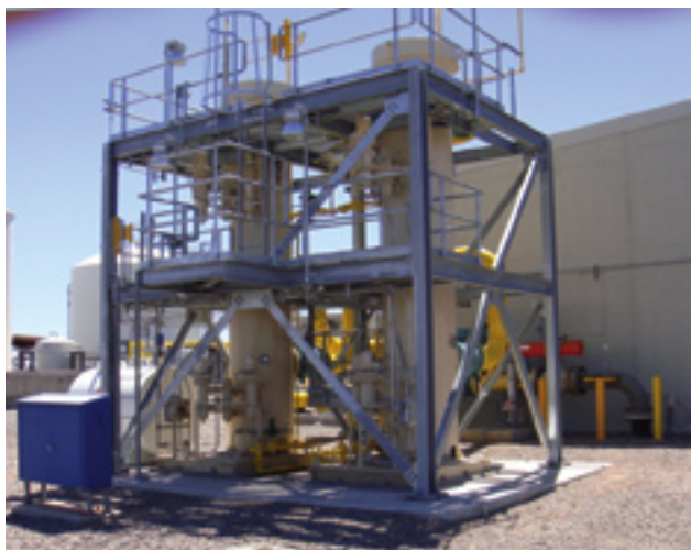
1. Coalescing filters protect against gas liquids (left)
