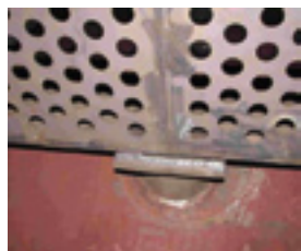
1. Perf plate is welded to the HRSG only at the bottom center position
