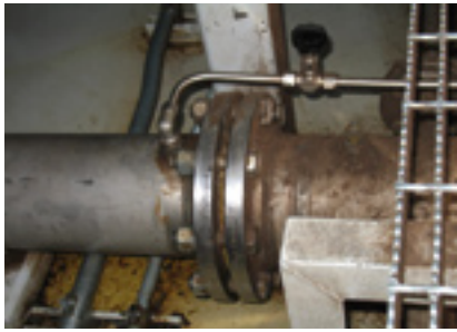
19. Oil is supplied to the LO pump thrust bearing via a connection on the discharge piping (above)
