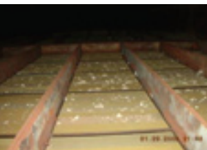
7. Catalyst face is fouled with insulation
