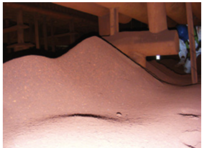
9. Foreign material removed from finned tubes must be collected and sent to a landfill
