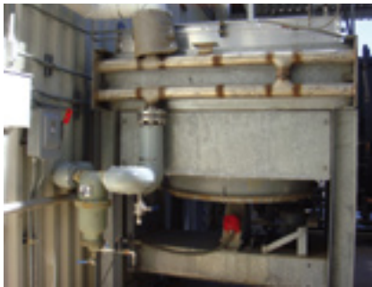
4. Fin-fan cooler allows use of GT compressor air for plant use
