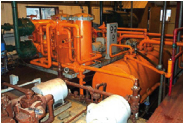
4. Lube oil system takes up some serious floor space
