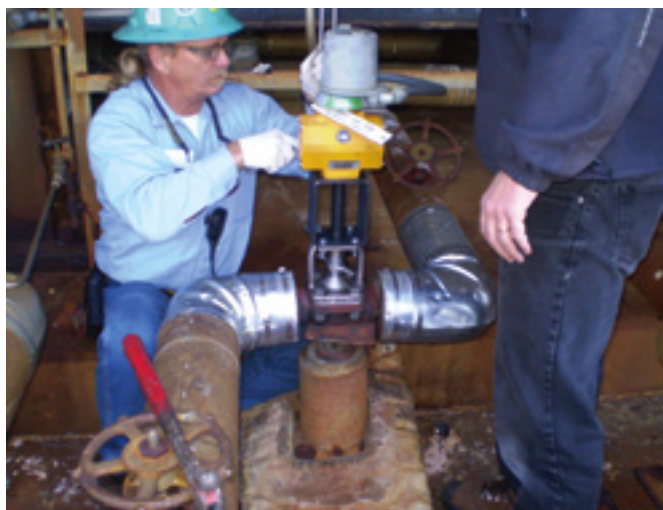
3. Ball valve, 1 in. and pneumatically operated, is installed in drain line to handle 2300 psig/950F steam conditions
