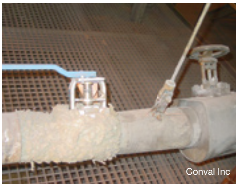
4. Ball valve for main-steam drain isolation service replaced an ineffective gate. Body is of F91 material
