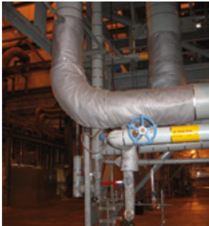
3. Removable insulation facilitates P91 hardness surveys
