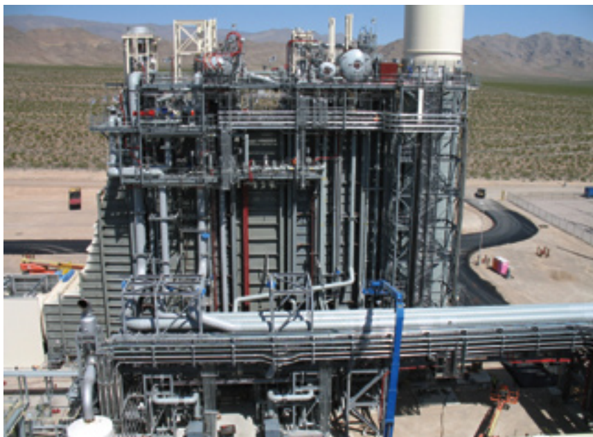
3. Heat-recovery steam generator is a triple-pressure natural-circulation unit equipped with gas-only supplementary firing to support summer peak demand
