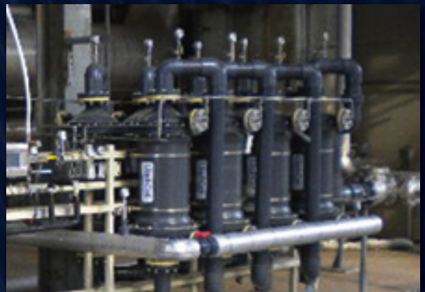
14-inch Degassing System Installed to prevent additional boiler corrosion
