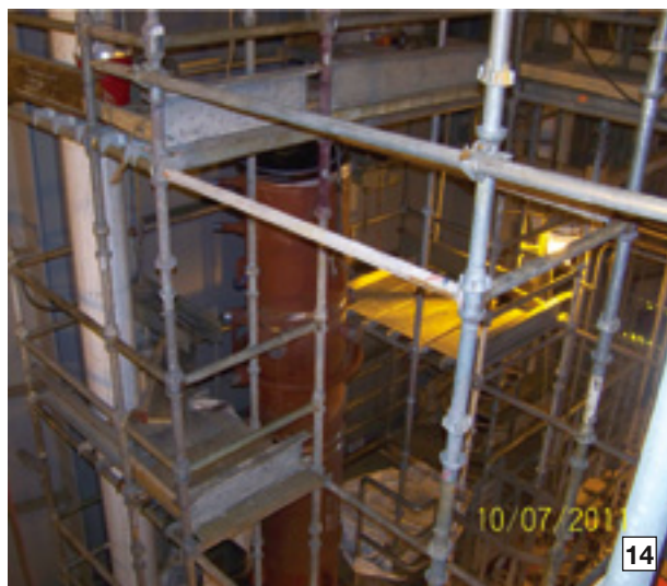
13-17. Top vertical section of new interstage piping, incorporating the attemperator, is hoisted into place in Figs 13-15. Lower section remains suspended over the elbow in Fig 16; welder joins two segments in Fig 17
