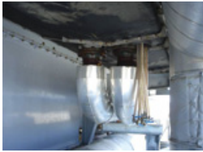
7. Chiller-coils are easy to drain before ambient temperature plummet using flexible hoses
