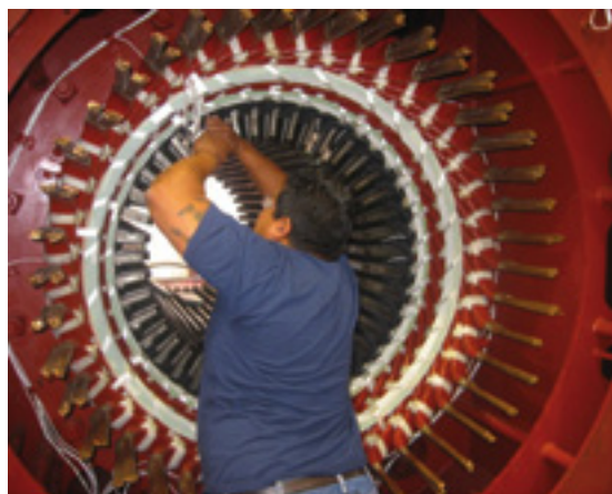
3. Generator stator rewind “zero hours” a major component of the classic Frame 5 generator. With the proper winding redesign, output can be increased
