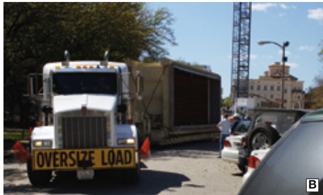
8A-G. Unloading of HRSG modules and duct sections and their placement in the building required several separate handling steps and close coordination among all parties involved
