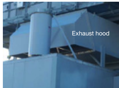
8. Exhaust hood prevents cold air from blowing directly into the generator compartment
