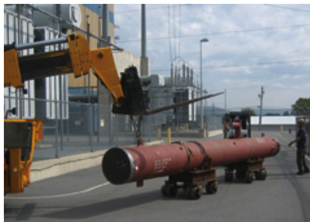
9-10. New section of pipe is wheeled into the plant (left) and prepped for welding (right)
