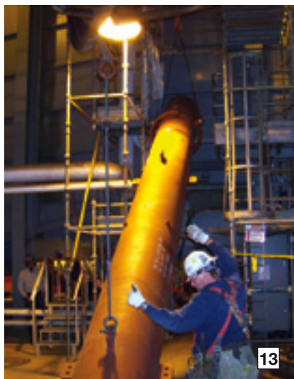
13-17. Top vertical section of new interstage piping, incorporating the attemperator, is hoisted into place in Figs 13-15. Lower section remains suspended over the elbow in Fig 16; welder joins two segments in Fig 17
