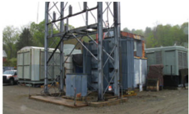
6. Fifty years later, the back side of the Ascutey enclosure (left) shows stack, and roof and side of the engine compartment, have been removed to access the rotor for a shop visit. Cables from the unit transformer to the grid were disconnected to allow safe crane access (right)
