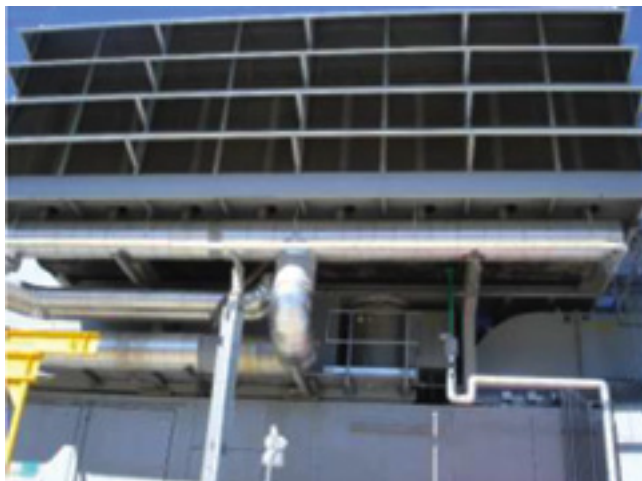
1, 2. Platforms were installed to facilitate safe access to chiller-coil drains (left) and air inlet house (right)
