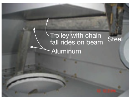
4. Generator-fan lifting device eliminates unsafe working environment
