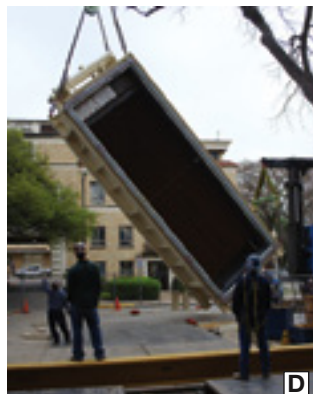
8A-G. Unloading of HRSG modules and duct sections and their placement in the building required several separate handling steps and close coordination among all parties involved
