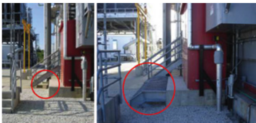
3. A trip/fall hazard (left) was avoided by modifying ground-level access (right) to a critical cabinet
