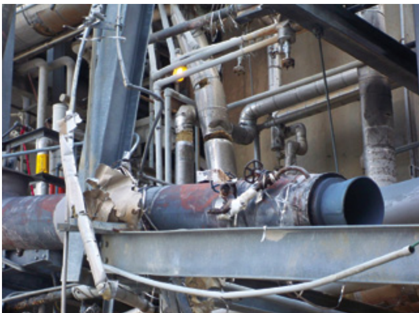
15. Catastrophic failure of a shop weld on a 16-in. flow element in a nominal 1500-psig/900F main steam line miraculously injured no one
