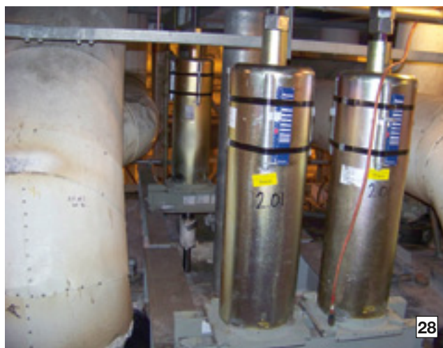
25-28. Replacing fixed supports on the upper headers for Reheater 1 with spring cans is expected to reduce significantly the number of tube failures in the years ahead. Lugs supports are added in Fig 25, spring cans and associated hardware are shown in Figs 26 and 27; the installed cans are in Fig 28
