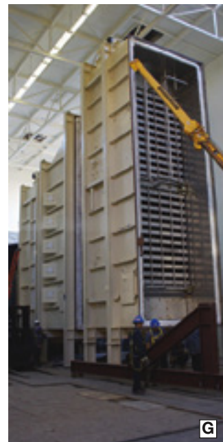
8A-G. Unloading of HRSG modules and duct sections and their placement in the building required several separate handling steps and close coordination among all parties involved
