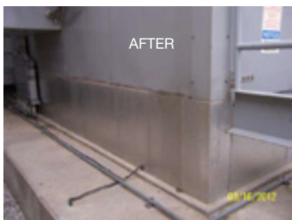
11. Insulating package base structural members minimizes heat loss and reduces the potential for freeze-up issues
