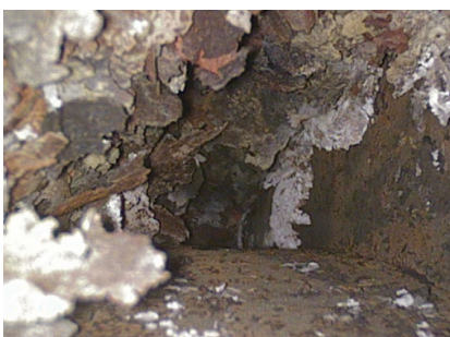
21. Condition of the quaternary annulus before cleaning
