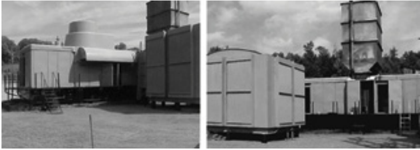
5. Ascutney gas turbine shortly after installation in 1961. Control cab is at the far left in the left-hand photo and adjacent to the auxiliaries compartment; the air inlet house is at the right and perpendicular to the enclosure. The engine compartment is visible on the other side of the air inlet; the generator and exciter are to the right of the stack
