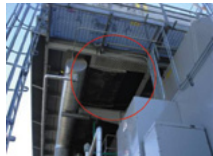
10. Bird screens prevent roosting pigeons from clogging condensate drains
