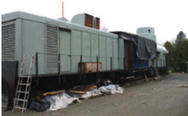
6. Fifty years later, the back side of the Ascutey enclosure (left) shows stack, and roof and side of the engine compartment, have been removed to access the rotor for a shop visit. Cables from the unit transformer to the grid were disconnected to allow safe crane access (right)
