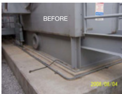
11. Insulating package base structural members minimizes heat loss and reduces the potential for freeze-up issues
