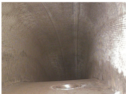
22. Quaternary annulus after cleaning with ATS' dry in-situ procedure
