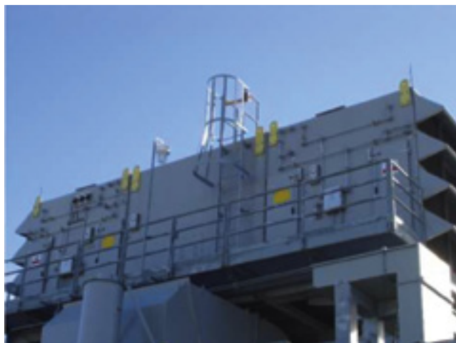
1, 2. Platforms were installed to facilitate safe access to chiller-coil drains (left) and air inlet house (right)
