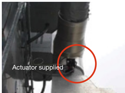
9. Damper actuator (left) was replaced by manual operator (right) to improve cold-weather reliability
