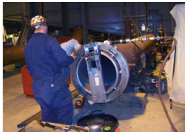
9-10. New section of pipe is wheeled into the plant (left) and prepped for welding (right)
