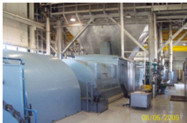
4. First Frame 5 used in a combined cycle is still operating at Wolverine Power Supply Cooperative Inc, Cadillac, Mich. The product name for the 1 x 1 single-shaft configuration is STAG 105
