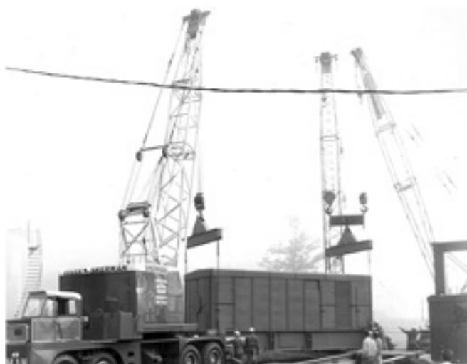
1. Generator section is lowered into position at Central Vermont Public Service Corp's greenfield Ascutney plant in 1961. It is believed to be one of only four MS5001D generating sets still in service. CVPS owns two of the four
