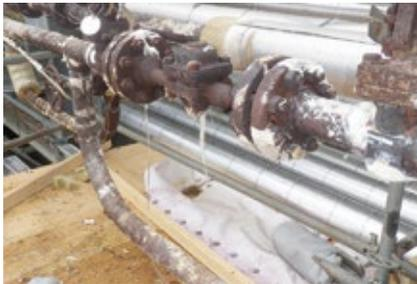
**3. Steam trap** arrangement used in Newington's cold-reheat piping
