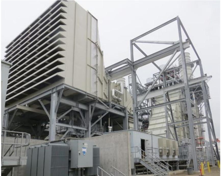
1, 2. First 7FA.05 in foreground above exhausts through a heat-recovery steam generator which supplies the grey market D11 steamer below
