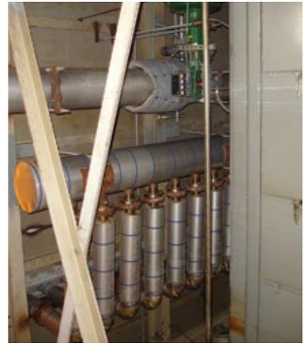
25. Reverse-acting valve allows injection of steam via inlet bleed heat system to boost output
