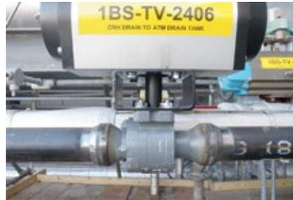
**5. Smart drain valves** replaced steam traps in the cold-reheat system
