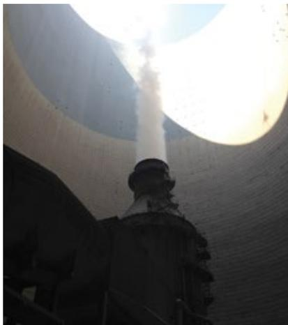
5. Hot flue gas promotes air flow through Qinling's cooling tower
