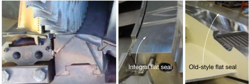
**4. New integral seal** is much more difficult to repair correctly, even for normal wear, than the old style replaceable seal
