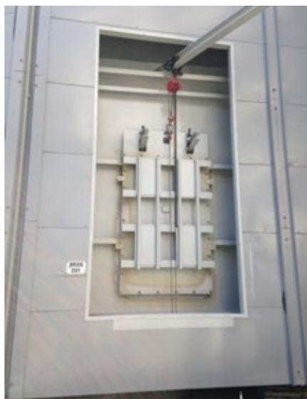
**2. The new door** required a trolley system for removal/replacement (left); door interior is at the right
