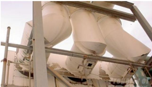
**C. Peeling or discolored paint** typically warns of excessive heating (above)
