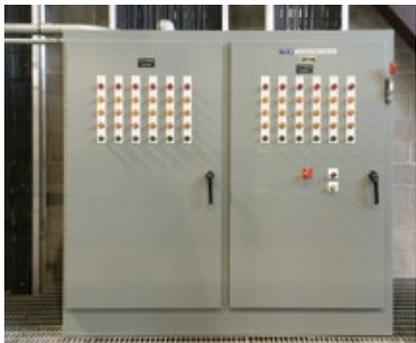
control cabinet serves each turbine (Fig 3). The cabinets are equipped with an integrated monitoring system consisting of current sensors, ground-fault indicators, etc; also, local remote switches, auto switches, on/off lamps, and alarm indicating lamps.
