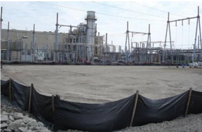
22. Existing steam turbine will be complemented by a new 27-MW steam turbine/generator destined for the prepared site behind the HRSGs
