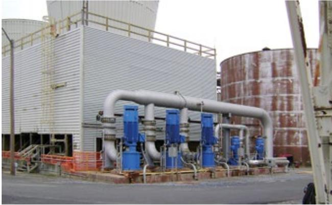
17. Main and auxiliary circ-water pumps overhauled
