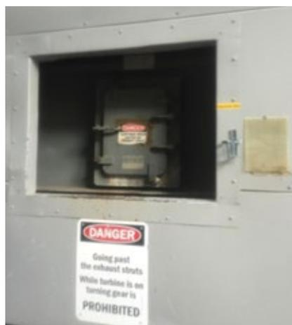
**1. The original HRSG access door** was not conducive to quick entry/exit
