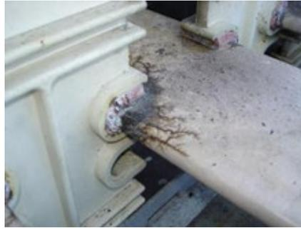
**6. Blown non-seg bus** at right is rare, but it happens; at left, damage caused by insulation break-down
