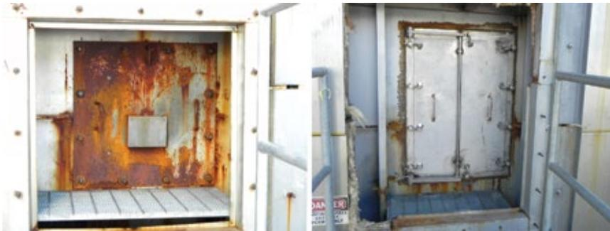
**2. Replacing bolt-on access hatch** (left) with pivoting door at right dramatically reduced the risk of injury to maintenance personnel
