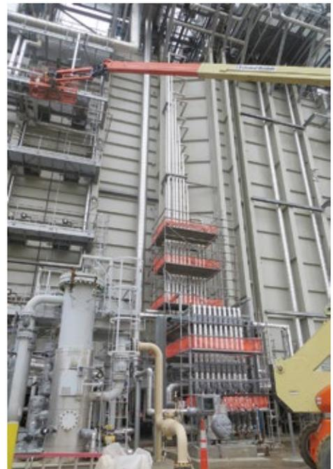
**5, 6. SCR ammonia system** reflects latest design. Blowers at left direct air to the heaters used to vaporize aqueous NH<sub>3</sub> (left). Delivery system assures proper distribution of reagent to the catalyst bed (right)
