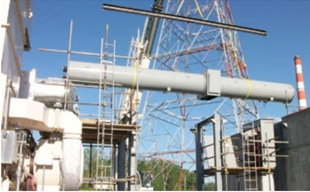
**8. Circular non-seg bus** has rigidity to facilitate transport and crane lifts
