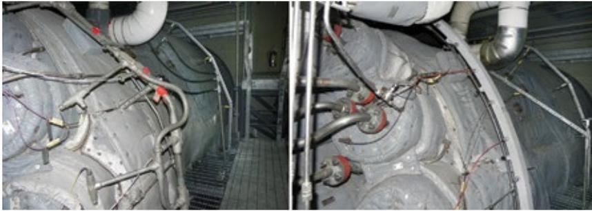
**1. Plant personnel** redesigned and replaced the original instrument wiring system (left) with one that provides more robust support and protection (right)
