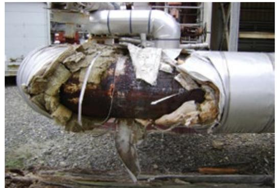
4. Corroded and misaligned steam pipe
