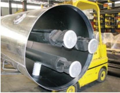
**5. Circular non-segregated phase bus** is an alternative to the rectangular design shown in Fig 4 and offers many advantages of isophase bus
