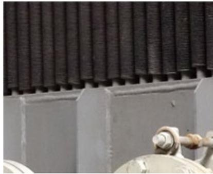
4. Qinling's indirect-cooled ACC features nominal 50-ft-long finned tubes at the base of the natural-draft tower. High-purity water circulates through the closed-loop cooling system
