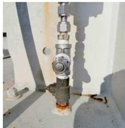
**Addition of a valve and test port** facilitates hook-up of test instruments to verify proper operation of equipment
