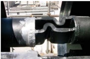
**9. Inherent rigidity** of circular non-seg bus minimizes structural support requirements (above)
