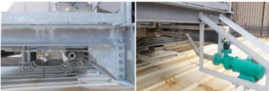
1. Original location of evap-cooler pumps is shown at left, new location at right
