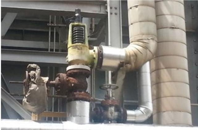
**11. Locking device** to prevent closure of block valve when steam system is in operation appears to be missing. A proper drain line at a low point in the steam vent system also seems to be missing (left)
