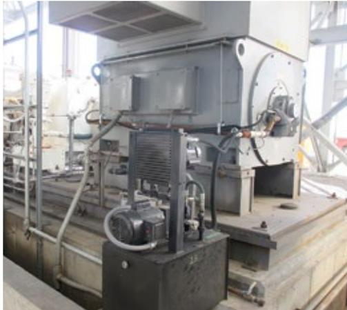
**Self-contained oil reservoir/cooler/pump skid** reduced wear and tear on motor bearings
