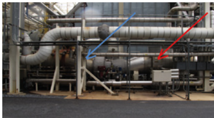
A. Rotor air cooler, or kettle boiler, is found in the majority of plants powered by 501F and 501G gas turbines (left)
