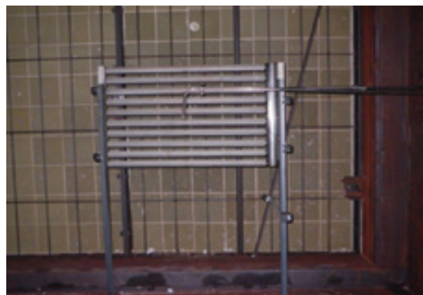
4. Supplemental AIG assembly installed at Clearwater Cogen
