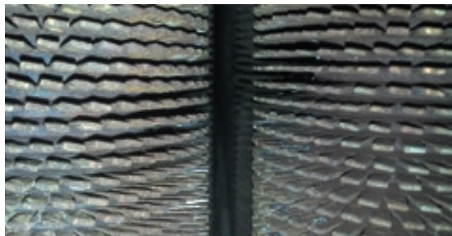
4, 5. Typical fouling and bridging of tubes before cleaning is shown at left. At right, the same tubes have been restored to “new and clean” condition by blasting with CO 2 pellets
