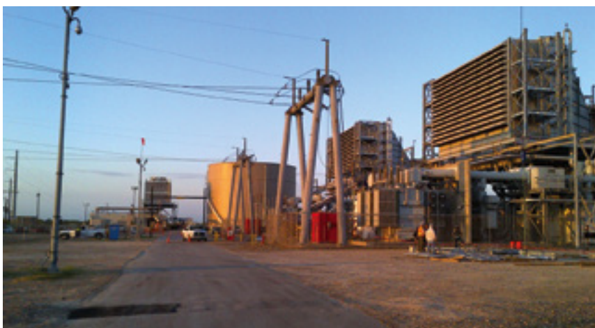
1. Frontera Energy Center's new inlet-air houses feature outside egress on both sides (foreground). Chiller is to the left of the thermal energy storage tank
