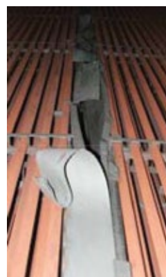
12. Failed baffle was designed to prevent turbine exhaust gas from bypassing heat-transfer surface by flowing between adjacent panels
