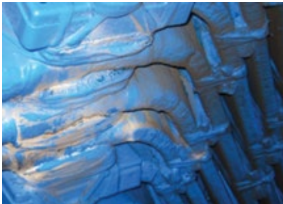
1, 2, 3. Dusting is indicative of early-stage vibration in endwinding
