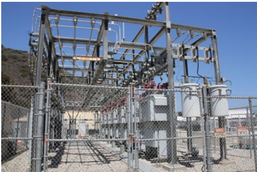
5. Substation delivers power to the island through three 12-kV circuits
