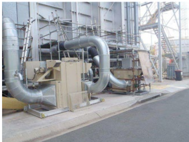
3. Long-term layout of Swanbank's HRSGs relies on dehumidifiers for the water/steam circuit and gas path
