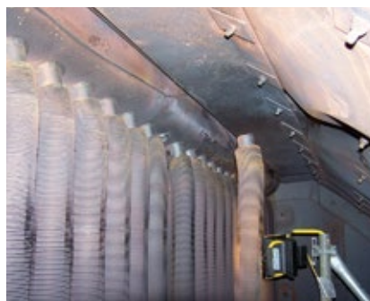
2. Tube-to-header joint failures in the HP/HT superheater were caused by desuperheater overspray
