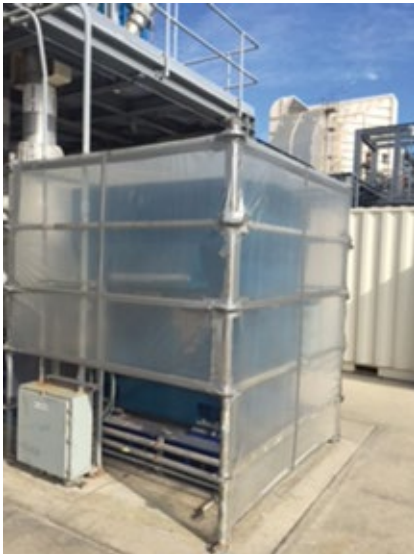
5. Plastic hood covers the boiler-feed-pump motor to protect against ingress of moisture and sea salt
