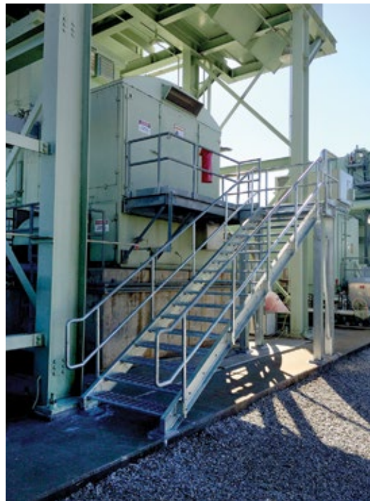
1. Making the workplace safer by facilitating access to equipment. Generator terminal enclosure before stairs were added is above; after, right
