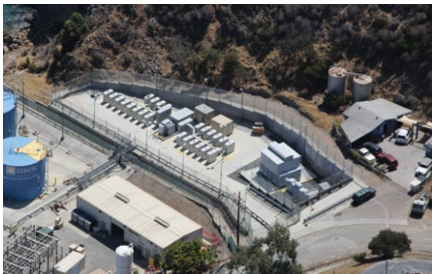
2, 3. Twenty-three 65-kW micro-turbine/generators (at left in enclosed area at center of photo) are located adjacent to the 1-MW NaS battery and power conditioning system (right). Close-up of battery and PCS is below. They allow SCE to optimize diesel operation to minimize emissions and more precisely respond to wide fluctuations in demand
