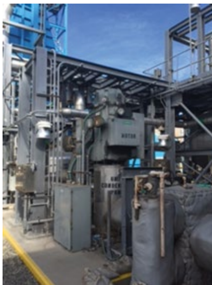
6. Several platforms and access doors were added to facilitate inspection and maintenance of the GT exhaust duct
