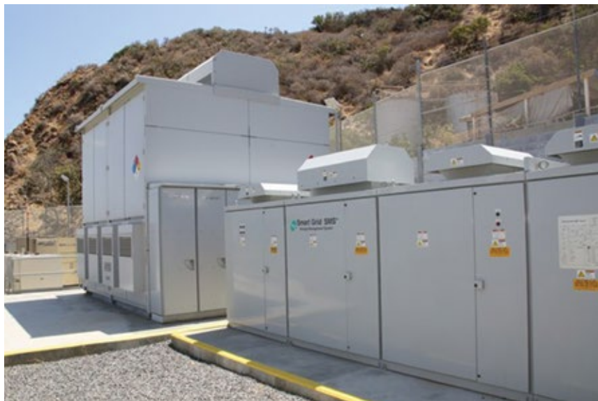
2, 3. Twenty-three 65-kW micro-turbine/generators (at left in enclosed area at center of photo) are located adjacent to the 1-MW NaS battery and power conditioning system (right). Close-up of battery and PCS is below. They allow SCE to optimize diesel operation to minimize emissions and more precisely respond to wide fluctuations in demand
