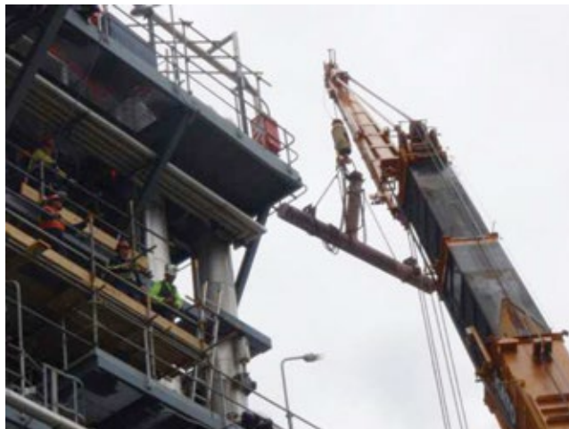
4. Otahuhu's at-risk P22 headers were replaced with ones made of P91
