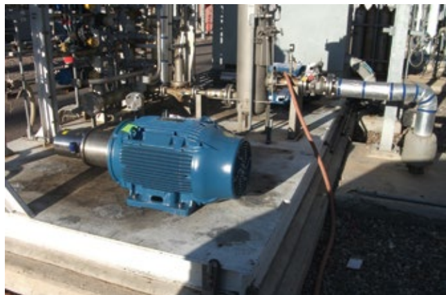
1. Existing pad for the retrofit fogger has plenty of space for the more compact, precise, and reliable pump/VFD drive unit (left), compared to the original belt-driven pump/motor system (right)
