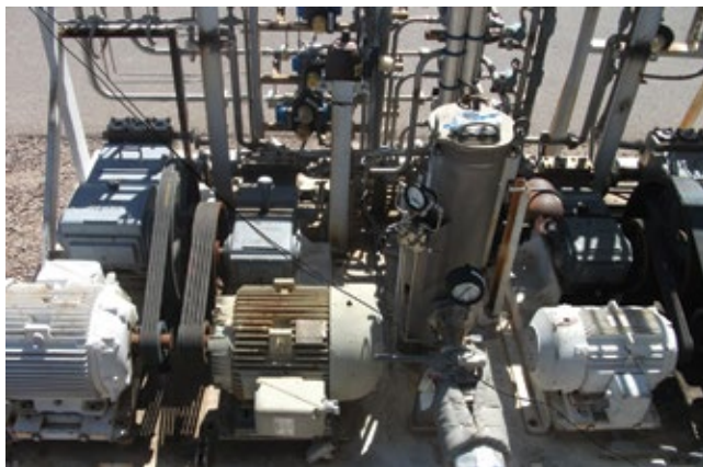
1. Existing pad for the retrofit fogger has plenty of space for the more compact, precise, and reliable pump/VFD drive unit (left), compared to the original belt-driven pump/motor system (right)
