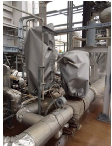
Uninsulated valve cover is typical of the freeze-protection steps taken to assure high availability in wintertime
