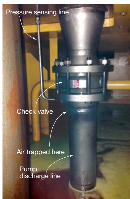
1. Before and after photos show the original arrangement of the lube-oil discharge piping at left and the simple mod at the right to protect against air-binding of the pump
