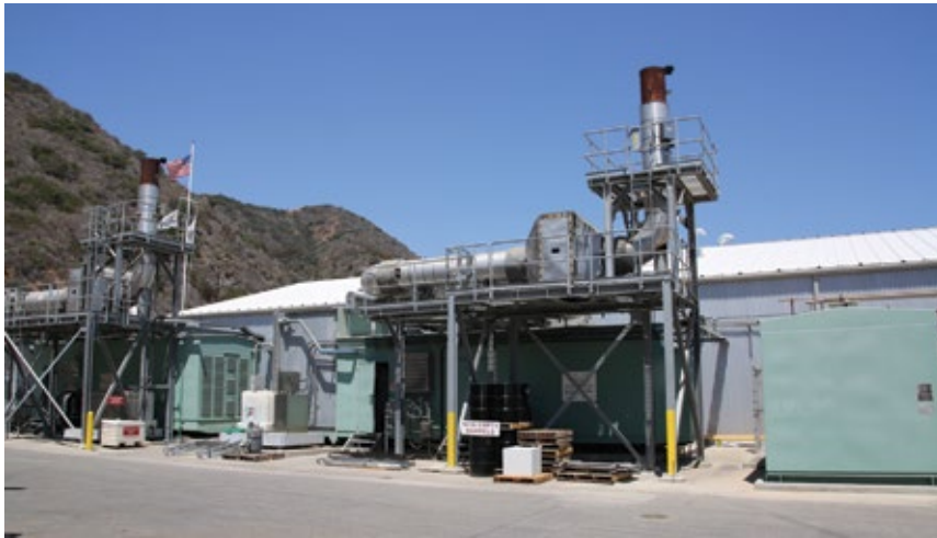
4. Diesel/generators , spanning unit sizes from 1 to 2.8 MW, were subject to ramp restrictions after SCR was added in 2004 for NO x control
