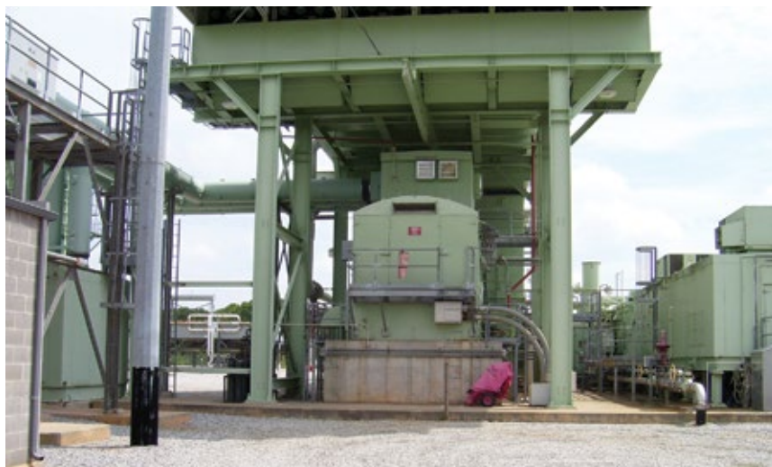
1. Making the workplace safer by facilitating access to equipment. Generator terminal enclosure before stairs were added is above; after, right
