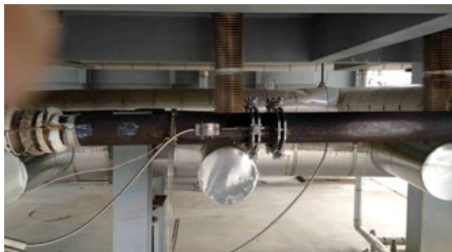
13. Prototype drain control system, on a superheater here, has been installed on three HRSGs to date
