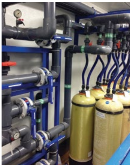
2. Original arrangement of 16 mixed-bed bottles jammed in a stationary truck trailer (left)
