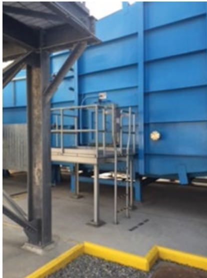
6. Several platforms and access doors were added to facilitate inspection and maintenance of the GT exhaust duct
