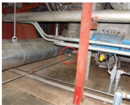
1. Manual drain valve shown after new piping was installed. Original configuration blew high-pressure combustion air into enclosure and exposed operator to numerous hazards
