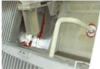
**19, 20. Achieving maximum performance** involves thorough inspection and the plugging of the smallest leaks with red gasket-forming silicone (above) and monitoring of fin condition and continually repairing damaged areas (right)
