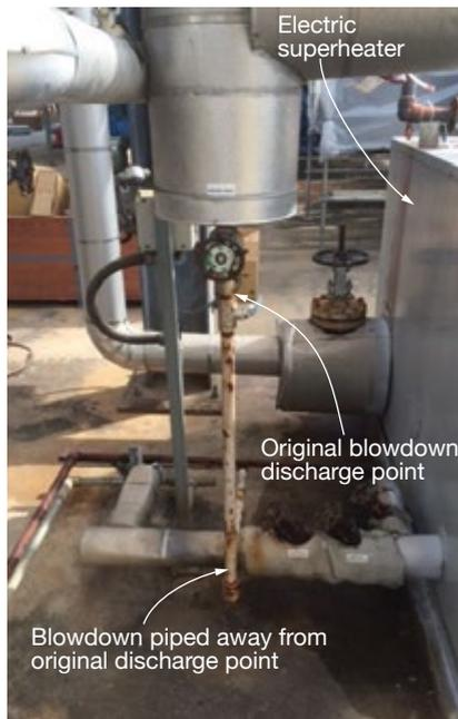
**1. Blowdown discharge location** for Effingham's auxiliary boiler was moved to prevent steam entry into the electric superheater
