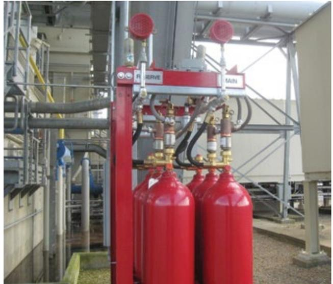
**2. High-pressure CO<sub>2</sub> systems** were added to serve the load tunnel (left) and collector cabinet (right)
