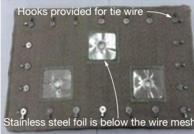
**8. Stainless-steel-reinforced high-temperature cloth insulation** protected by stainless foil and secured to the exhaust casing using stainless mesh is Arnold's recipe for success
