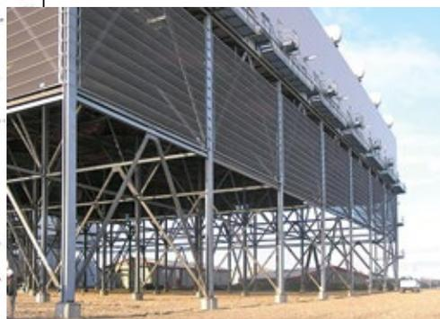
**2. Windscreens and shields are designed to reduce negative airflow patterns. Shown here is an example of a fixed screen**
