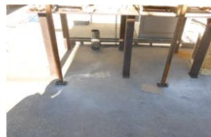
**2. Legs supporting trolley system** were bolted to the concrete pad to stabilize lifts
