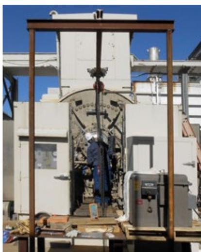
**3. Collector rings** are heated in oven (foreground, right of center), removed from oven, attached to chain-fall, lifted, and trolleyed to the generator
