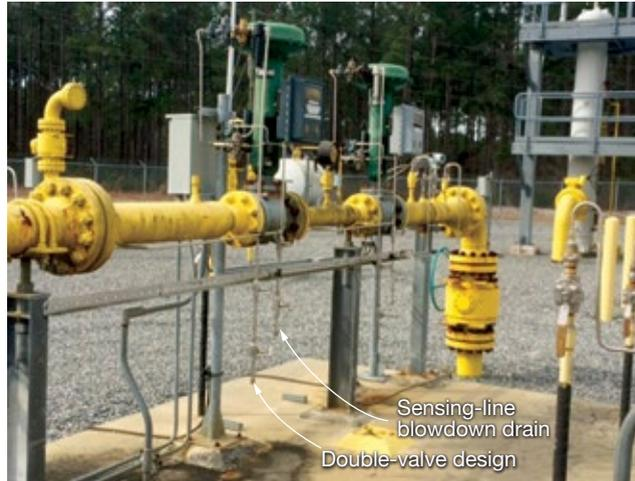
**4. Sensing lines** for fuel-gas-train control valves were equipped with drains and double valves to mitigate freeze-up in winter
