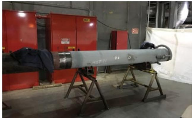
**2. New HP bypass desuperheater** has welds 10 ft farther downstream and includes a liner
