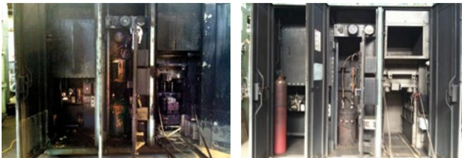
**7. Substation cabinet** fell victim to fire (left) and was restored using CO<sub>2</sub> (right)
