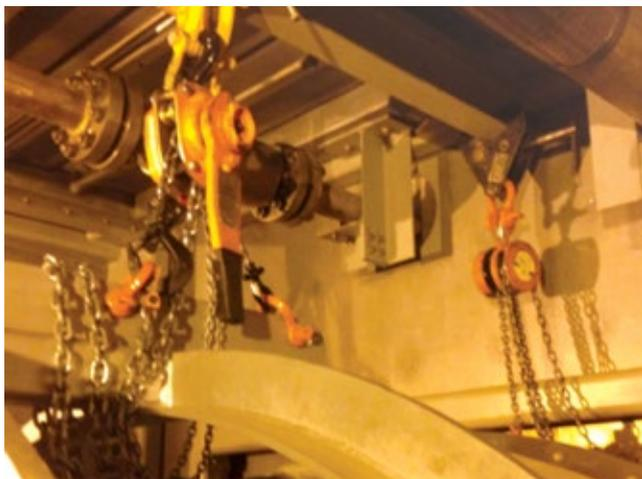
5. Exhaust diffuser and clamshells are rigged for removal
