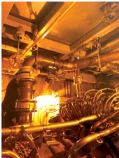
**3. Air piping** over the engine is rigged for bleed-valve removal
