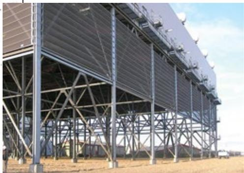
**2. Windscreens and shields are designed to reduce negative airflow patterns. Shown here is an example of a fixed screen**
