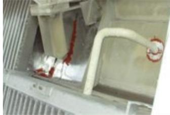
**19, 20. Achieving maximum performance** involves thorough inspection and the plugging of the smallest leaks with red gasket-forming silicone (above) and monitoring of fin condition and continually repairing damaged areas (right)
