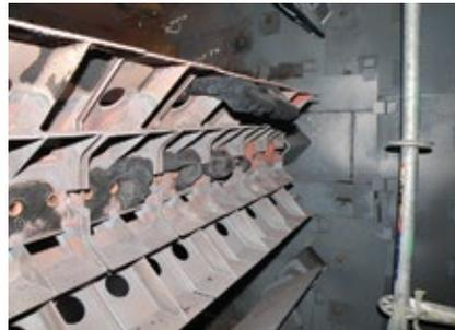
**4. A short flight could show locations of burner-tip coking.**
