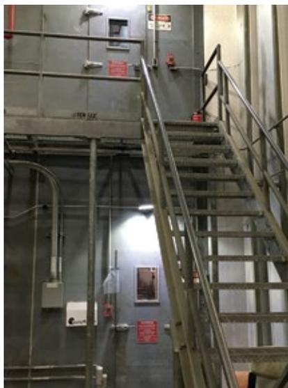
**5. Low-cost, low-maintenance package door windows** allow O&M personnel to assess interior conditions before entering a potentially hazardous situation
