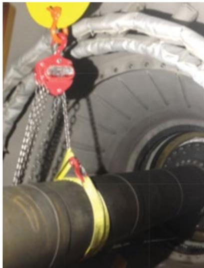
**4. Generator shaft coupling** is supported from fixture. The yellow lifting point for the shaft came with the package. Plant personnel removed the bulkhead in the generator compartment to access to the shaft easily
