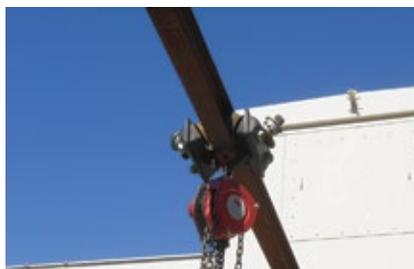
**1. Trolley system** with chain-fall hoist is used to move collector rings from oven to generator for installation
