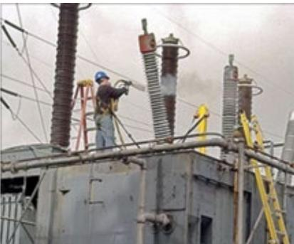
**10. Insulator cleaning** is fast and effective with CO<sub>2</sub>
