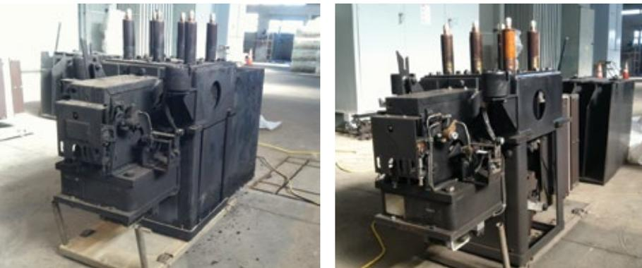
**8. Switchgear and breaker** cleaning with CO<sub>2</sub> is increasingly common. Before is at left, after at right
