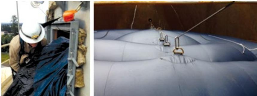
**6. Access door and platform** were added to accommodate the stack balloon (left); guy wire (right) holds the balloon during placement and is retracted during plant operation
