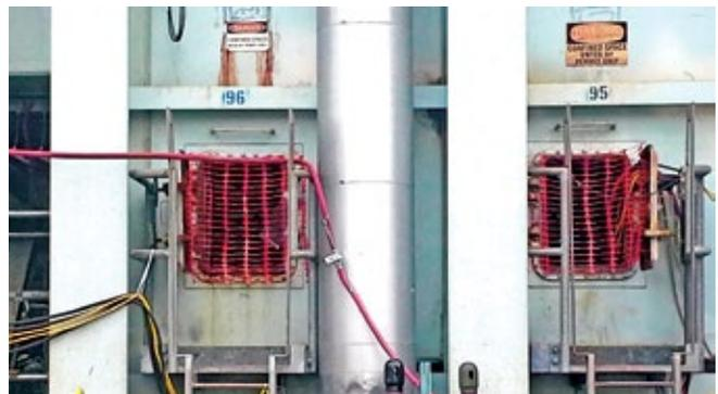
**7. Lower hatches for superheater and HP evaporator** access during outages. Temporary barricades are installed and lines for air, welding, and electric are secured
