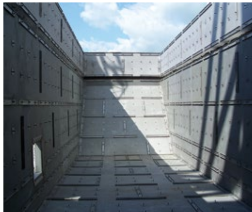
Internal liner: excellent (new)
