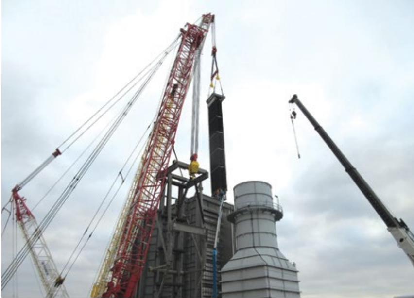
6. HRSG tube panel is put into place during construction
