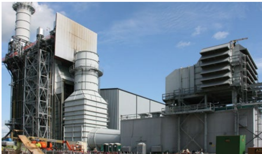
2. The heat shield located behind the GT exhaust stack allowed gas-turbine operation during construction and installation of steam-system components
