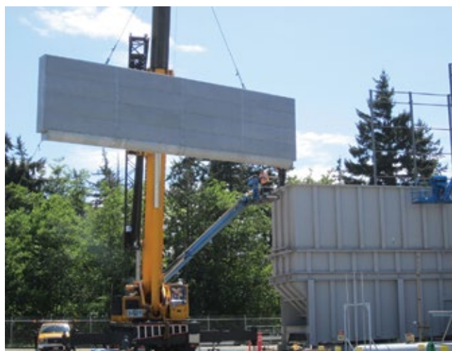
3. Baffle installation
