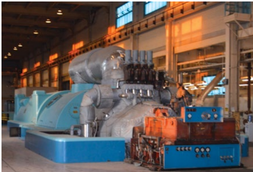
1. Vintage 160-MW steam turbine (left) was repowered at Victoria Power Station in 2007-2008. Internals of the unit's high- and intermediate-pressure sections are at right
