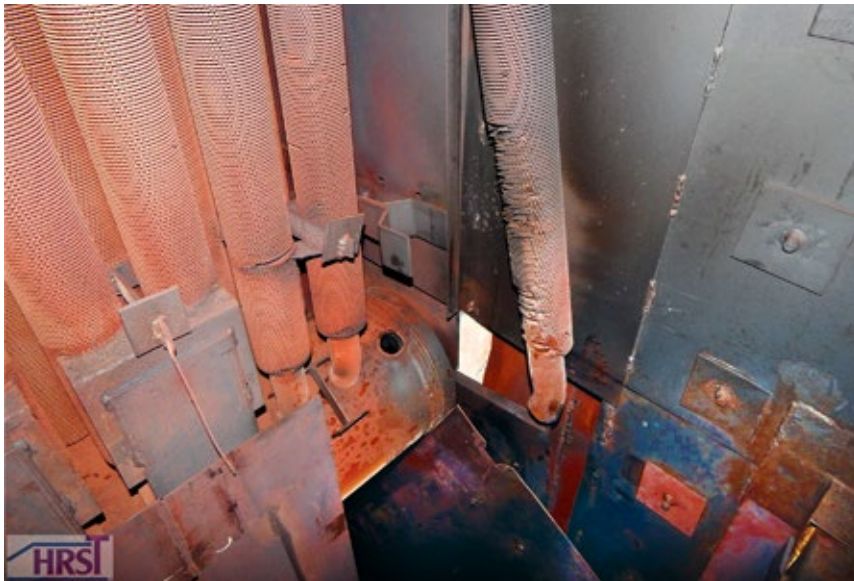
4. Tube-to-header weld failure was attributed to thermal quenching
