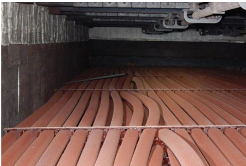
1. Bowed tubes were caused by overspray
