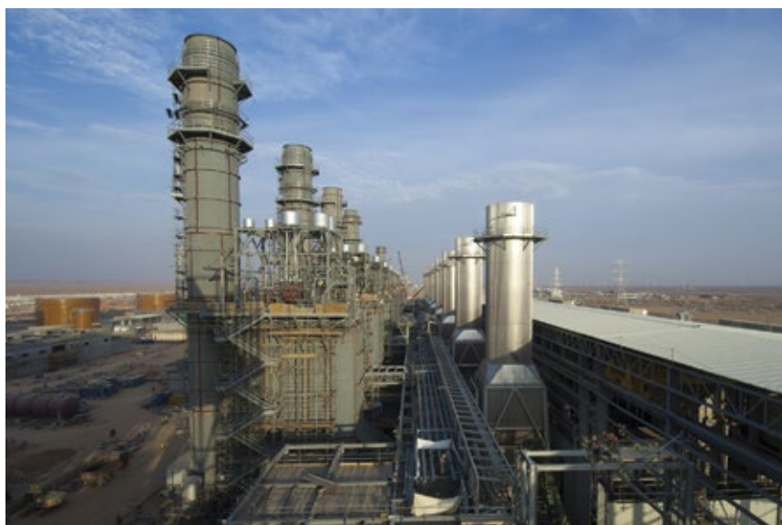
4. Saudi Electric's Power Plant 12 in Riyadh is equipped with 7FA.05 gas turbines capable of burning Arabian Super Light crude oil
