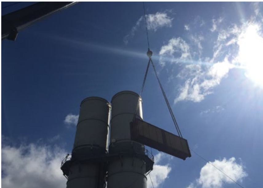
3. The crane will take up a significant amount of space during the project, so survey the laydown area carefully
