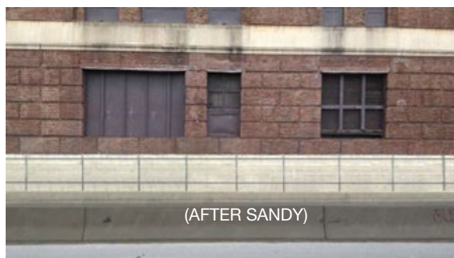
4. The seal perimeter at East River was hardened. Water ingress points discovered in abandoned doors and windows (left) were sealed with additional concrete barriers, brick, and mortar (right)
