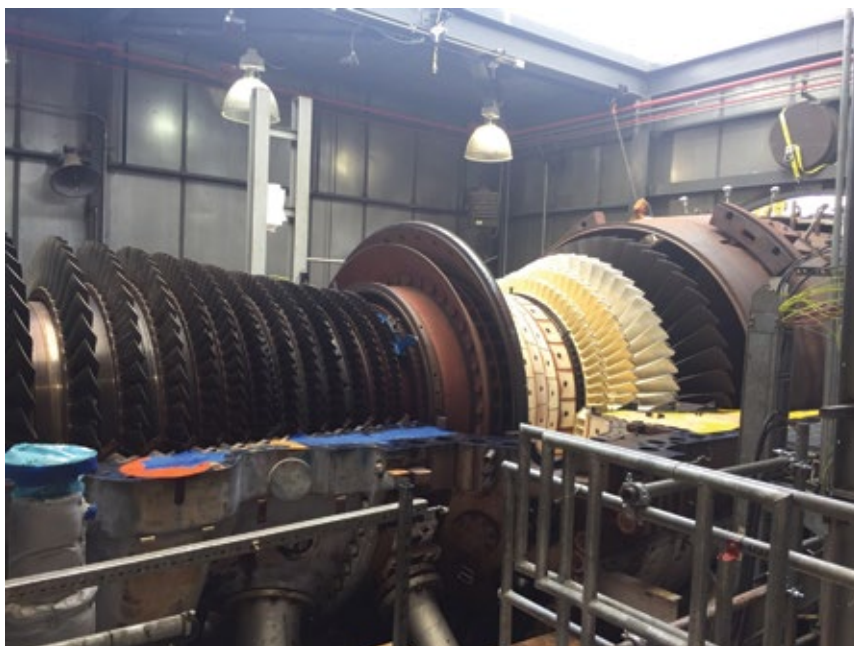
3. V84 gas turbine, rated 150 MW, began operating as a peaking unit in 2007
