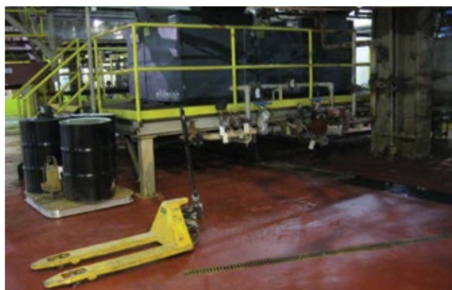
3. In all, 19 moats were installed at East River after the storm. As built, no moat existed at left; addition is at right
