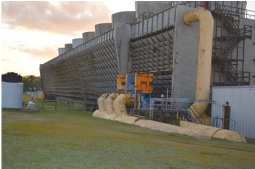
4. Cooling-tower and circ-water pumps are scheduled for overhaul to assure continued reliable operation
