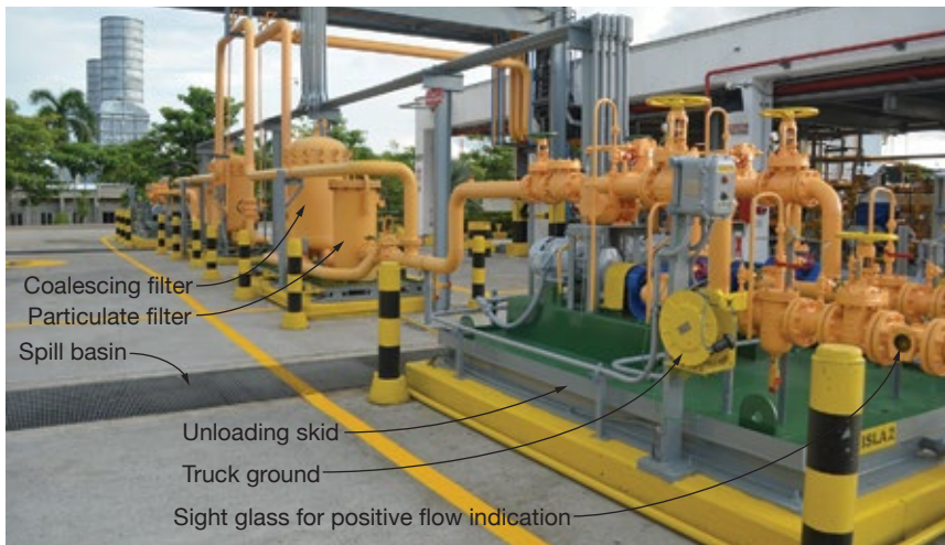
4. Unloading station is high-tech at Termocandelaria. Heavy video monitoring is in evidence to ensure safe operations. Lines painted on the deck ensure exact positioning of trucks to facilitate the connections of the trucks to the unloading skids. In the unlikely event that a spill occurs, it will be directed to the trench under the grating which connects to the oil/water separator. Coalescing and particulate filters serving adjacent unloading stations are arranged in parallel and are able to process oil from two unloading skids. Note, too, trucks must be certified "clean" before handling oil
