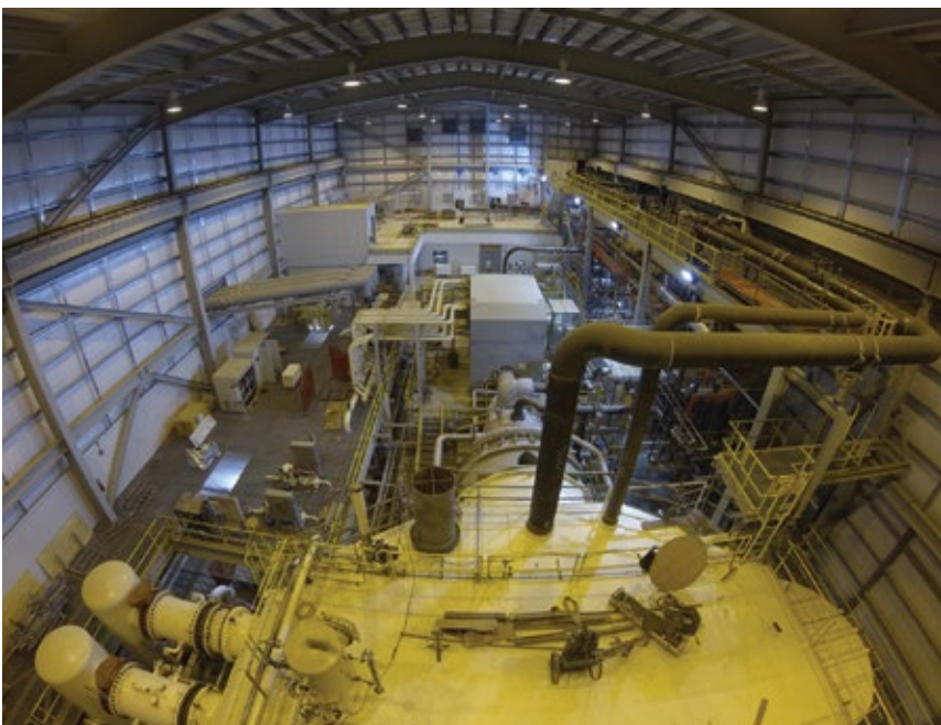
4. VAX steam turbine features an LP module (foreground, just beyond the condenser in yellow), a generator (box in center), and an HP module geared down to 3600 rpm (above)
