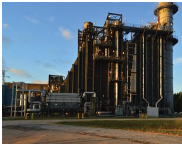
2. Gray-market gas turbine package (left), a Mitsubishi 501F, was purchased for the repowering, along with a Vogt (Babcock Power) HRSG (right)
