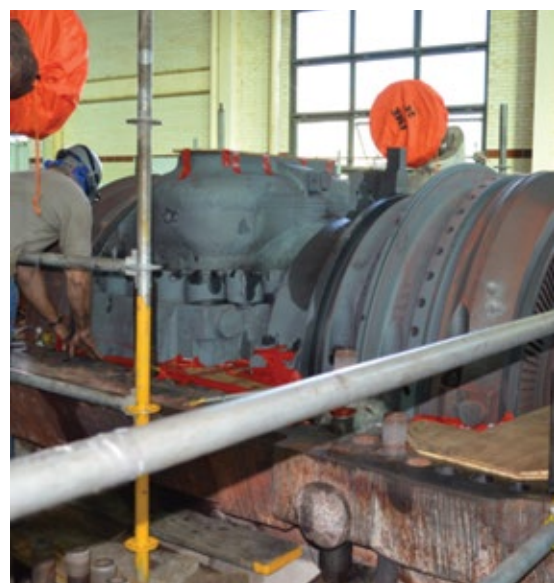
1. Vintage 160-MW steam turbine (left) was repowered at Victoria Power Station in 2007-2008. Internals of the unit's high- and intermediate-pressure sections are at right
