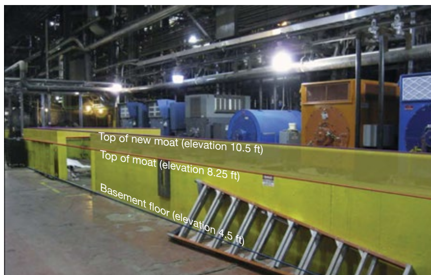
2. Moats around critical equipment at basement level were raised by more than 2 ft (left); moats were added in other areas—such as around control cabinets (right)
