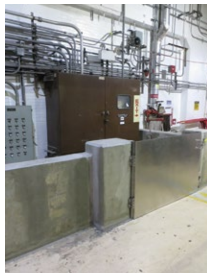
2. Moats around critical equipment at basement level were raised by more than 2 ft (left); moats were added in other areas—such as around control cabinets (right)
