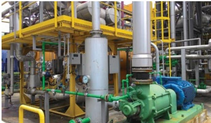
**1. Vacuum pump** was installed to supplement the starting steam-jet ejector and reduce the time to breaker close
