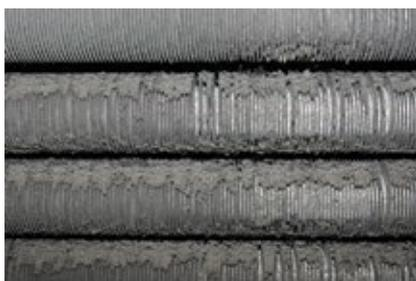
**4. Fouling** (fibers, dust, pollen, etc) of ACC bundles restricts air flow, limits heat transfer. Deposits shown have a fairly weak bond, but 50% closure of heat-transfer surface
