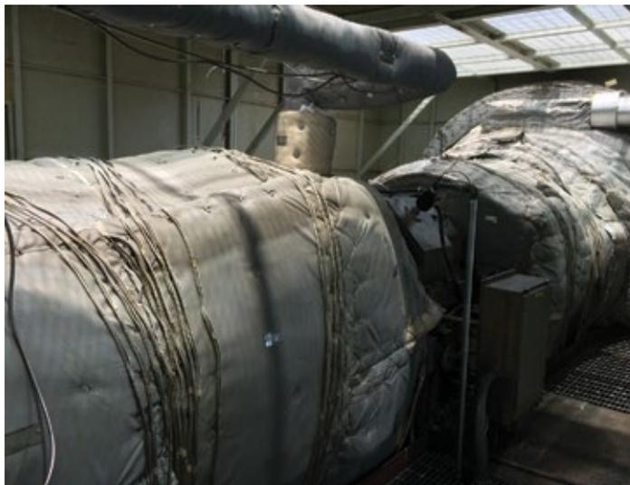
**A10 steam turbine** has heating blanket to enable fast starting
