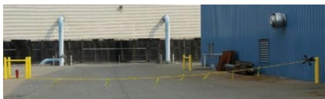
**Simple solution.** Lightweight plastic chain is easy to see and deploy to prevent exposure to hazardous materials during unloading operations
