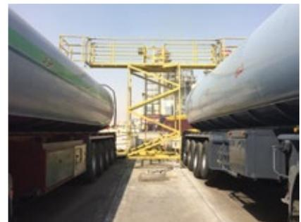
**1. New platform, designed by plant staff, serves two oil tankers simultaneously**
