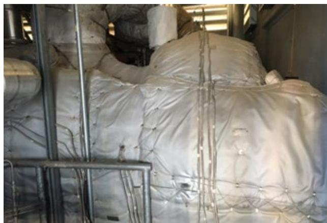
Blankets for heating the HP cylinder (left) and crossover (right) to enable faster starts
