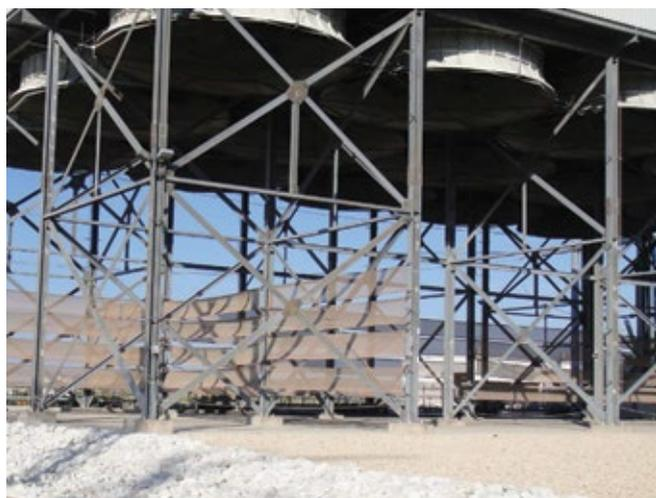
**11. Placement of ground-level screens** was based on results of CFD modeling
