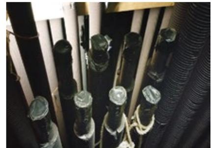
**13. Tube leak repair required access four rows back**
