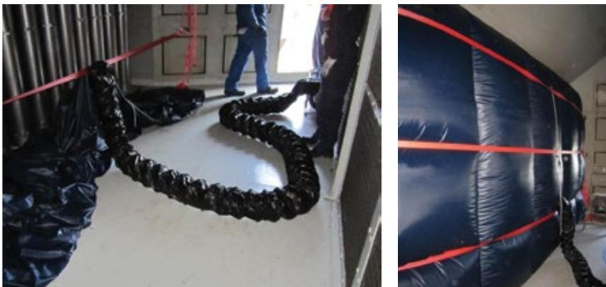
Duct balloon of this size certainly is easy enough for one person to install and remove
