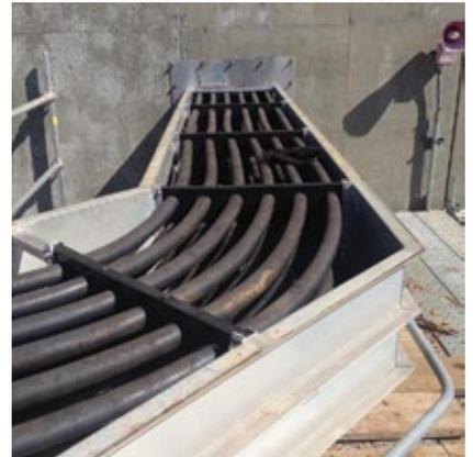
**3. Long-lived spacers** of high-density polyethylene were installed without incident
