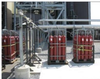
**46. Hydrogen tank farm** is typical of that installed at many plants
