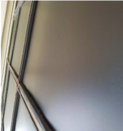
**4. HDPE sheets** between the air-inlet pocket frames and filters seal off air flow through the gas turbine, keeping relative humidity below 10%
