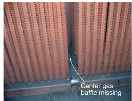
**3. Troublesome gas baffles** should be repaired or replaced, not removed. Latter can lead to downstream overheat failures
