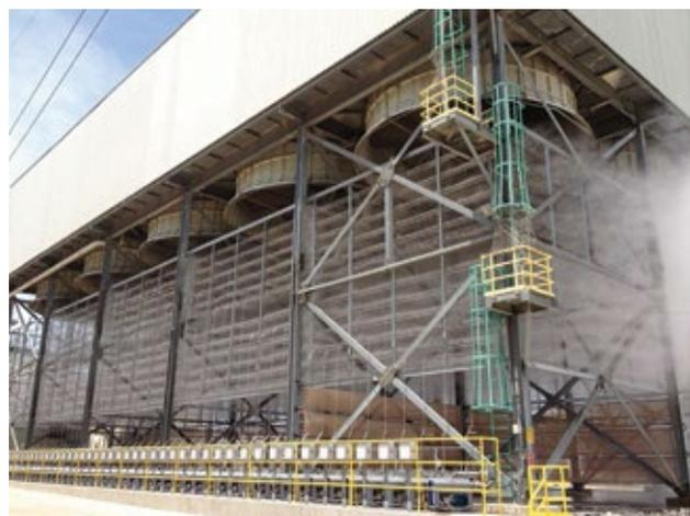
**12. Fogging system** installed at Midlothian to demonstrate performance improvement increased steam-turbine output by 5.8 MW at 100F and 30% relative humidity
