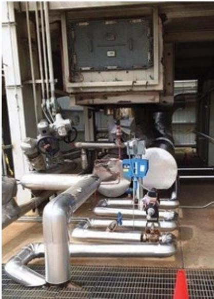
**6. Problem solved** with new automated drain line and addition of access doors
