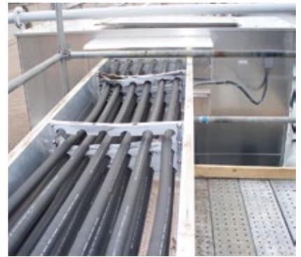
**1. Support blocks deteriorated** allowing cables to sag
