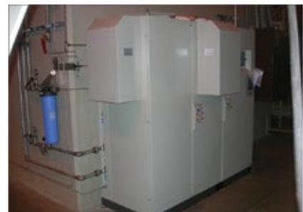
**47. Onsite hydrogen generators** are an alternative to receiving hydrogen by truck, in bottles
