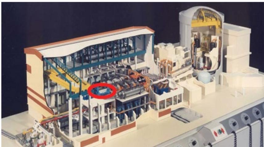
**48. Powerplant model** shows the revenue machine (generator, encircled by red ellipse) virtually hidden by other equipment
