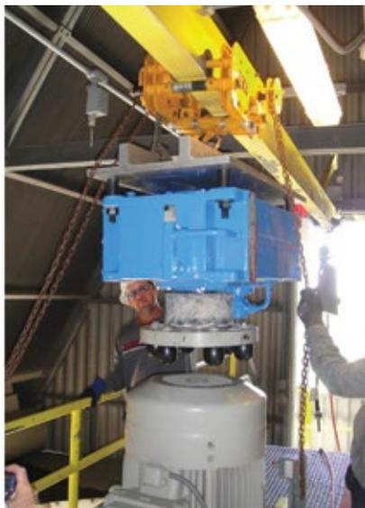
**10. Low-profile lifting devices** are used to remove fan motor drivers and gearboxes
