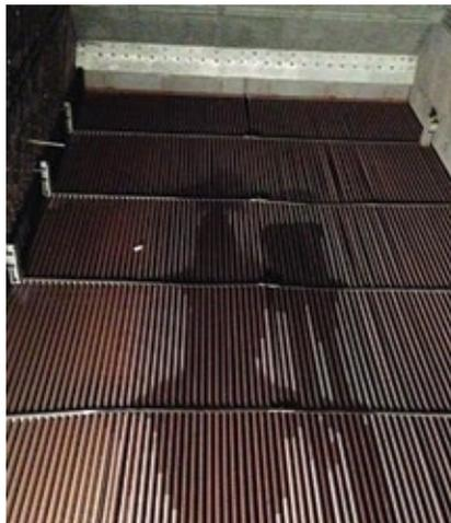
**12. This leak was found by filling the reheater with water via RH attemperator sprays**
