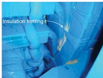
12. Endwinding vibration is a major cause of dust generation
