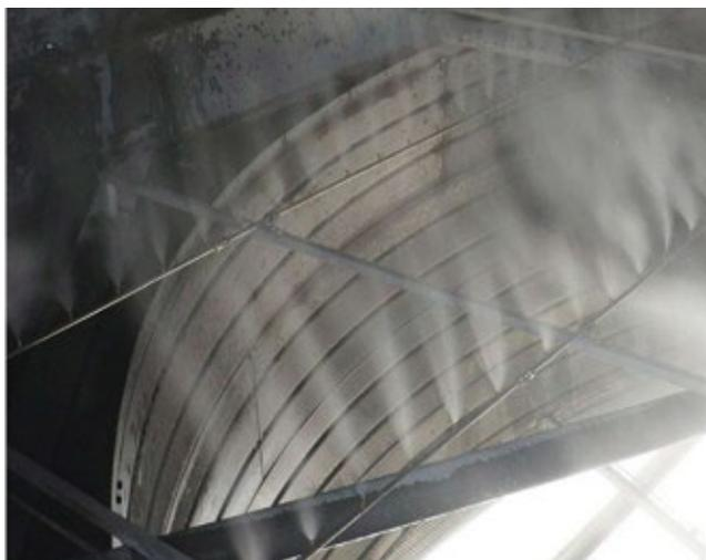
9. Plumes from fog nozzles, installed to improve thermal performance, are visible for only a few feet before evaporation
