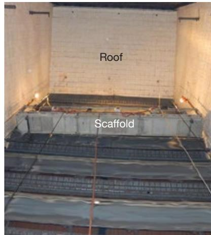
**7. Scaffold** at left is prepared for duct-burner baffle-reinforcement at right
