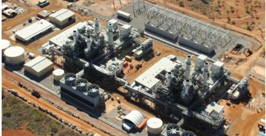
**5. Diamantina Power Station**, which produces 240 MW with two 2 × 1 power blocks, took steps to reduce dissolved oxygen in cycle water
