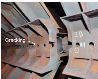
**2. Deterioration of duct-burner baffles and runners can cause excessive downstream temperatures**
