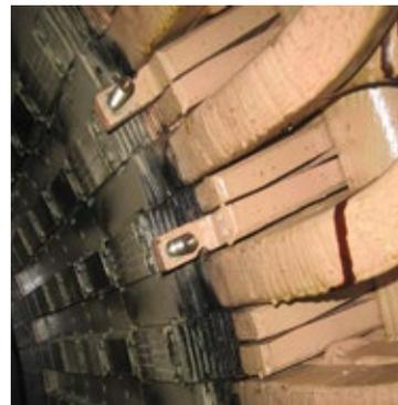
**40. Mechanical vibration** contributes to insulation degradation
