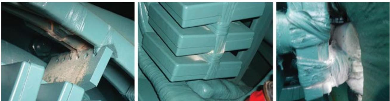
**34. Several cases of endwinding and connection-ring vibration** were found during generator inspections. At left and right is connection-ring dusting on blocks/ties, in center is greasing on series loop blocks
