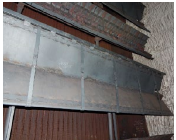
3. Burner baffles often support the burner elements. Baffles prone to sagging and buckling (above), typical for one manufacturer's offering in the 1999 to 2004 period, can be replaced with a stronger and more durable design (below)
