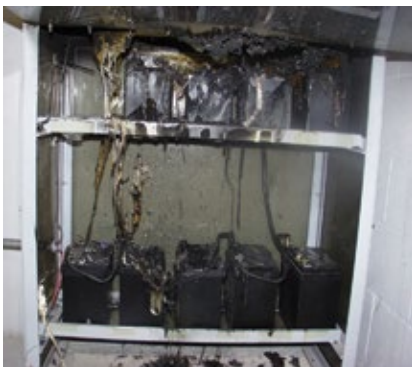
4. Batteries demand your attention. A thermal runaway can occur when a battery is being charged and the heat generated exceeds the rate at which it can be dissipated through the battery case to the environment
