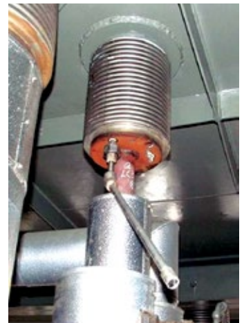
4. Shoring up economizer tube return bends with supports shown can help prevent cracks from corrosion fatigue (above)
