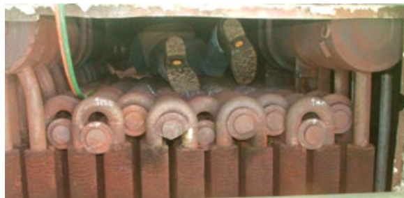
4. Shoring up economizer tube return bends with supports shown can help prevent cracks from corrosion fatigue (above)
