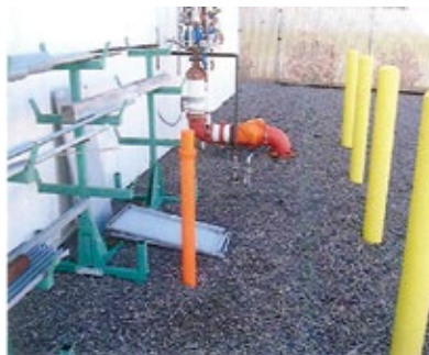
9. Cathodic protection system test station, post-mounted and easily seen, is installed near where the natural-gas line enters. System is of the non-powered (sacrificial) type
