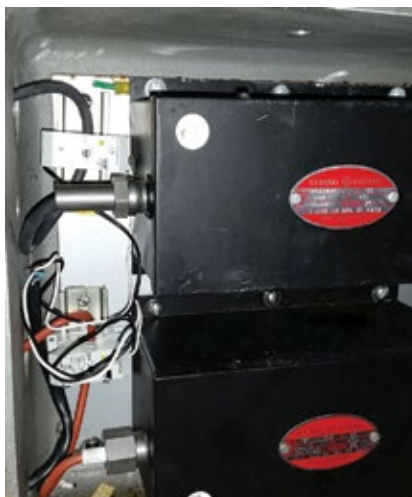
1. Current transformers are installed in the ignition-transformer cabinet
