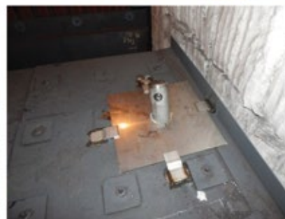
2. Cameras installed in the duct-burner area can wirelessly relay images back to the control room to check in real time for flame impingement on tubes, which will help prevent creep and overheat damage
