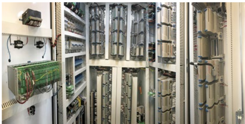
2. Cabinet layout was an important consideration in replacement of GT OEM control system at this peaking facility; some panels were relocated to make the I/O flow more logically
