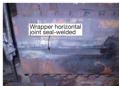
14. Some users say welding strips of plate to the outside horizontal joint is the most effective way to eliminate wrapper leaks
