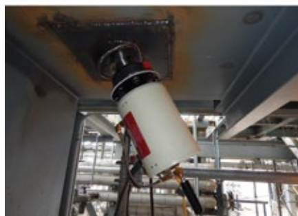
2. Cameras installed in the duct-burner area can wirelessly relay images back to the control room to check in real time for flame impingement on tubes, which will help prevent creep and overheat damage
