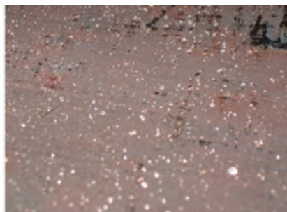
9. Duct inspection showed water beading from the Anodamine treatment at the tube inlet (left) and on the lower-duct metal surface (right)
