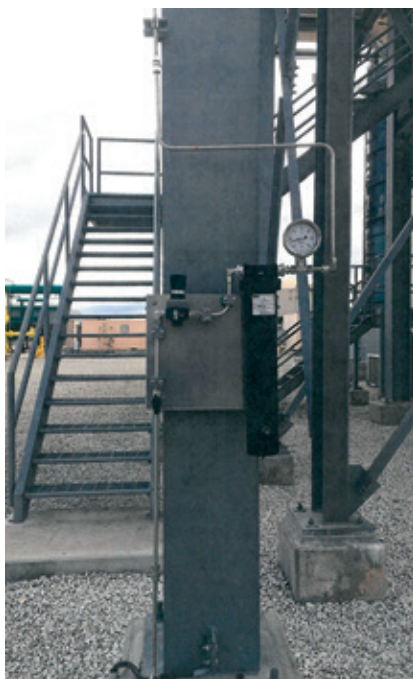
3. Purge-air station is equipped with an additional desiccant air dryer, pressure regulator, and pressure gage with isolation valves
