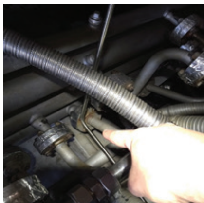
2. Technician points to the ring header-to-pigtail flange (left) where the gasket (right) was damaged and allowing leak-by
