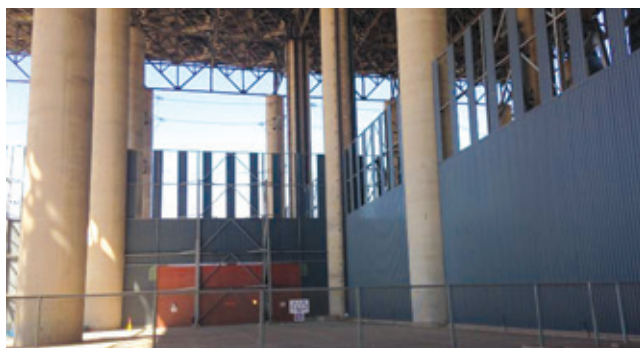
3. The at-grade wind walls at Medupi (photo) were extended from Matimba's 33 ft to 47 ft
