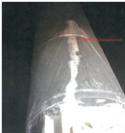
1. Unit 3 isophase bus bar (A phase) presents evidence of moisture intrusion
