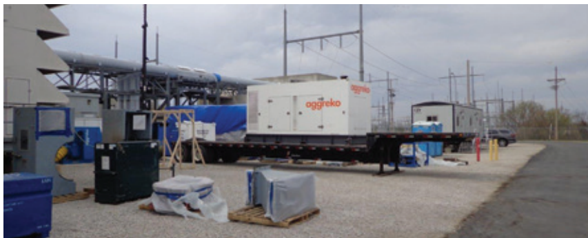
1. Rental generator gobbles up site space and requires ongoing support by plant staff for refueling, etc
