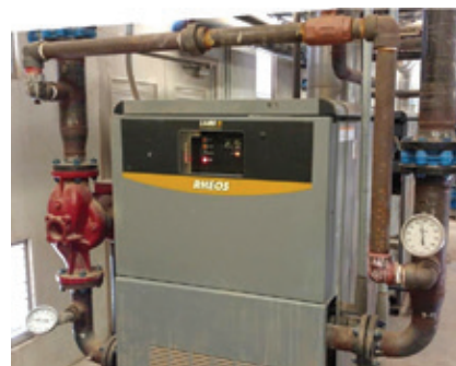
3. Gas heater has a bypass throttling valve to maintain the recommended minimum inlet temperature
