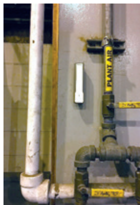
4. ANThill locator beacons are installed at critical locations in the plant
