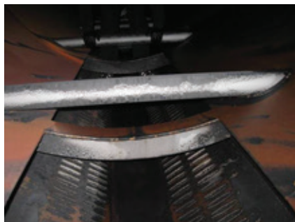
8. MEA/Anodamine treatment mitigated upper-duct corrosion found during the 2011 inspection (left). Photo at right was taken in 2016
