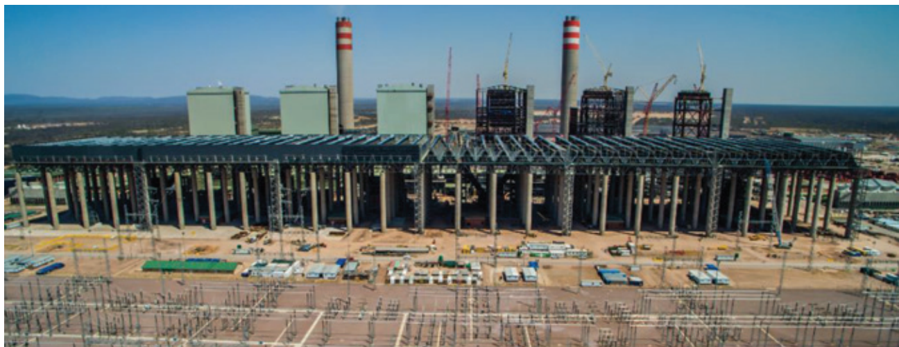
1. Eskom's Medupi Power Station in South Africa, rated 4764 MW, features the world's largest air-cooled condenser. Three of the plant's six coal-fired units were in commercial operation at the time of the 2017 ACC Users Group meeting in Las Vegas. According to published reports available to the editors, Medupi will achieve full commercial operation in 2020
