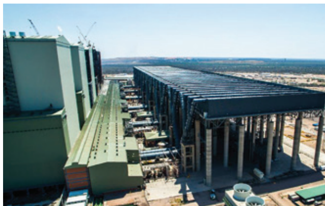
2. The Matimba Power Station's ACC (left) provided valuable lessons learned for the nearby Medupi (right)—especially regarding site layout, fan height, and wind walls
