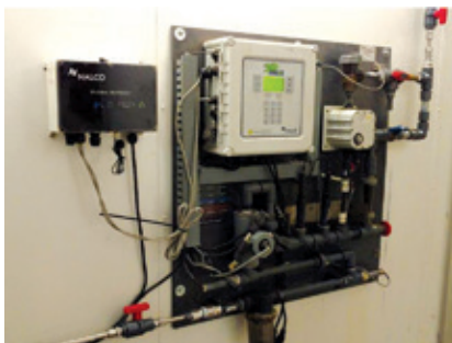
2. 3D TRASAR controller monitors KPIs—such as pH, conductivity, turbidity, etc—in real time
