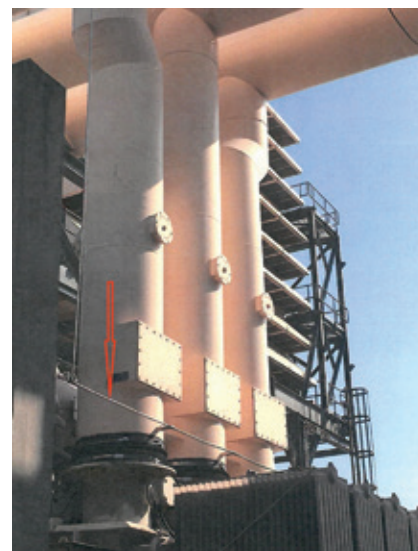
5. Purge air is delivered to the primary sides of the two auxiliary transformers
