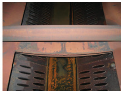
8. MEA/Anodamine treatment mitigated upper-duct corrosion found during the 2011 inspection (left). Photo at right was taken in 2016
