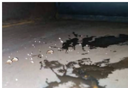
9. Duct inspection showed water beading from the Anodamine treatment at the tube inlet (left) and on the lower-duct metal surface (right)
