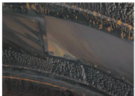
10. Protective shroud for the steam-turbine expansion joint was found in better condition in 2016 after MEA treatment (right) than it was in 2011 (left)
