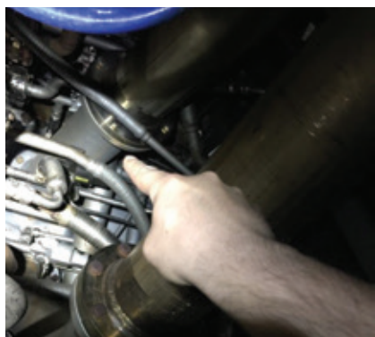
3. Flange, typical of those in ninth- and 13th-stage extraction lines (left), was broken to replace damaged gasket at right
