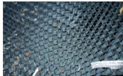
2. Biological growth after switching to calcium hypochlorite on demand
