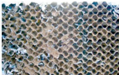
1. Biological growth while using batch addition of sodium hypochlorite
