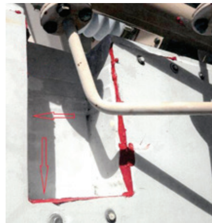
2. Bushing enclosure was modified during plant construction. The flaw introduced has been repaired
