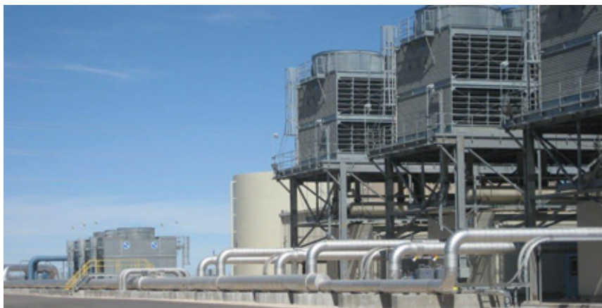
1. Inlet air chillers for the two gas turbines are arranged at groups of three (far left and right) with the storage tank in between
