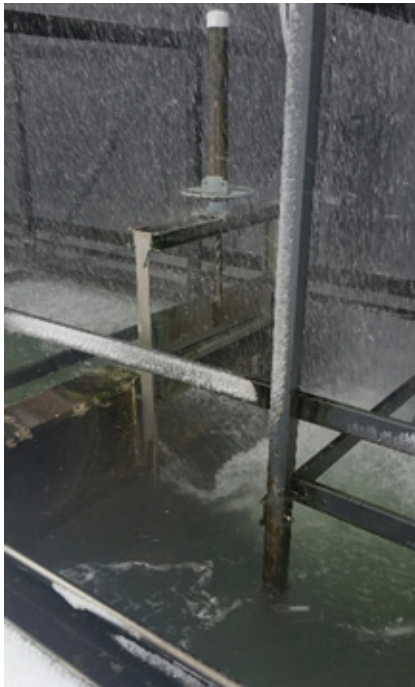
3. Since the original installation, plant personnel modified the weir compression panels into knife gates operated by valve wheels
