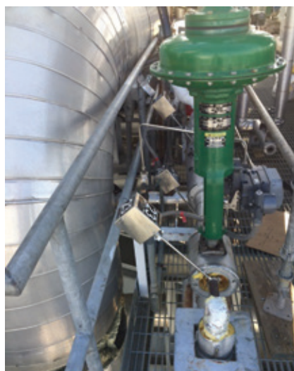
1. Acoustic monitor is installed on reheat attemperator spray valve as part of the EPRI-sponsored project at T A Smith
