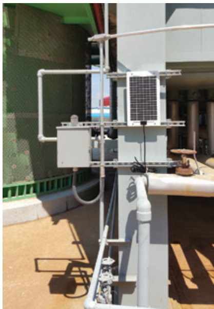
3. Solar panel keeps batteries powering wireless instruments charged
