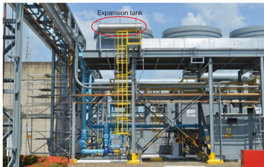
3. Expansion tanks for the closed cooling systems are located high above the generators. Simplified system schematic is in Fig 1
