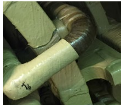
B16. New tie stands out after removal of the old tie and blocking, cleaning, and addition of new conforming material
