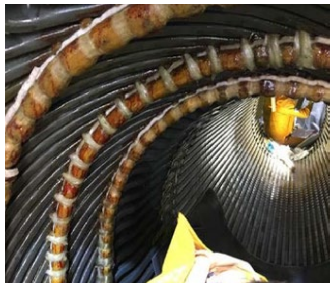
B18. Endwinding structure after completion of repairs
