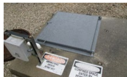
Original manhole arrangement is at left, new hinged manhole cover at right
