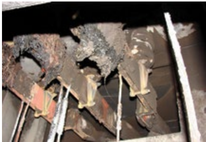
B34. Overheating attributed to a lack of maintenance destroyed this non-seg bus
