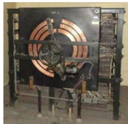
C25. Excitation systems have evolved over the years from rheostats prior to the 1950s (photo) to electromechanical amplifier in the 1950s and 1960s, to magnetic/analog in the 1970s and 1980s, to today's digital excitation systems
