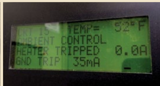
Add smart-panel amp indication on each circuit as well as a light to visually indicate when the circuit is energized to facilitate walk-down verification of proper operation
