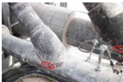
9. P91 large branch connections are known for their susceptibility to flank-side cracking
