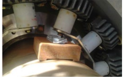
E4, E5. Ground alarm following a shutdown for lack of market demand alerted staff to rust accumulations on rotor and exciter components caused by condensation/improper layup
