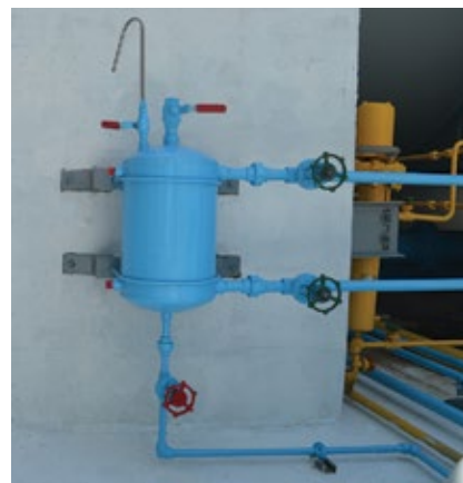
2. Chemical addition system for corrosion control protects the closed cooling system
