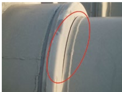
B33. Excessive movement of expansion bellows is conducive to cracking damage
