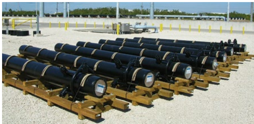
6. New, extended-length HP attemperators provide more residence time for the evaporation of spray-water droplets
