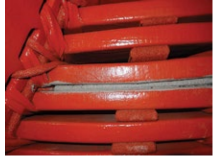
B7. Discharge oxidation at phase splits is easy to see
