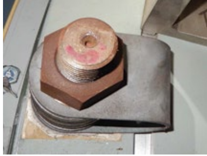
B6. Proper torqueing of keybars is critical in preventing their fracture
