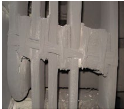
B12. Original blocking and tie arrangement does not meet quality standards
