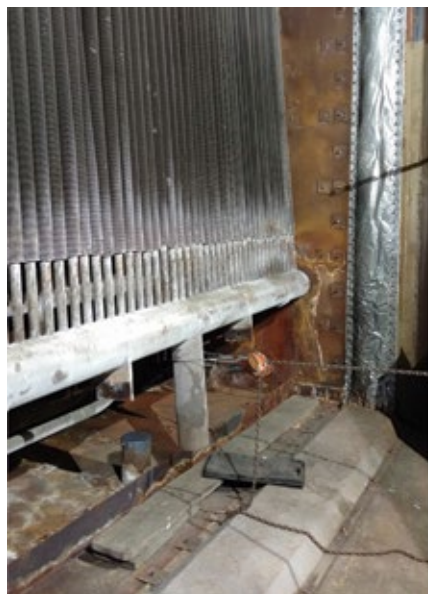
4. Preparation of the lower-header area for inspection and weld repair was facilitated by the model
