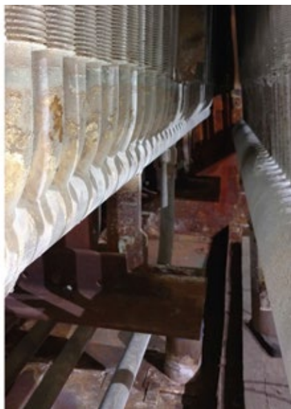
4. Preparation of the lower-header area for inspection and weld repair was facilitated by the model
