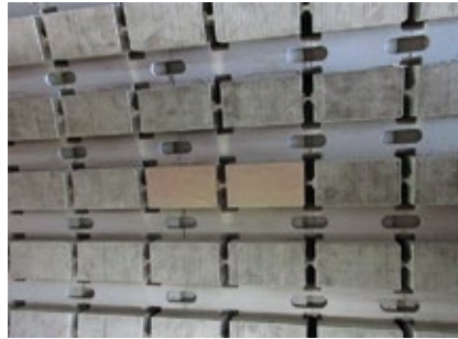
B23. Damaged areas had a coat of red dye applied to weep into the laminations before coating with a buff paint
