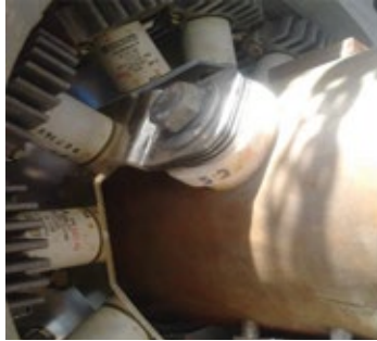
E4, E5. Ground alarm following a shutdown for lack of market demand alerted staff to rust accumulations on rotor and exciter components caused by condensation/improper layup
