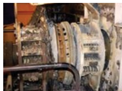
D7. Collectors are the most significant contributor to operations-caused forced outages
