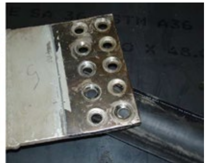
B32. Improper bolting and lack of maintenance are conducive to damaged contact surfaces at connection points
