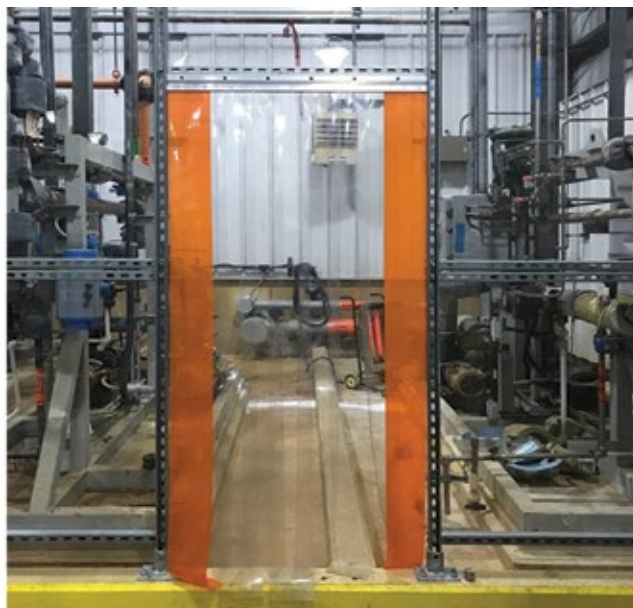
Protective barrier of transparent Plexiglas® is supported by Unistrut® frame (left); entry curtain of chemical-safe plastic is at right
