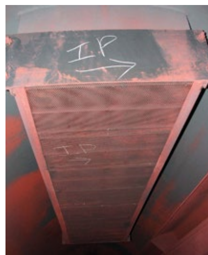
2. Perforated plate incorrectly installed under the mesh pad (should be above pad)
