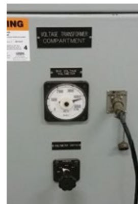
3. MTAP installed at switchgear compartment is monitoring voltage
