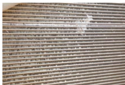
3. Blockage of air passageways prevents optimal heat transfer, reducing thermal efficiency
