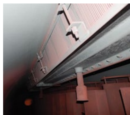
1. Condensate trap on baffle-style (chevron) steam separator
