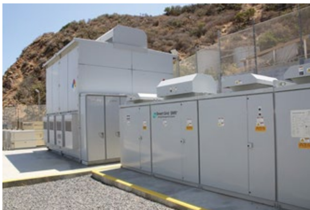
Twenty-three micro-turbine/generators (center of photo at left) are adjacent to the 1-MW battery and power conditioning system—all located in the enclosed area. Battery and PCS details are at right
