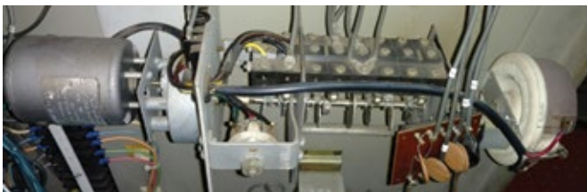
1. Motor-driven set point 70-R4 is used for speed/load adjustment (left). Limit switches and associated cams for setting 70-R4 operating points are shown at right
