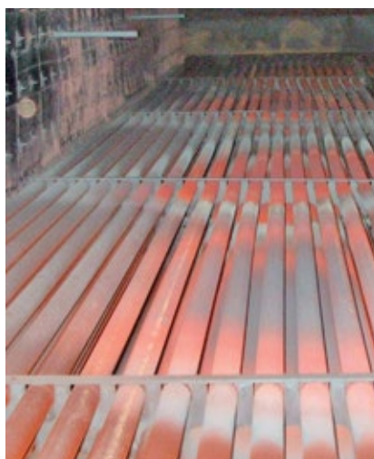
8. Flame impingement on tubes
