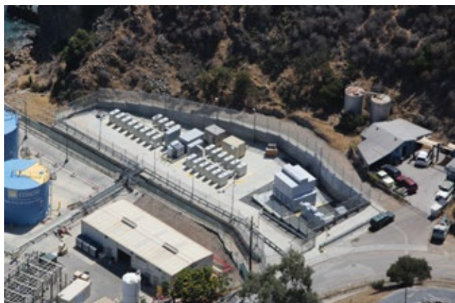
Twenty-three micro-turbine/generators (center of photo at left) are adjacent to the 1-MW battery and power conditioning system—all located in the enclosed area. Battery and PCS details are at right
