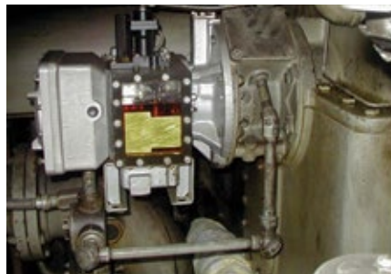
2. A typical fuel regulator by Young & Franklin is at left, the plug providing access for gag adjustment is highlighted at right
