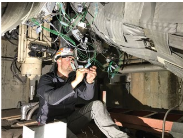
4. Warming system for a D11 steam turbine can be installed within a 10-day window, according to Arnold Group (left). It can bring the turbine from a cold state to hot-start condition within 2 to 2.5 hours (right)
