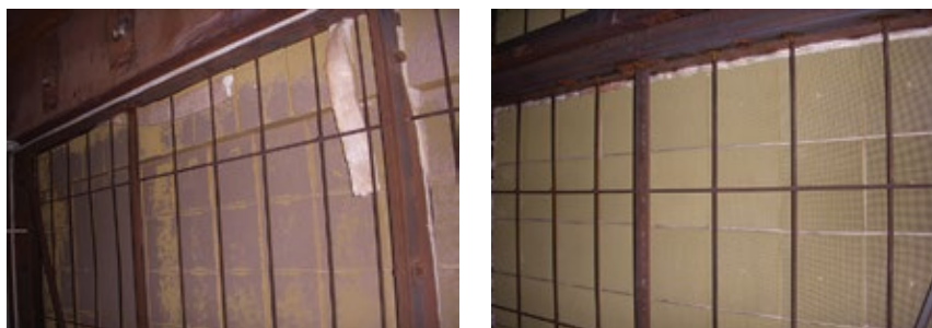
Before/after SCR catalyst cleaning left/right
