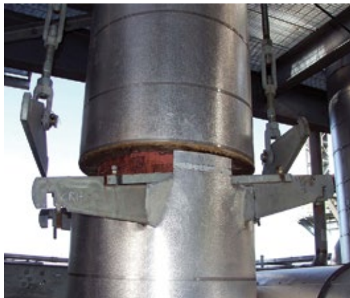
11. Effects of water hammer on cold reheat line
