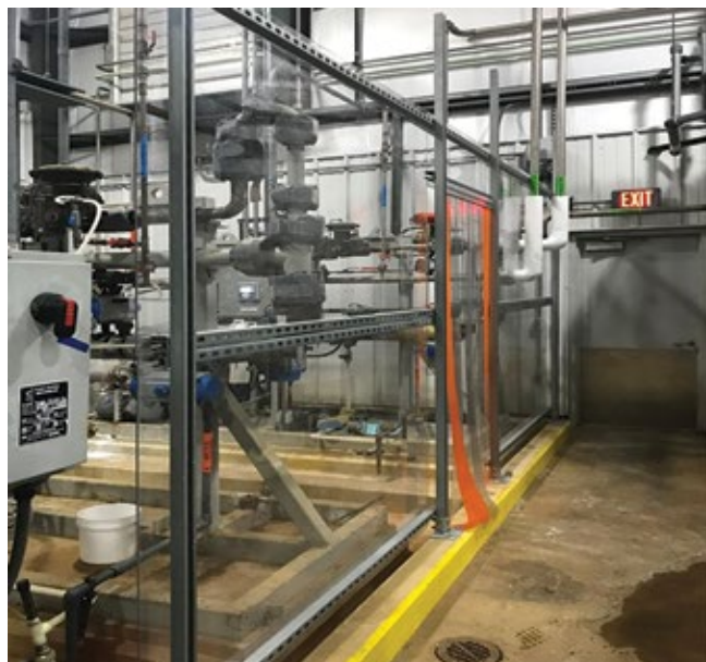
Protective barrier of transparent Plexiglas® is supported by Unistrut® frame (left); entry curtain of chemical-safe plastic is at right
