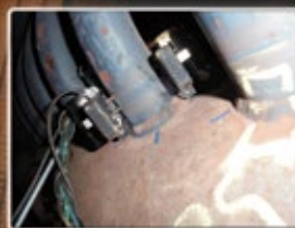
Claw Tool for Tube to Header Weld Cracking
