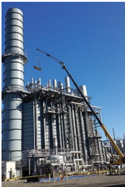
Crane picks section of catalyst (left) and moves it to ground (above) for cleaning
