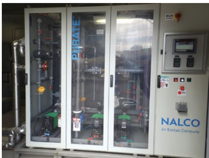
High Desert's biocide, chlorine dioxide, is made onsite
