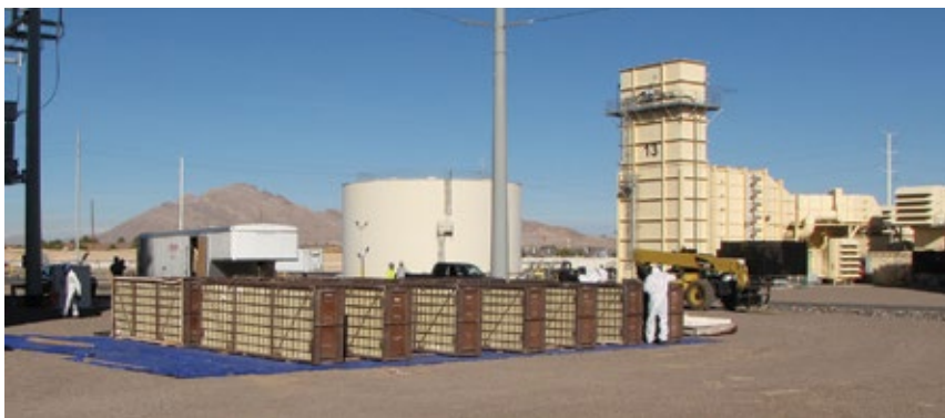
Crane picks section of catalyst (left) and moves it to ground (above) for cleaning
