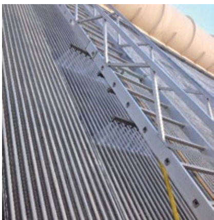
5. Cleaning is performed most often by a semi-automatic spray system traveling on a track
