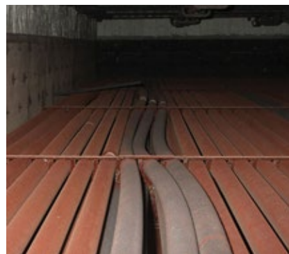
3. Reheater tubes stressed because of water leakage through desuperheater
