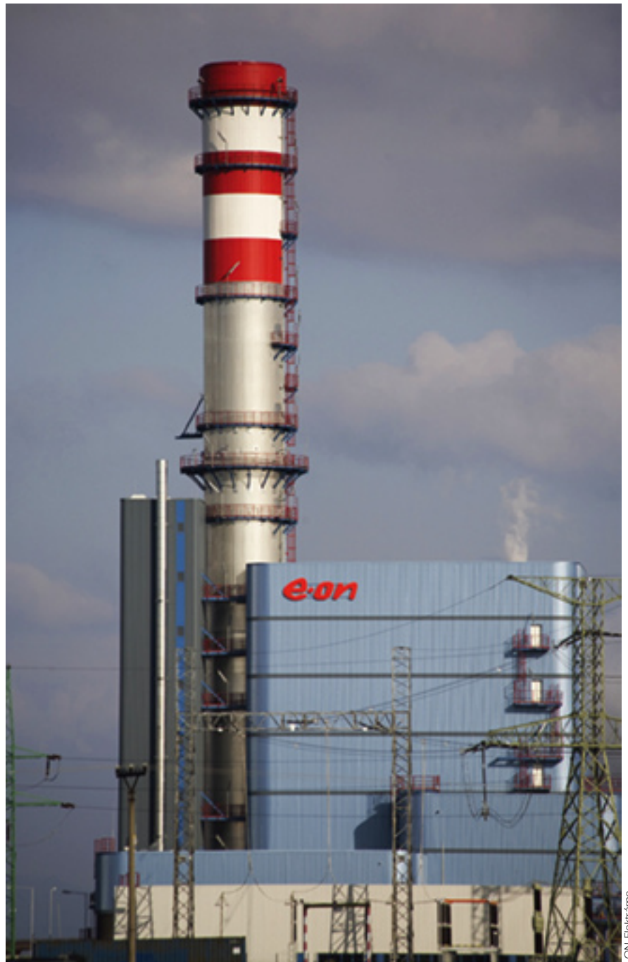
A 434-MW combined-cycle merchant plant in Malzenice, Slovakia's first private powerplant, was completed in late 2010 by E.ON Elektrárne.
