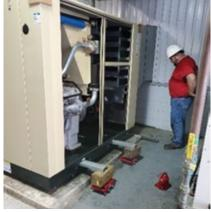
**9. Tight squeeze** moving the new compressor into existing space
