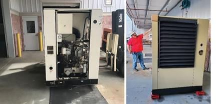
**8. The new compressor**,  $89 \times 54 \times 76$  in. high and weighing nearly 5500 lb, is lifted (left) to allow the placement of four caster rollers (right) for maneuverability
