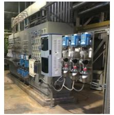
**1. Upgraded and expanded** panel/ instrumentation underpins the KPI index developed for tighter control of water chemistry
