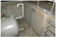
1. Pipe extension promotes safety by eliminating the need to enter the pit to pump out the tank
