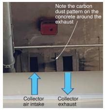
2. The collector air-intake and exhaust ports were in close proximity to each other
