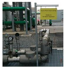
7. Permanent signage for each sump has sump name and discharge location
