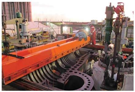
**3. Portable mill set-up** on the horizontal joint helped to correct casing distortion **COMBINED CYCLE** JOURNAL, Number 67 (2021)
