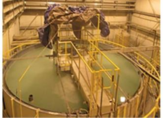
**4. Access provided by the catwalk** is in evidence here. The tarp is used to cover the clarifier during annual highpressure cleanings to capture fugitive dust and debris
