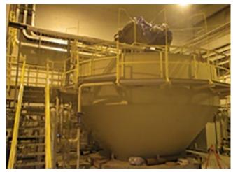
**3. Catwalk** is suspended from the clarifier with supports bolted to the weir frame and support legs free-floating and interlocked by the catwalk itself. This fastening arrangement was selected to avoid damaging the clarifier's 40-mil internal epoxy coating
