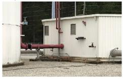
3. Jumper cable supplies a secondary source of power to the jockey pump when deployment in the event of a sudstation service is not available
