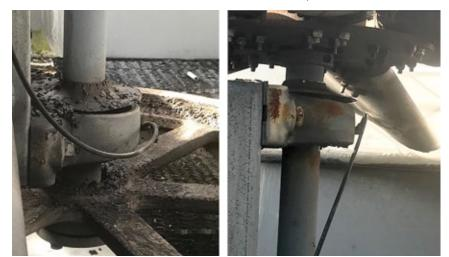
7. Grease is supplied to the bearings (lower at left, upper at right) via flexible hose
