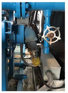
1. When the station-service transformer is out of service, power is supplied to the jockey pump from an alternative source via the welding receptacle
