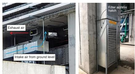
3, 4. Ductwork (left) conveys filtered air from the new intake location at grade (right) to the collector
