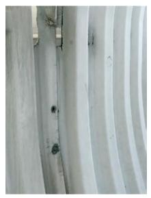
**1. Original stacks** were made of molded fiberglass, with sections bolted together on the inside
