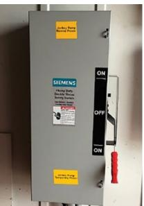
2. Selector switch transfers electric supply for the jockey pump from station service to an alternative source connected to the welding receptacle
