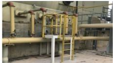
2. Staff-designed platform provides access to level switch without need for a ladder
