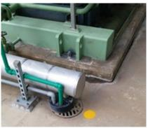
8. Drains have color circle to identify the sump to which is connected
