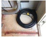
4. Jumper cable is ready for rapidden loss in station service power
