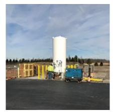
5. CO<sub>2</sub> bulk storage system holds enough gas for 10 generator purges
