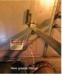
6. New fittings allow the operator to grease the fans and their motors without ever coming in contact with moving parts. No LOTTO required for normal PMs
