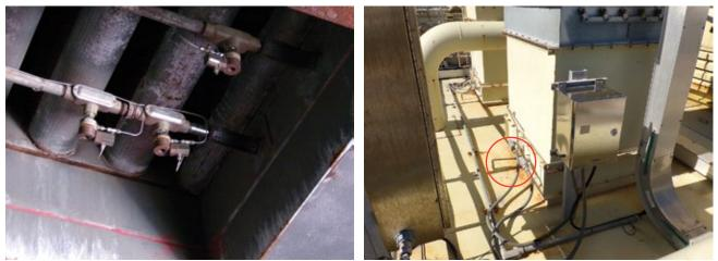
2. Haz-gas detectors (left photo) can be accessed from the compartment roof (circle in photo at right) where the analysis equipment is located
