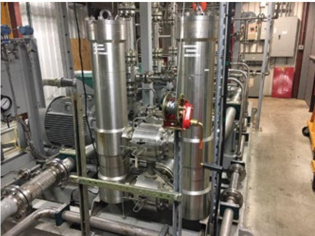
4. Winch, shown here installed on the plant's "east filter," can be moved to the west filter to remove that element when needed
