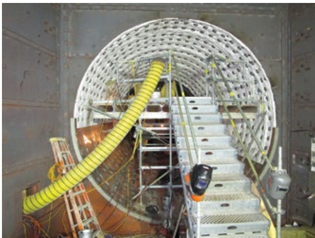
10. Innovative scaffold system accommodates simultaneous activities
