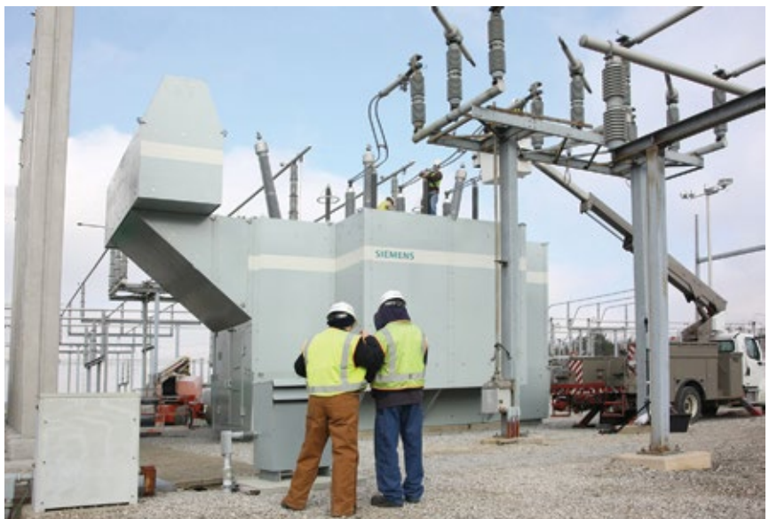
2. Panels comprising the protection system are removed for major maintenance
