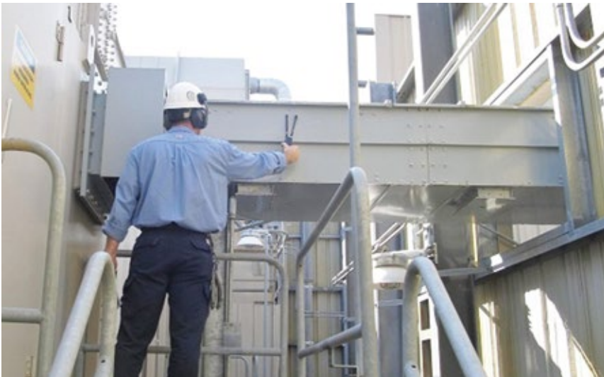
7. Generator is checked for radiated EMI above, bus below
