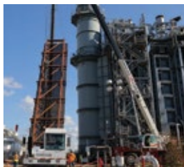
TEiC Installing HARP
