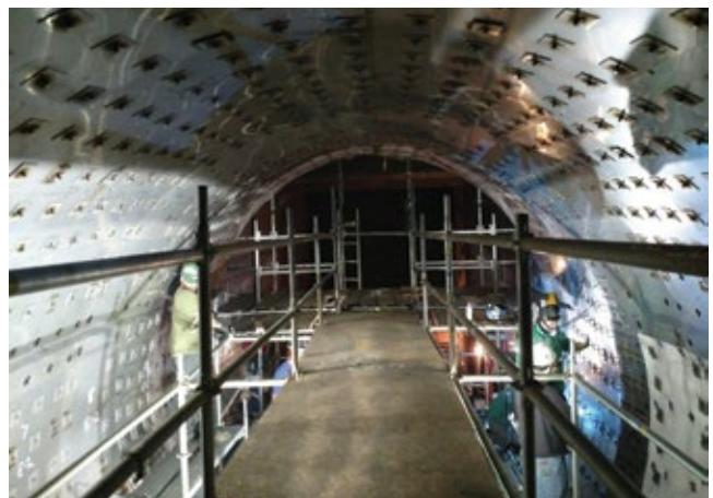
9. Scaffolding was installed on the new lower liners
