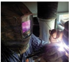
Installation of Replacement Metallic Casing Seal
