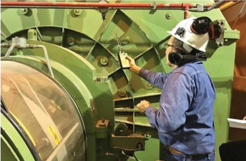
7. Generator is checked for radiated EMI above, bus below
