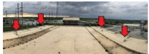
Fixed ladder (left), guardrails (center), and access-plate handles contributed to a safer workplace
