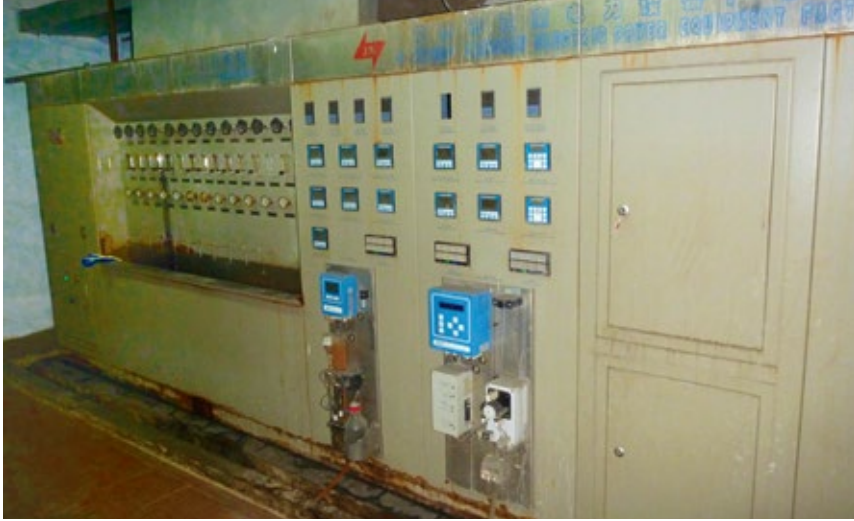
2. The entire sampling and analysis system at this plant had been out of service for eight years
