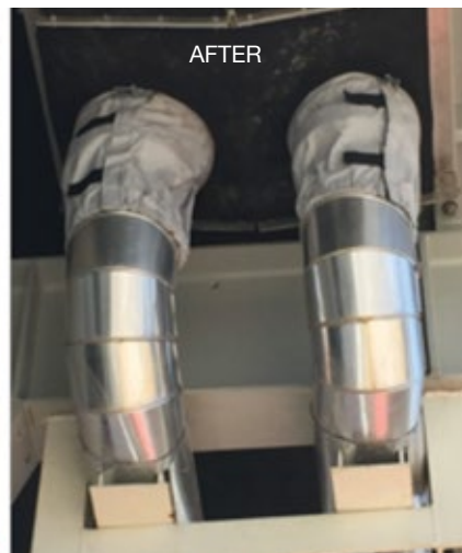
4. Penetrations for the chiller's cold-water coils , as installed (left), allowed leakage of unfiltered air into the filter house. Expansion-joint-type covers were installed to protect against this (right)
