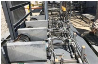
Legacy fog system skid with ceramic-plunger pumps is at left, upgrade to water-lubricated Danfoss pumps is at right
