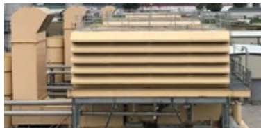
Fixed ladder (left), guardrails (center), and access-plate handles contributed to a safer workplace
