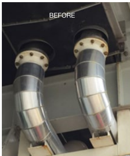
4. Penetrations for the chiller's cold-water coils , as installed (left), allowed leakage of unfiltered air into the filter house. Expansion-joint-type covers were installed to protect against this (right)
