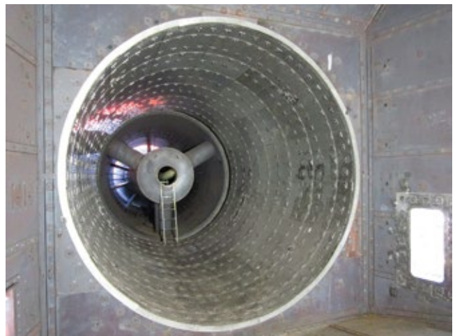
11. Completed upgrade of 7FA diffuser duct
