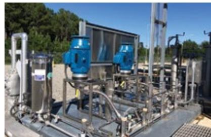
Legacy fog system skid with ceramic-plunger pumps is at left, upgrade to water-lubricated Danfoss pumps is at right
