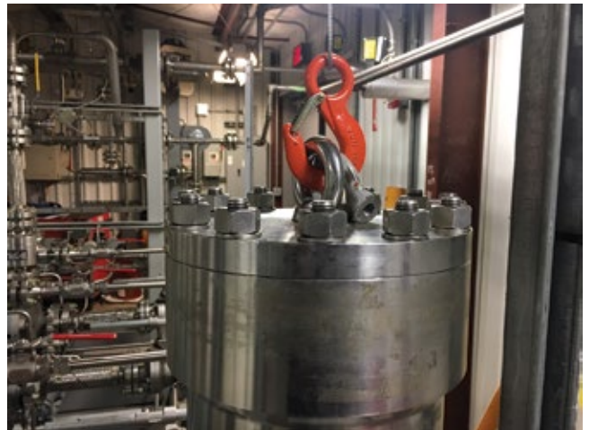
4. Winch, shown here installed on the plant's "east filter," can be moved to the west filter to remove that element when needed
