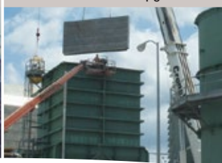
Exhaust Silencer Upgrades
