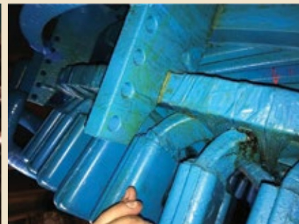
1, 2. Inspections in the early 2000s found problems primarily on the stators—such as connection-ring vibration (left) and stator bar vibration (right)
