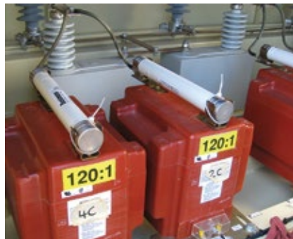
1-3. PT fuses migrating out of their clips (left), holding fuses in place with zip ties was not successful (center), new style of fuse clip at right eliminated fuse migration
