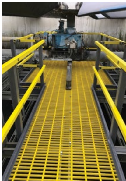
7. Permanent work platforms, made of FRP, have a net free opening of 83%. Photo left is looking in at fan, looking out at right
