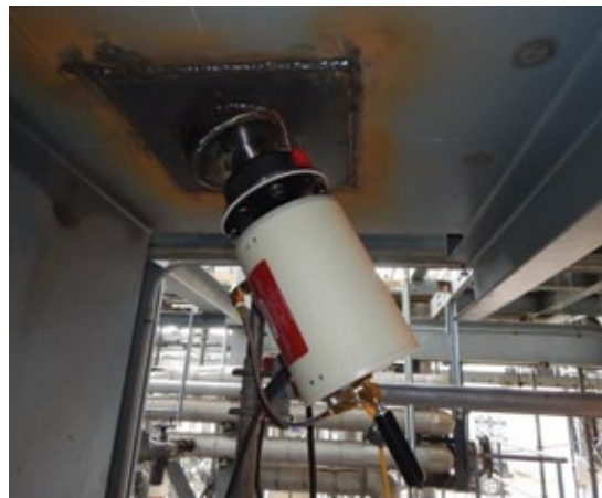
2. Camera was retrofitted to help identify early signs of duct-burner trouble
