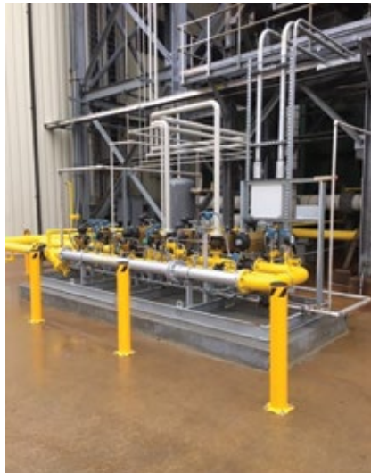
2, 3. Fuel-gas skid and distribution manifold for the duct burners are at left, burner platforms at multiple elevations at right
