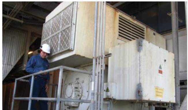
2870-hp motor, 13.8 kV, 100 amps
