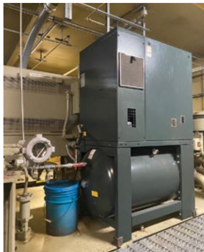
4. AirCenter replacement air compressors had more than three times the capacity of the original equipment
