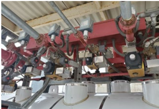
7. In-line odorizers are installed in high-exposure areas
