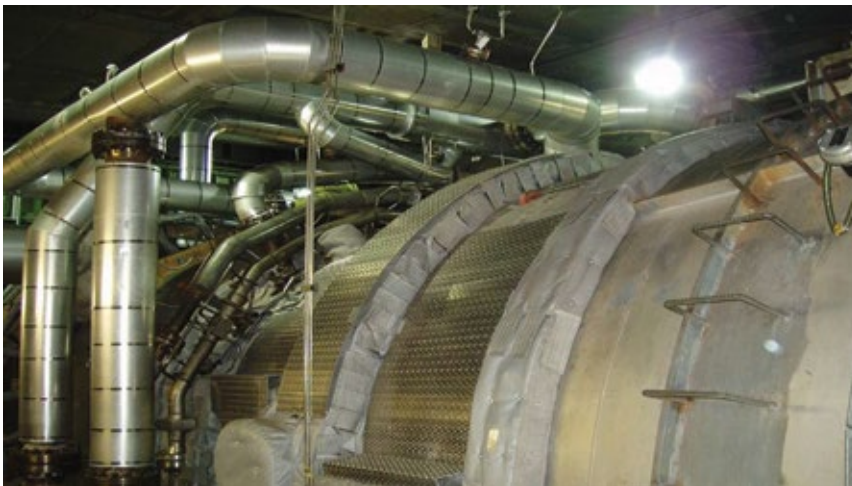
2. Step protection is a clearly visible component in the GT24/26 single-layer insulation system
