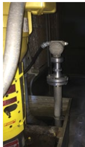
5, 6. Evap-cooler basin as seen from the outside with solenoid valves installed (left); basin level transmitter is at right
