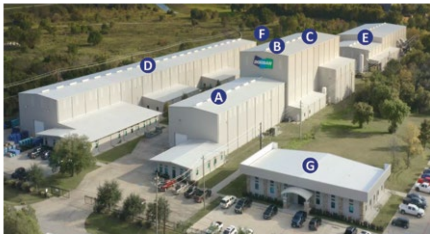
1, Doosan Turbomachinery Services has more than 100,000 ft 2 of shop operations under roof at its La Porte facility, with room for expansion. Rotor bay A in the photo has dual 30-ton cranes, rotor high bays No. 1 (B) and No. 2 (C) each have 100-ton and dual 30-ton hooks, component repair shop (D) has 30-, 10-, and dual 5-ton cranes, thermal spray coating area (E) is equipped with dual 30-ton cranes. Building F is the blast/surface modification facility and G is the admin building
