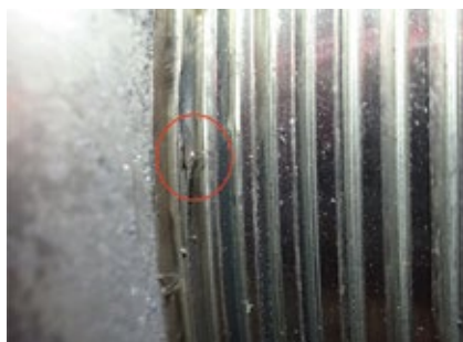
15. J-seal installation tip: Butt-gap overlap at left is not acceptable; gap overlap of 0.010 to 0.020 in. at right is acceptable
