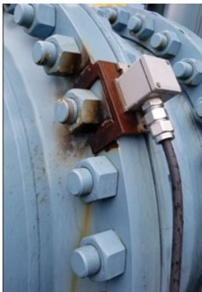
3. Radio-frequency device installed on circulating-water pipe disrupts the lifecycle of algae shortly after their creation
