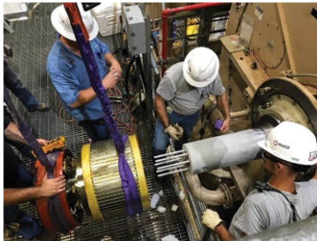
4. New exciter field is installed
