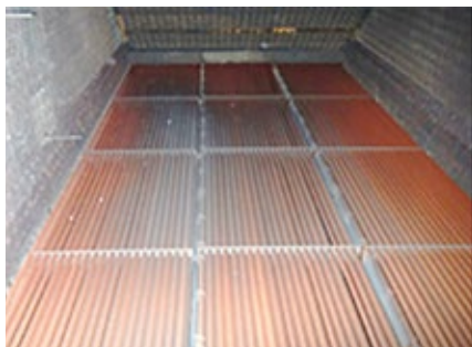
9. Identical HRSGs , mirror images of each other, show overheating at the higher elevations and biased toward the fuel inlet to the duct burners (left side at left, right side at right)
