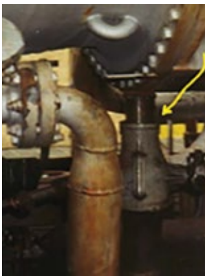
9-4. Temporary mechanical jack is shown in place
