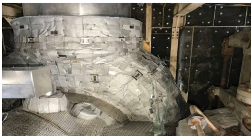
1. ARNOLD advanced single-layer turbine warming system
