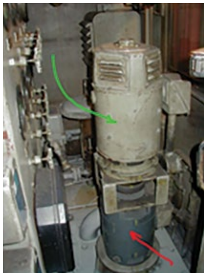
13-1. Emergency lube-oil pump , located inside the oil tank, has both dc (green arrow) and ac (red arrow) motor drives arranged in piggyback fashion
