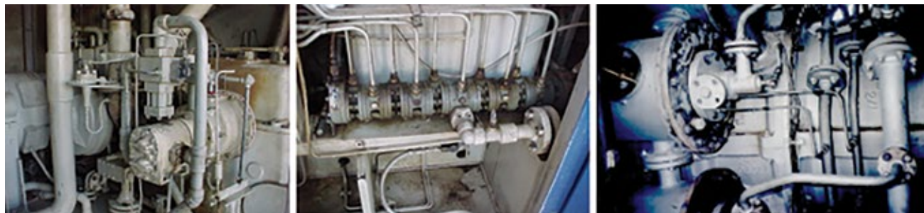
11-2. Operation of the fuel pump (left), flow divider (center), and combustion chamber (right) can be adversely impacted by cold weather, making heaters necessary
