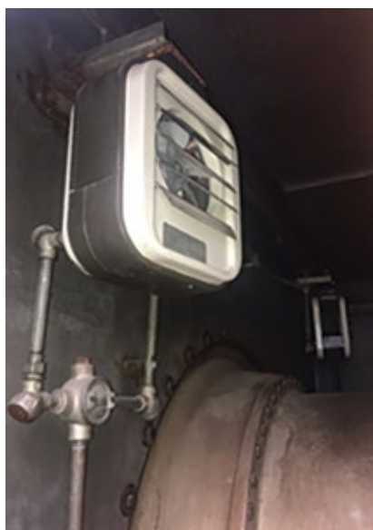
11-1. Space heaters are installed in the accessory and turbine compartments to promote reliable operation of critical fuel-system components
