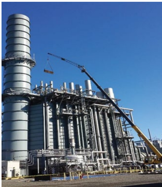
6. Groome replaced the ammonia injection grid and SCR catalyst in this HRSG
