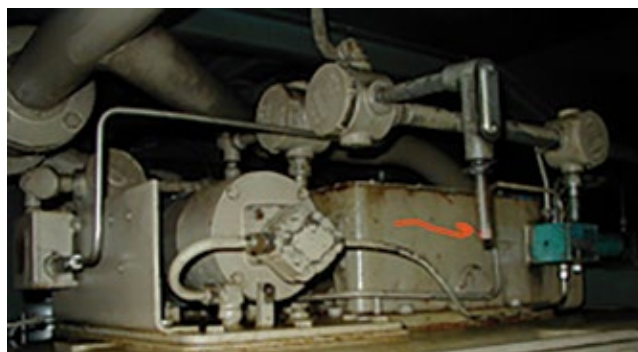
10-2. Temperature sensor for CO 2 system activation is in accessory compartment here (right)
