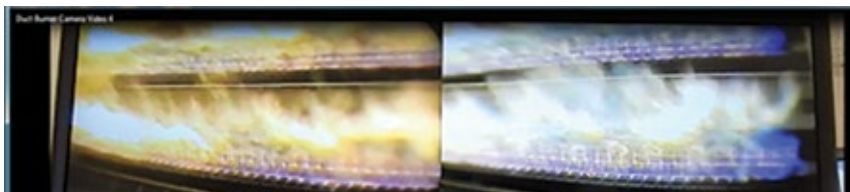
11. Duct-burner flame length can be monitored using a camera and control-room display
