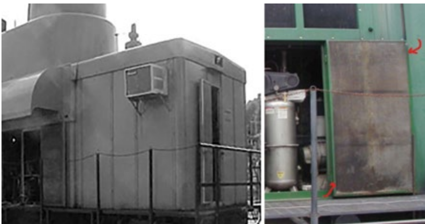
10-4. Seals for package panels and doors (left) must be maintained in good condition to prevent leakage of CO 2 . Seals at right should be replaced
