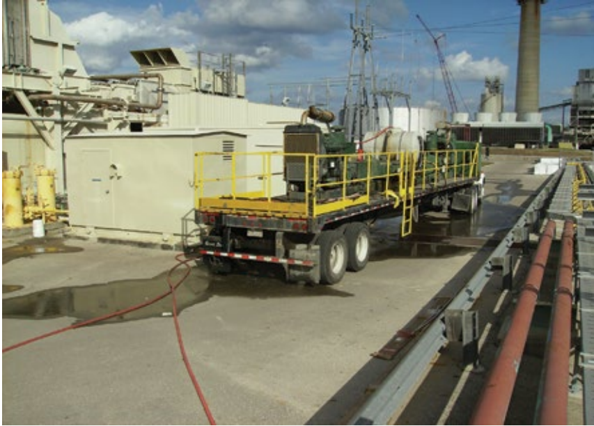
2. Hydrolazing liquid-fuel lines to remove coke is no small task; flatbed holds all the equipment required
