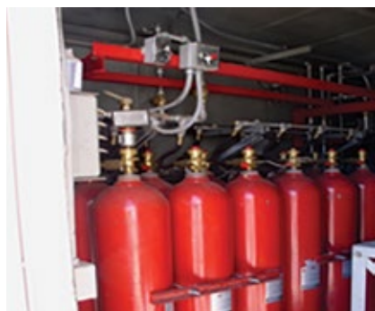
10-1. Cardox fire-protection system was used in GE’s early package power plants (left)
