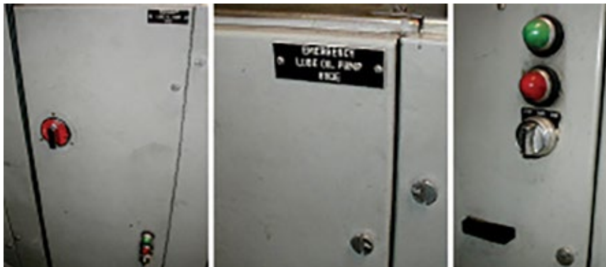
13-2. Motor starter (dc) inside the motor control center shows details of the panel, nametag, sequence lights, and test switch
