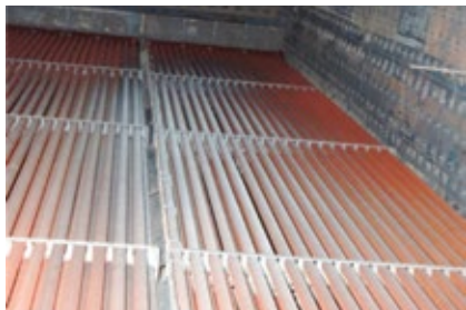
12. Gray zones in tubes downstream of the duct burner often correspond to long flames and possible overheating
