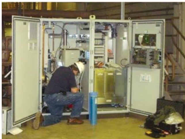
1. Nel Hydrogen's onsite hydrogen production system requires little space to serve a 500-MW plant
