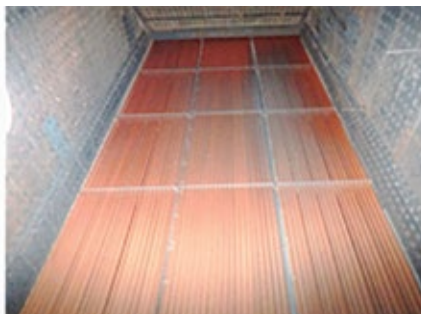
9. Identical HRSGs , mirror images of each other, show overheating at the higher elevations and biased toward the fuel inlet to the duct burners (left side at left, right side at right)
