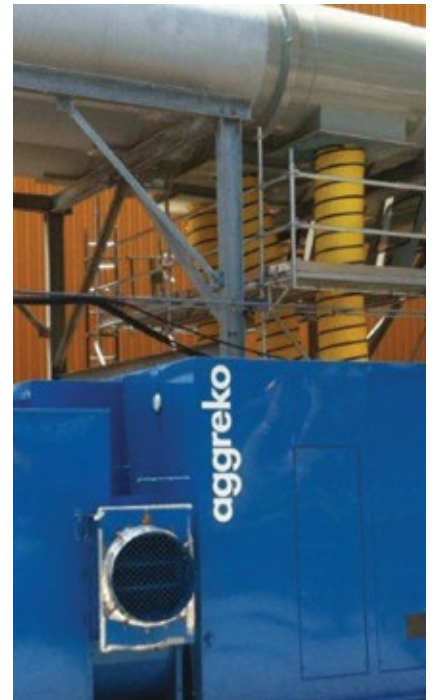
4. Electrical Builders' forced-air system cools busduct conductors and controls condensation
