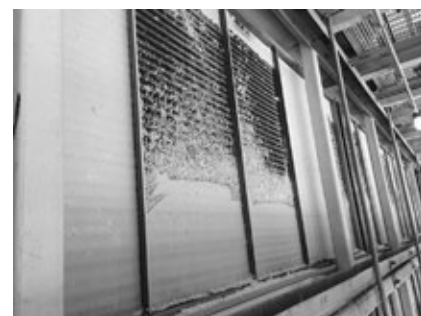
2. Ice buildup on the upstream face of the glycol heating coils impedes air flow
