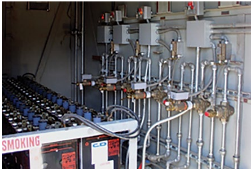
10-3. Modified CO 2 system was moved to an external building
