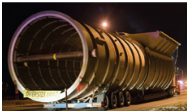
10. Stacks were trucked to the site in two pieces
