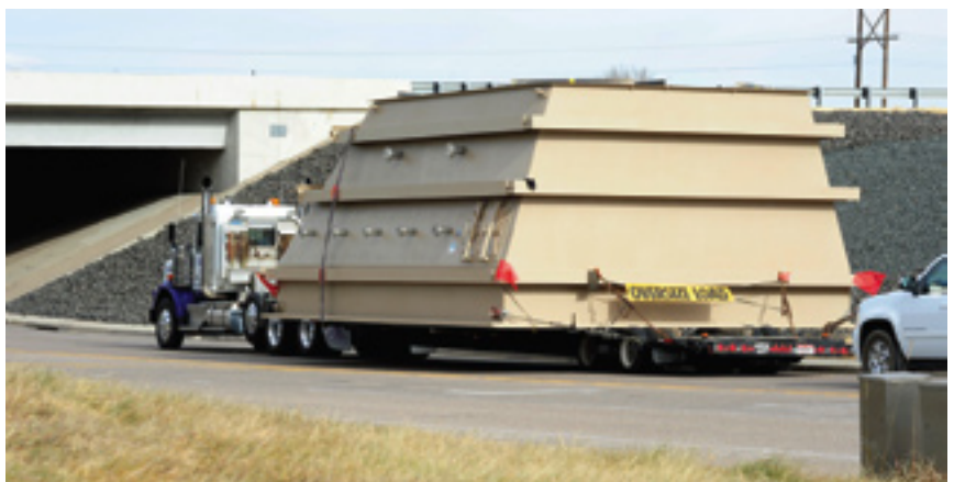
9. Very large subassemblies were prefabricated and shipped to Pueblo
