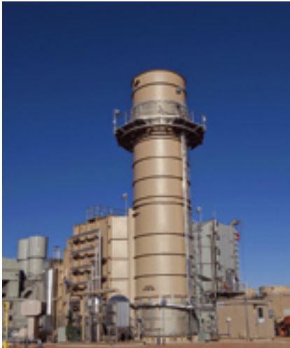
5, 6. Exhaust section for Pueblo LMS100 features redundant equipment (PLC connections to the plant DCS, tempering-air fans, ammonia vaporizers) to maintain NO x and CO emissions within permit limits
