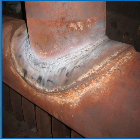
Problematic design features hindering inspection
