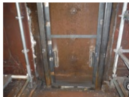
4. New sidewall structure with vertical slide affixed to the casing provides the necessary rigidity for catalyst module support and sealing
