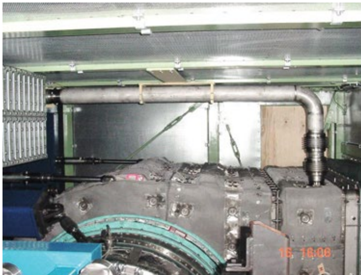
ARNOLD Group insulation systems for LM2500 and LM6000 engines are designed for a perfect fit to the gas turbine thereby maximizing the lifetime of the thermal shield
