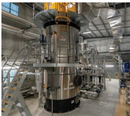
8. A 13-MW electrode boiler serves New Zealand's Open Country Dairy
