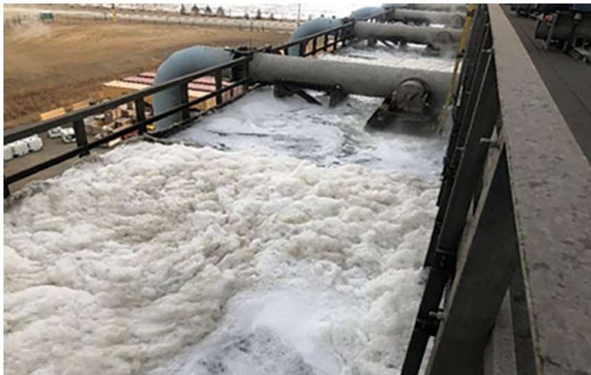
4. High levels of total dissolved solids and organic material cause foaming in the cooling tower
