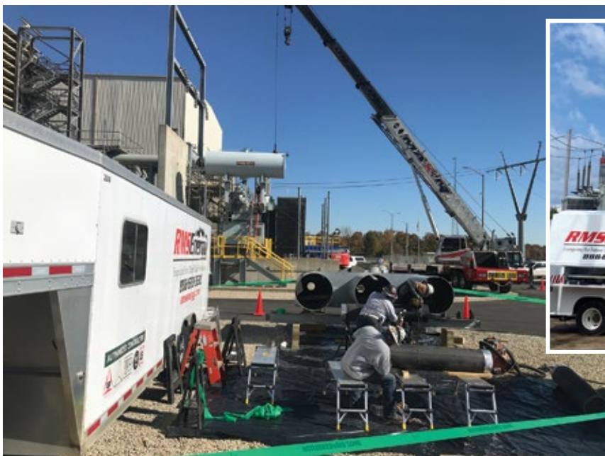
Proper assembly (left) and installation (right) of bus duct are necessary to prevent moisture ingress
