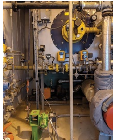
2. New controller (above) is located in front of the boiler (right)
