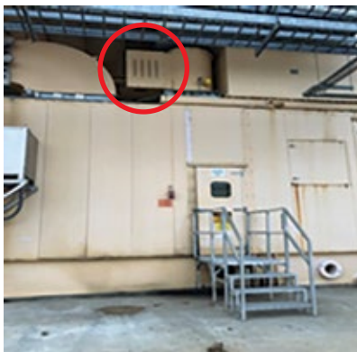
2. The need for a platform to access generator fans is in evidence here. Photo at left was taken before platform installation, at right after
