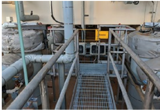
4. New platform facilitates the safe removal of condensate strainers
