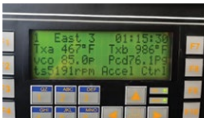
1. Data displayed when operating at full speed/no load (FSNL) are the following: Turbine speed, 5191 rpm; turbine exhaust temperature (average of all working exhaust thermocouples), 467F; compressor discharge pressure, 76.1 psig; fuel-pump stroke, 85 psig
