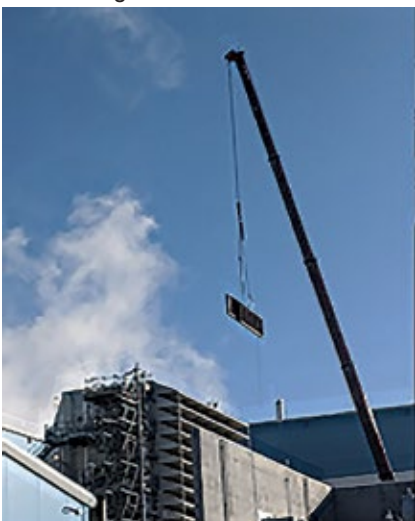
2. New coils are lifted into position
