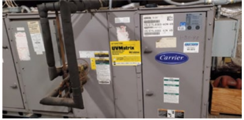
3. UV-light ultrafiltration system improved air quality in the admin building and control room
