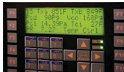
2. Data displayed after the engine is synchronized to the grid (so-called base temperature control) are the following: Turbine speed, 5191 rpm; turbine exhaust temperature (average of all working exhaust thermocouples), 851F; compressor discharge pressure, 90.0 psig; fuel-pump stroke, 168 psig
