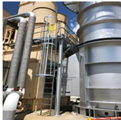
1. Turbine package fans before (left) and after (right) installation of platform to facilitate access and make the work location safer
