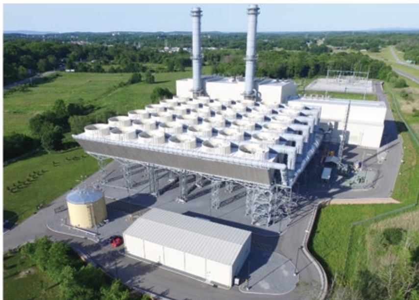
3. In-Air induced-draft ACC was the first such unit installed in the US
