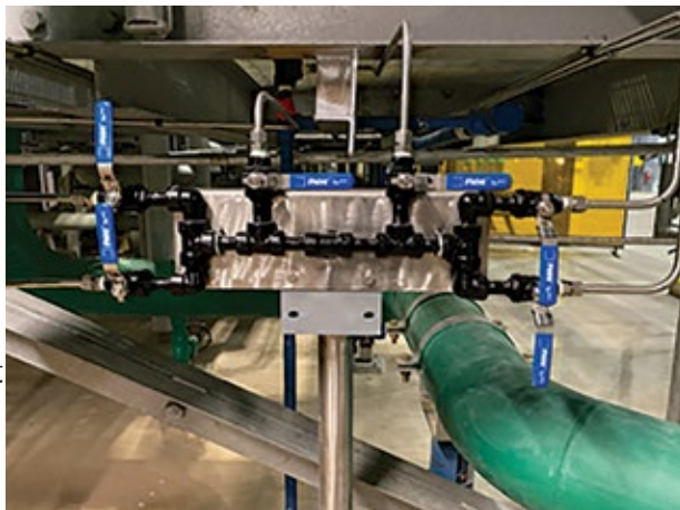
4. Manifold station for filling “U” seals simplifies what had been a time-consuming job with safety risks
