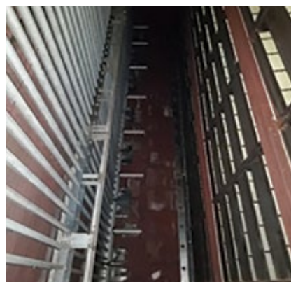
3. New AIG with center support and inside header shown here enabled Milford Power to meet its new operating-permit limits
