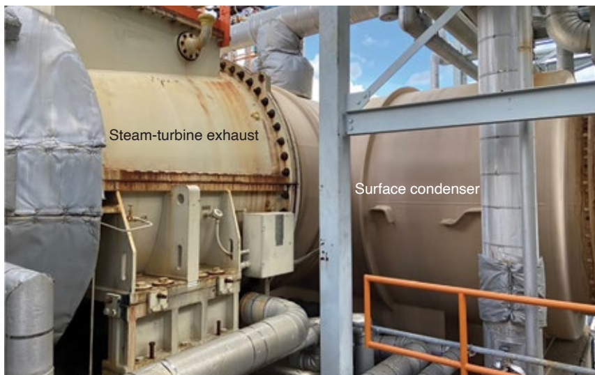
1. Arrangement of surface condenser and steam-turbine exhaust
