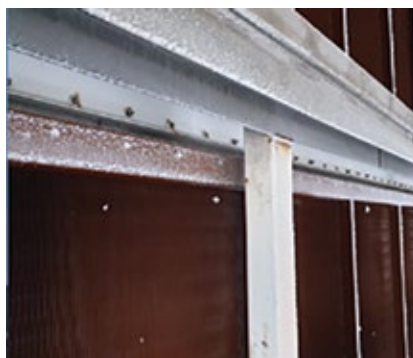
3. Ice be gone with new coils in place
