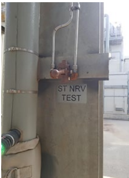
2. New location for NRV test valve
