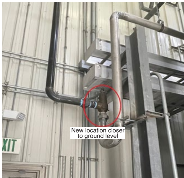
1, 2. Safety/relief valve, located in a congested area (left), was moved closer to ground level to facilitate inspection (right)
