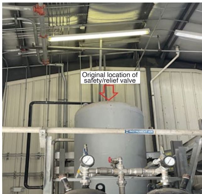
1, 2. Safety/relief valve, located in a congested area (left), was moved closer to ground level to facilitate inspection (right)
