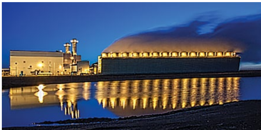
6. Shepard's cooling tower now operates at 5.2 cycles of concentration, up from 3.2
