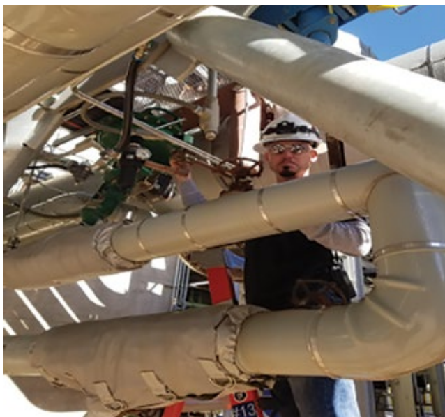
1. Test valve as originally installed (left), note that the operator's position to perform the test does not allow for safe viewing of the actuator (right)
