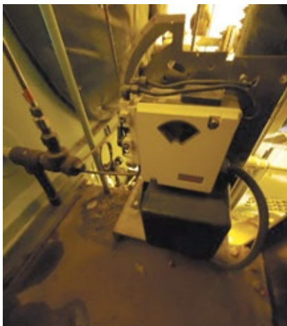
1. Original controller was located on top of the boiler, by the steam drum
