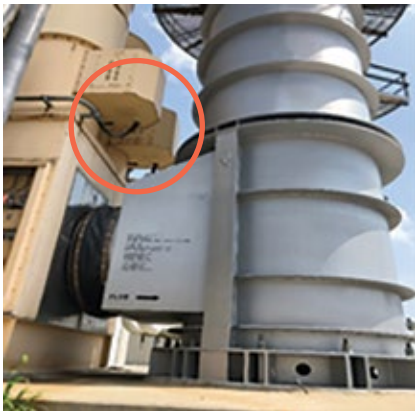
1. Turbine package fans before (left) and after (right) installation of platform to facilitate access and make the work location safer
