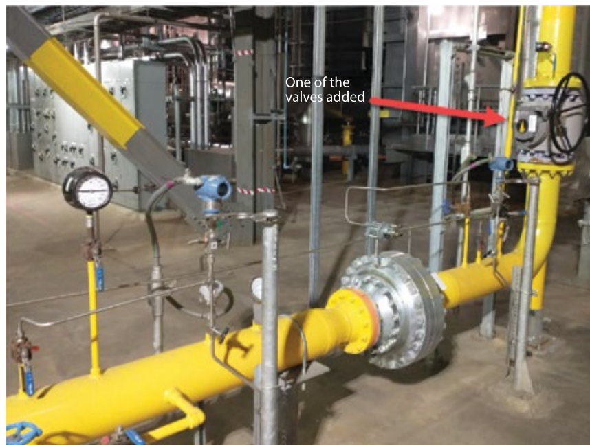
1. One of the new isolation valves added for each generating unit
