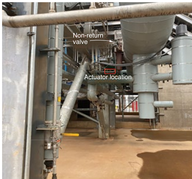
1. Test valve as originally installed (left), note that the operator's position to perform the test does not allow for safe viewing of the actuator (right)
