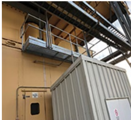
2. The need for a platform to access generator fans is in evidence here. Photo at left was taken before platform installation, at right after
