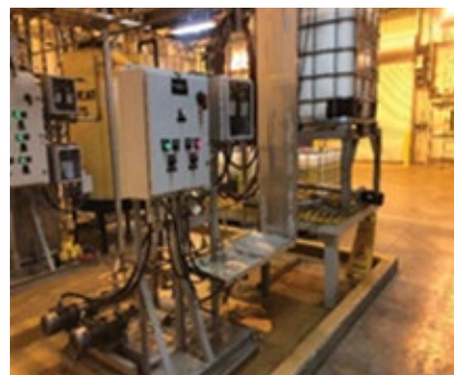
5. Anti-foam pump skid has dealt successfully with Shepard's cooling-tower foaming issue
