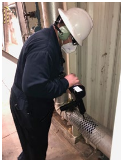
1. Technician checks steam trap for proper operation at left, views results above
