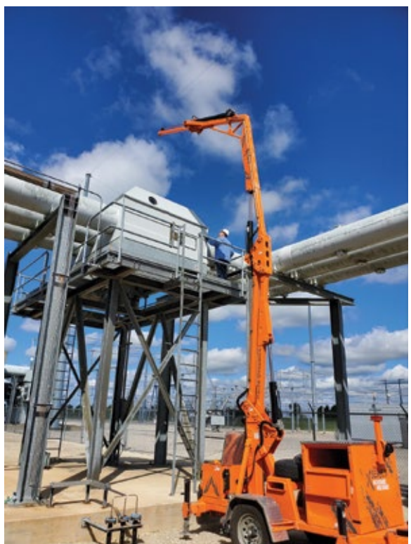
3, 4. Mobile tie-off system in travel mode at left, ready for work at right.
