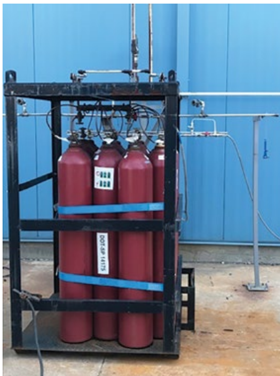
1. Hydrogen for Marcus Hook's generators is delivered in 16-cylinder cradles
