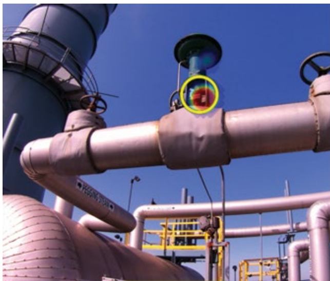
2. Pegging-steam leaking from control valve
