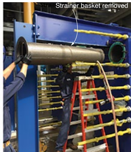
5. Removal of the strainer basket for the plate-and-frame heat exchanger was a difficult task before modifications were made
