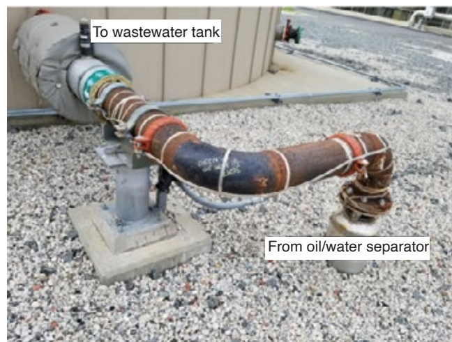
1. Original piping between the oil/water separator and the wastewater tank is at left, new arrangement with the three-way valve is at right
