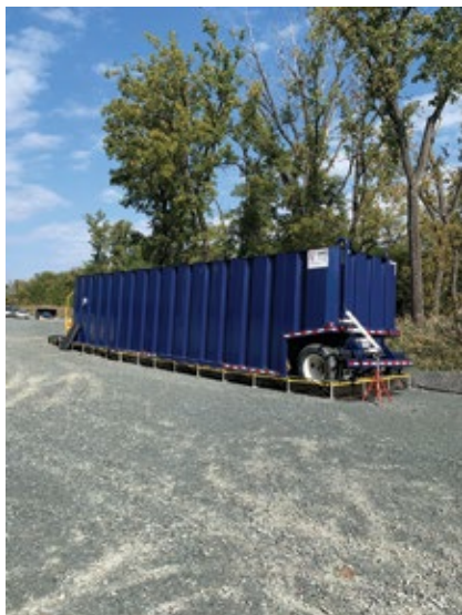
3. Sump pumps transfer water, recovered as geotubes drain to the frack tank above, to the cooling tower
