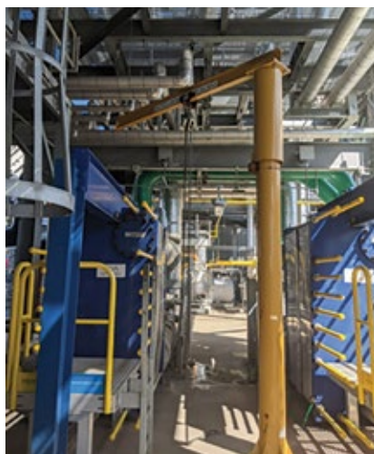
6. Jib crane, installed between both heat exchangers, facilitated removal of the blank flanges to access the strainer baskets
