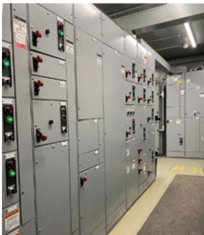
5. MCC indicator lights and sockets in the PEECCs were replaced with much brighter, relampable LED fixtures. No mods to wiring or bucket mounting were required
