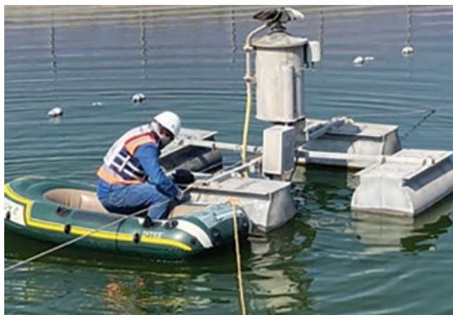
2. Mechanical evaporator is set in final position
