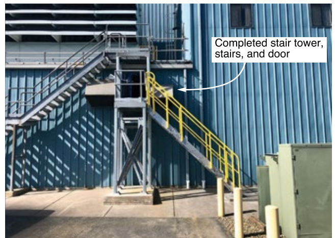
10. New staircase provides access to the intake fans via a doorway cut in the building wall
