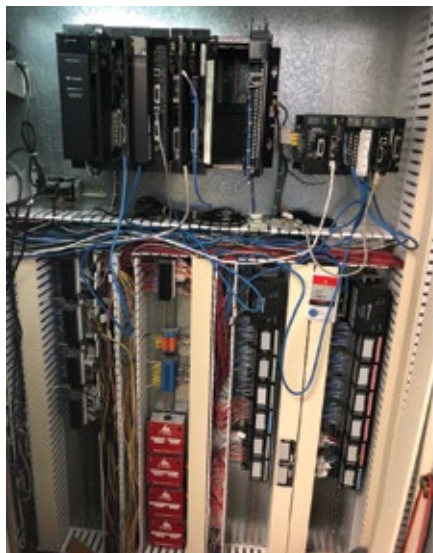
1. Original BOP PLC (left) was obsolete and replaced with GE's fully redundant RX3i PLC at right
