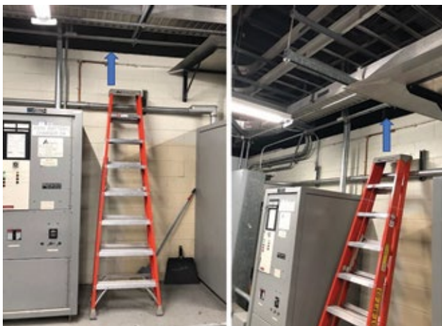
9. The plant, as designed, required a ladder to access the MCC intake fan and filter units
