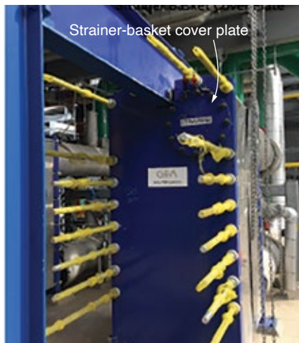
5. Removal of the strainer basket for the plate-and-frame heat exchanger was a difficult task before modifications were made
