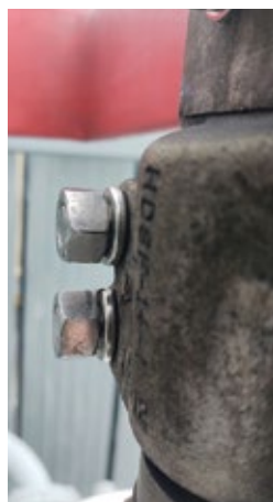
8. Loose neutral bushing in the GSU for the STG (left)
