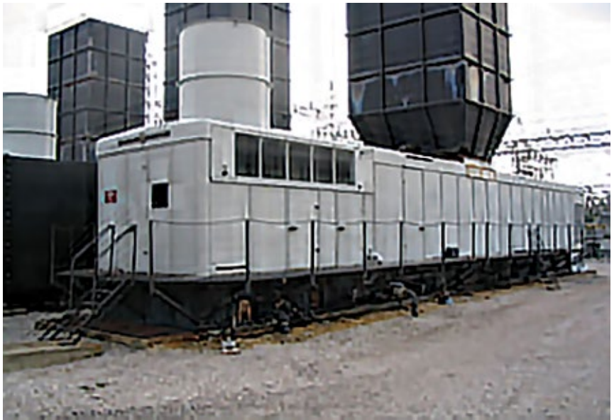
3. Package Power Plant powered by an MS5001L engine at a utility generating station dates back to 19688
