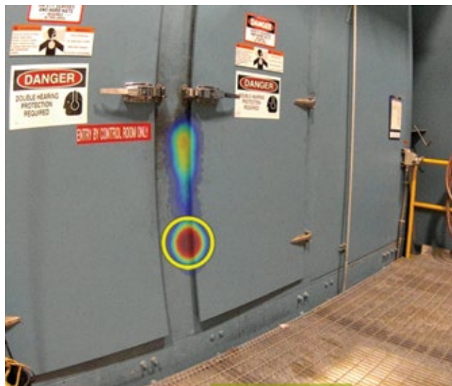
3. Damaged gasket allows air leakage at package door
