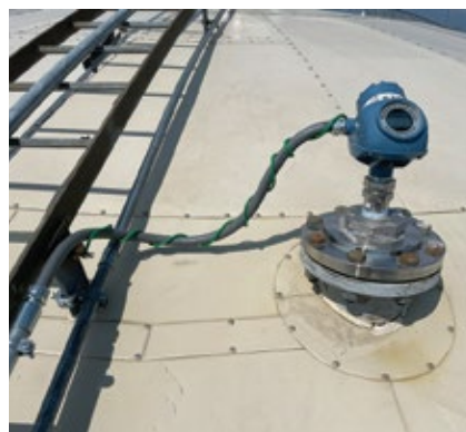
1. Guided-wave radar transmitters are located at the tops of the tanks
