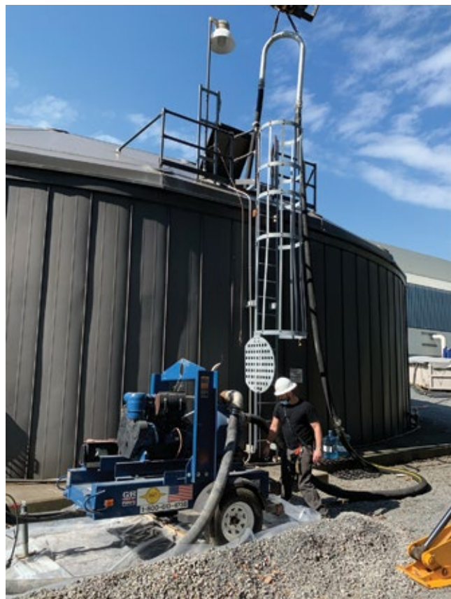
1, 2. Semi-solid waste material is pumped from the chlorine contact chamber (left) to geotubes (right) by an engine-driven pump
