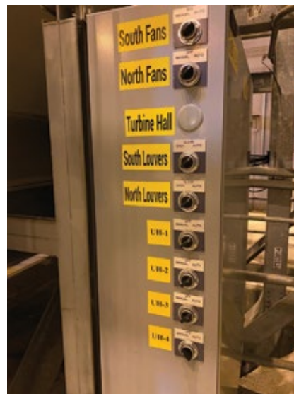
2. DCS operator screen (left) and local control panel (right) facilitate control of turbine-hall HVAC equipment
