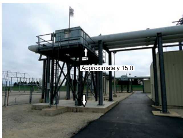
1, 2. Personnel have adequate fall protection when generator breaker work can be performed from platforms designed into the plant
