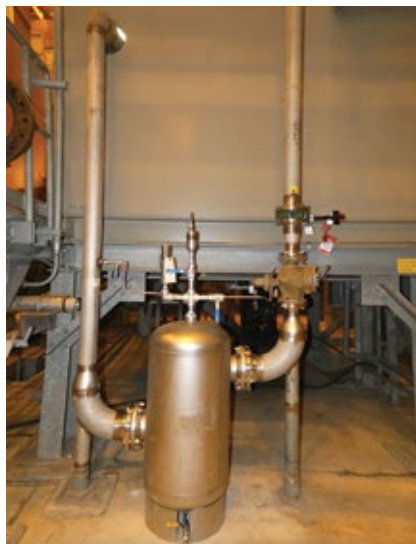
3. Vortex air separator is located in the demineralized-water forwarding piping at the inlet to each water-injection skid
