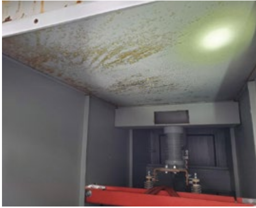
3. Condensation is in evidence in PT cabinets
