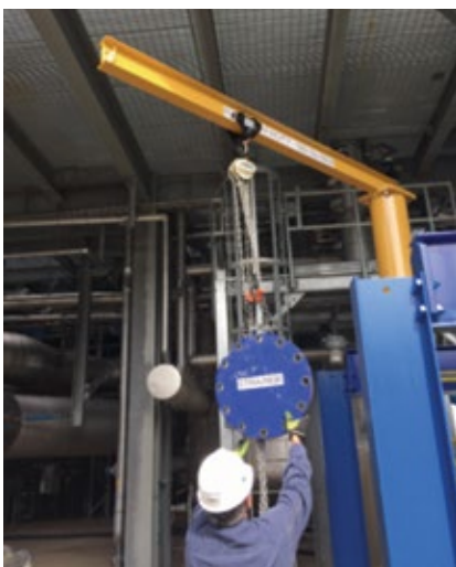
7. Blank flange is lowered to floor level using the jib crane
