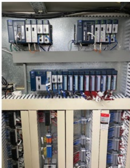
1. Original BOP PLC (left) was obsolete and replaced with GE's fully redundant RX3i PLC at right
