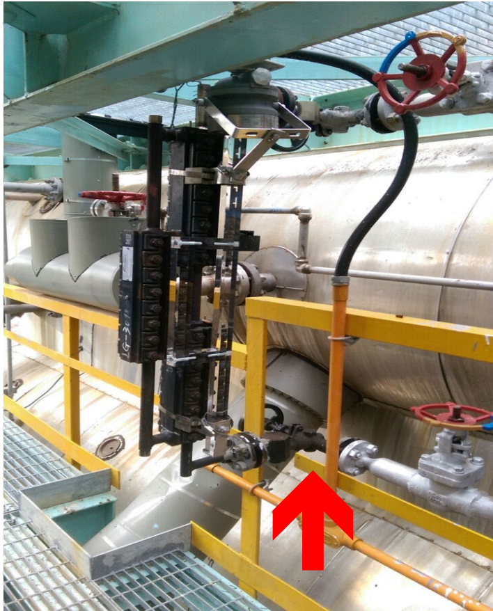
A drain valve is missing on this lower water gage valve
