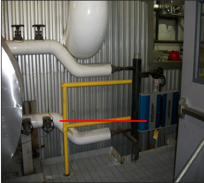
Installation error with gage elevation
