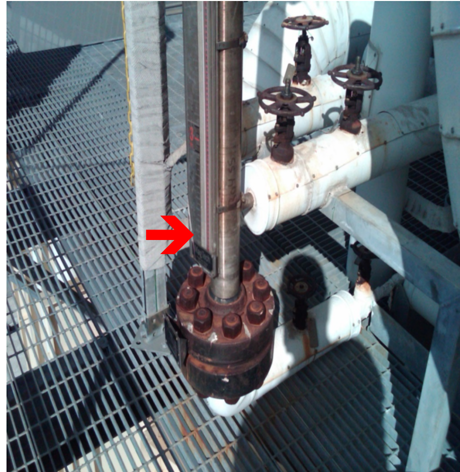
The scale on this magnetic level gage extends below lower connection, it will always indicate some level.
