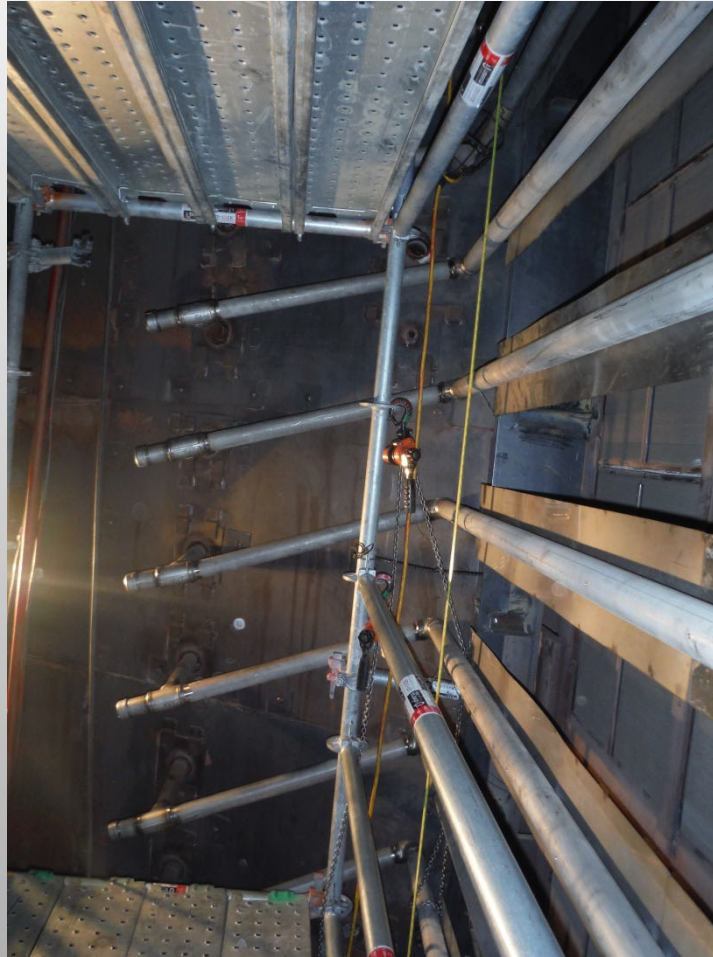
New SS AIG Pipes With Mixing Baffles Attached
