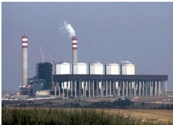
5, 6. The ACC at Kusile Power Station in South Africa (above) and view of fans from below (right)
