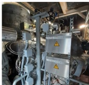
4. Single-layer insulation and step-protection system from Arnold is installed at left. All electrical connections, center and right, are moved away from the casing
