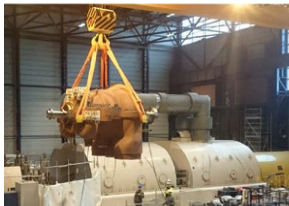
4. Single-layer insulation and step-protection system from Arnold is installed at left. All electrical connections, center and right, are moved away from the casing
