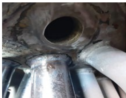
7. P91 stubs were replaced with ones of increased wall thickness
