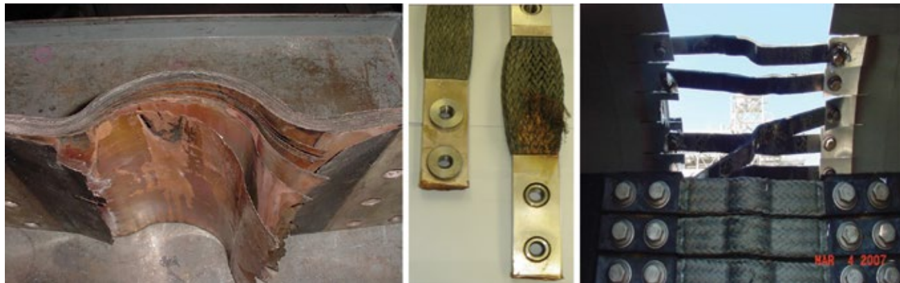
4. Some things to look for when troubleshooting bus duct: Cracked laminations caused by vibration or air flow (left), damaged flex braids caused by rubbing and/or abuse (center), and damage attributed to improper bolting and/or lack of maintenance at connection points (right)
