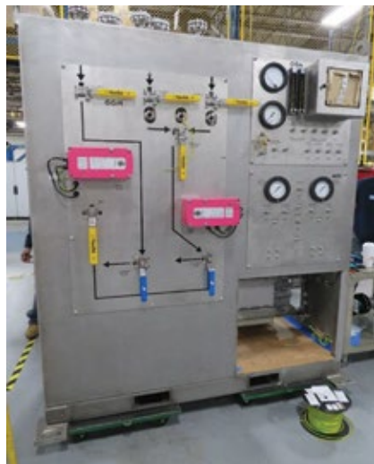
1. Automated gas manifold/ hydrogen monitoring system is recommended for plants wanting to reduce the time required to come back from an outage
