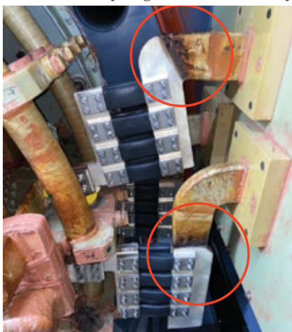
8. High-voltage connection inspections by qualified personnel allow rapid identification of overheating issues
