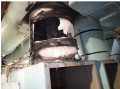
5. Damage resulting from an isophase-bus fault included the bushing-to-PT compartment failure at left and neutral and line enclosure damage at right
