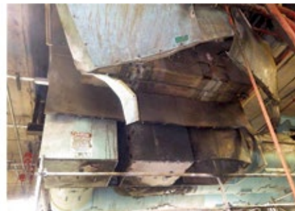
5. Damage resulting from an isophase-bus fault included the bushing-to-PT compartment failure at left and neutral and line enclosure damage at right
