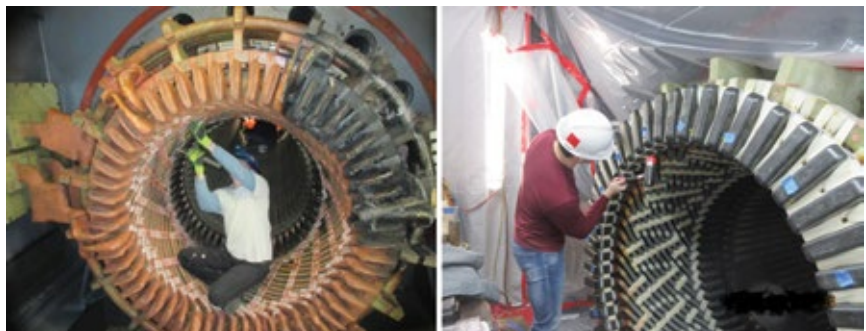
12. Repairs are made in photo at left to correct a stator failure (T6 neutral phase ring at flex leads). Rewind complete, the phase ring is prepared for bump testing at right
