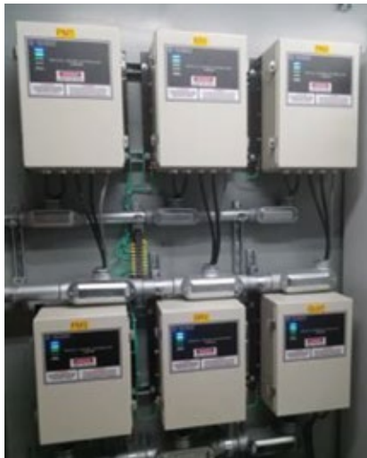
3. Digital motor controllers are powered by 120-Vdc batteries, have IP65-rated enclosures, accept 24- or 125-Vdc trip signals, and come with hazardous environment certification
