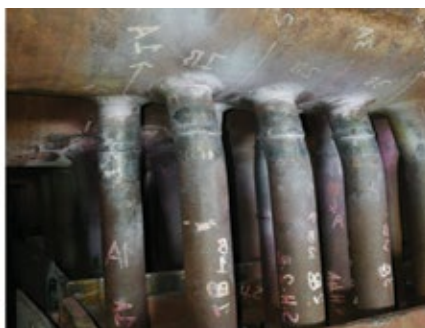
7. P91 stubs were replaced with ones of increased wall thickness
