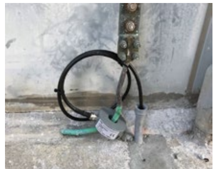
5. RFCT installed on the frame ground; usually coupled around the generator to the neutral ground connection
