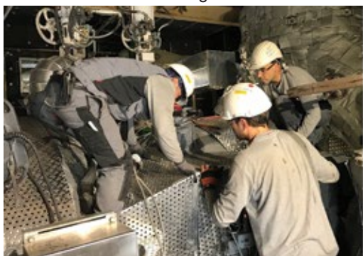
4. Single-layer insulation and step-protection system from Arnold is installed at left. All electrical connections, center and right, are moved away from the casing
