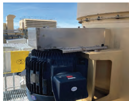
2. Pulley/belt guards benefit safety, improve reliability
