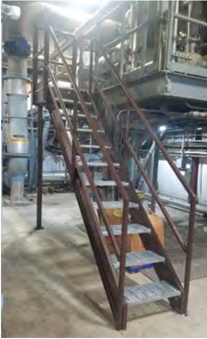
4. Stairs replaced ladder
