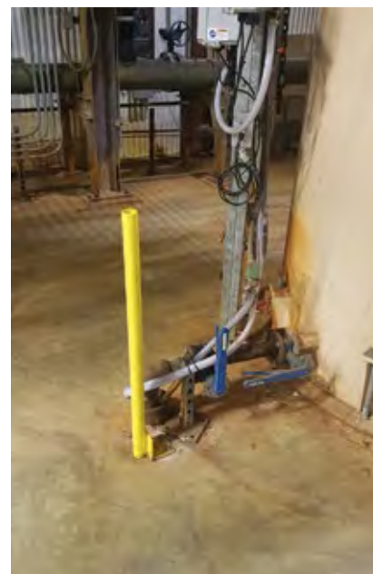
3. Posts help prevent people from walking into protruding objects
