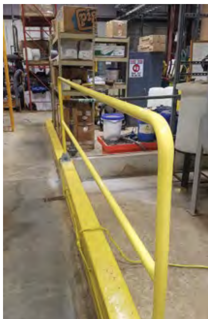
1. Guardrail protects against curb trip hazard
