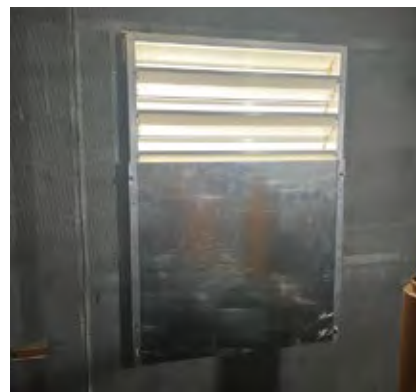
1. Natural ventilation to atmosphere is provided via stationary louvers
