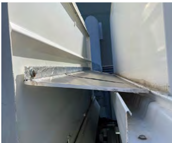
1. A plexiglass panel was installed on the breaker to protect against inclement weather
