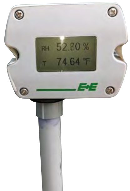
2. Sensor monitors both space temperature and humidity
