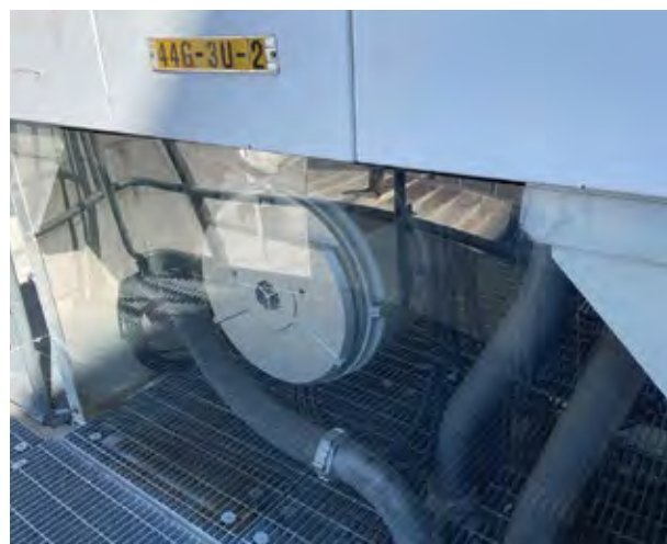
1. A plexiglass panel was installed on the breaker to protect against inclement weather
