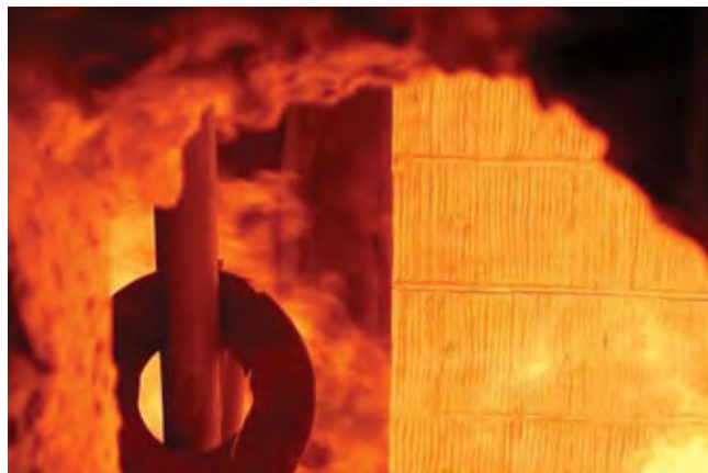
HRST Inc. With the duct burner at maximum firing, use view ports to visually observe the flames for length and shape. Important to avoid flame impingement
