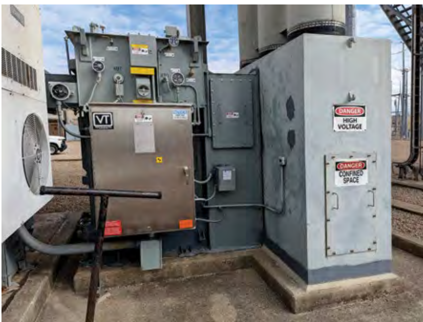
1. Excitation transformer is tied to the isophase bus through a dry bay shroud, where the flashover occurred
