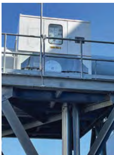
1. A plexiglass panel was installed on the breaker to protect against inclement weather
