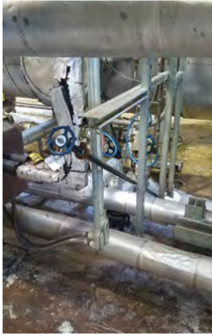
5. Valve operator extension eliminates crawling under piping
