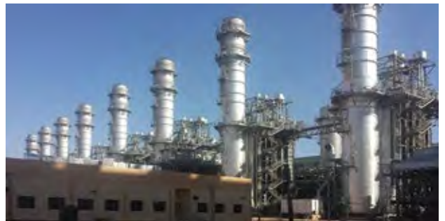
Faras is a 1610-MW facility with 17 gas turbines rated from 75 to 140 MW
