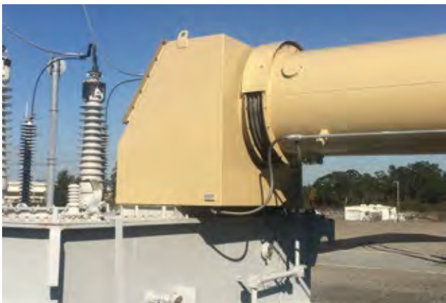
3. Updated circular isophase bus-duct support systems typically have fewer footers/columns and hangars than the traditional rectangular design
