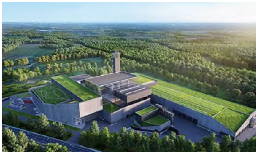
1. Poland's largest waste-to-energy plant in Warsaw features minimal visual impact and low-noise operation
