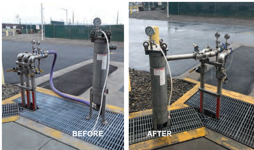
2. Permanent piping replaced flexible hose and original connections
