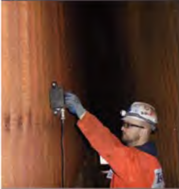
Through Fin Tube Scanning for Wall Thinning
