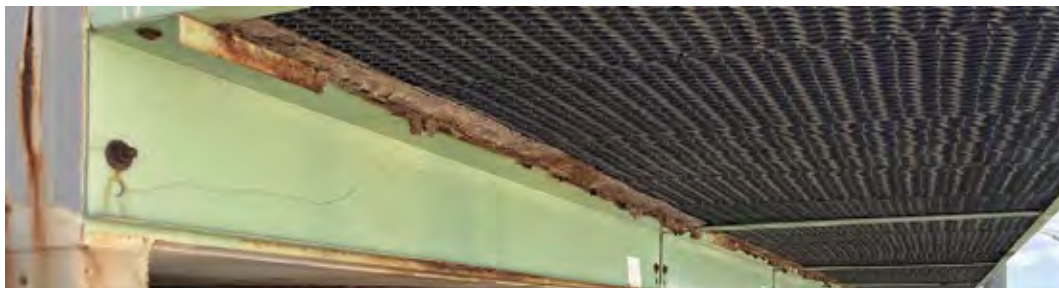
3. Moisture separator and other components for the inlet filter house, should not be neglected as gas-turbine plants approach the end of their design lives. Z bars, spacer, and hardware rust over time and begin to come apart
