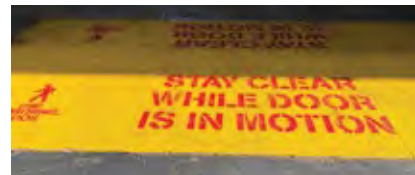
6. Conspicuous floor markings remind plant personnel and visitors to stay clear while the door is in motion
