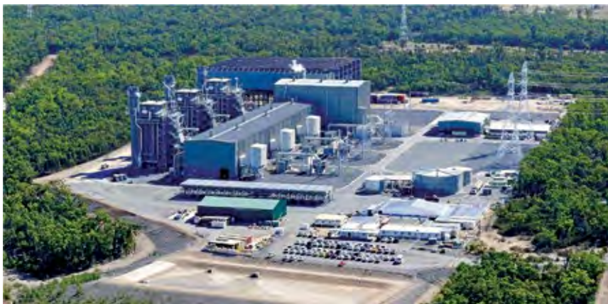
1. Darling Downs Power Station, a 630-MW, 3 × 1 coal-seam-gas-fired combined cycle, is powered by three Frame 9E gas turbines
