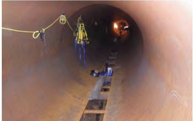
C. Largest main duct diameter is 23 ft (left)
