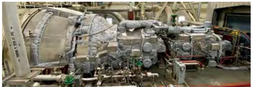
4. Siemens steam turbine is fully equipped with electrical-based warming system and advanced insulation to dramatically reduce combined-cycle startup time
