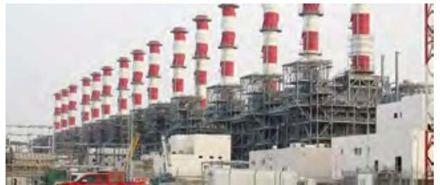
Qurayyah , started as an open-cycle powerplant and converted to fifteen 3 × 1 combined cycles
