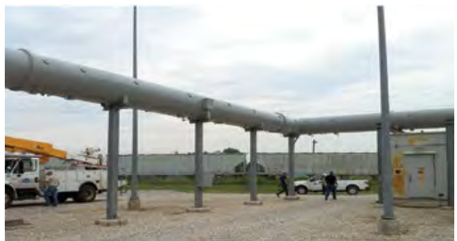
3. Updated circular isophase bus-duct support systems typically have fewer footers/columns and hangars than the traditional rectangular design
