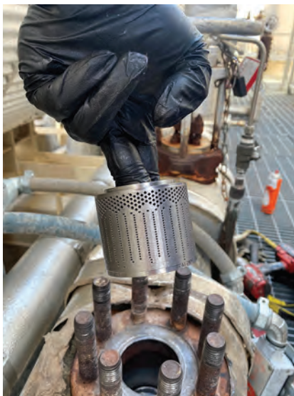
2. New trim is inserted into the existing valve body
