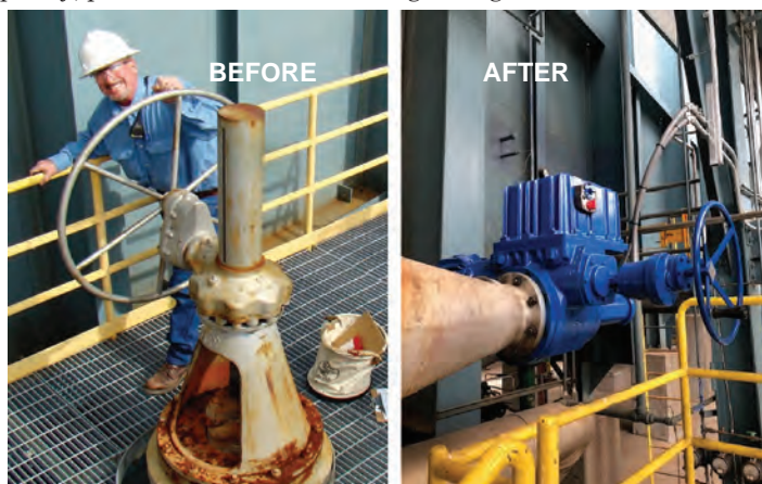
3. Valve operators were upgraded from manual (left) to motor-operated
