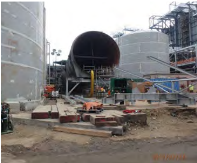
C. Largest main duct diameter is 23 ft (left)
