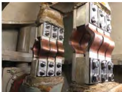
5. Flex links are being stocked by several vendors; universal size at left can be machined to fit different models and configurations, then holes are drilled for installation (right)
