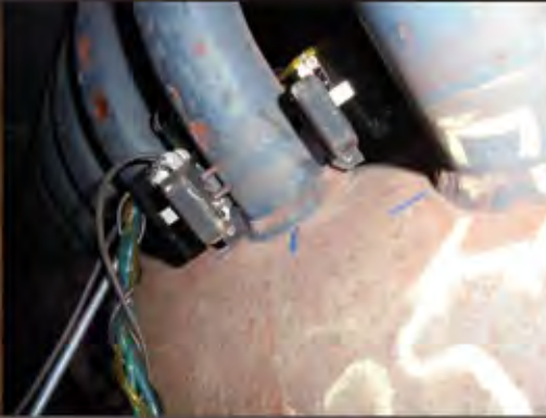
Tube to Header Weld Examination for Cracking
