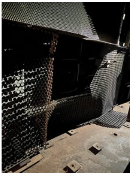
1. Careful design, robust framework, and heavy-gauge plate are required to prevent mechanical damage caused by the demanding environment downstream of the gas turbine
