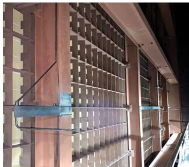
5. Periodic cleaning of catalyst (dirty at left, clean at right) is required to reduce performance-robbing pressure drop
