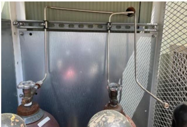
3. Bottles of inert gas are secured outside the shop (left); tubing brings the gas inside to the fixed manifold serving the welding machines (right)
