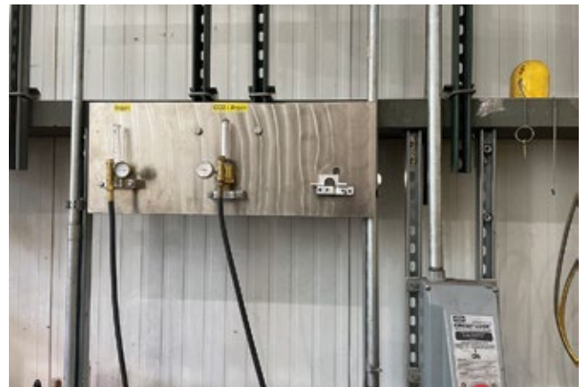
3. Bottles of inert gas are secured outside the shop (left); tubing brings the gas inside to the fixed manifold serving the welding machines (right)
