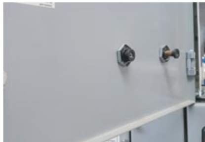
1. Pushbutton located outside motor starter, at left, is for resetting of the thermal overload; back side of the panel is at right
