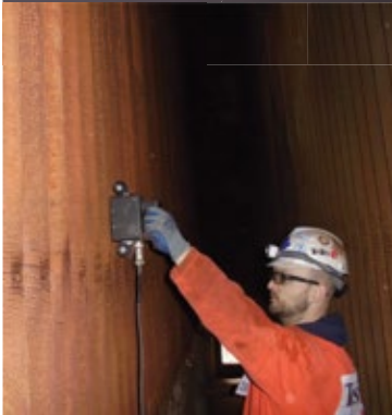
Through Fin Tube Scanning for Wall Thinning
