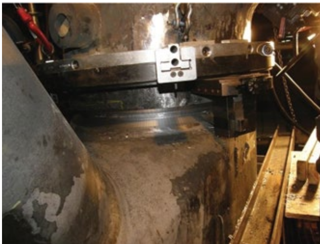
8. Creep-related failures may require full excavation of the damage (above)
