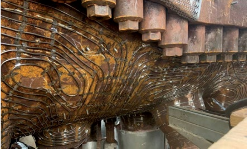
8. Permanent placement of redundant sets of heating wires on the turbine casing below the split line, plus the use of a heat-reflecting shield over the wires,
