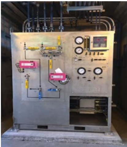
Environment One. Automated gas manifold H 2 monitoring system with automated purge-system options
