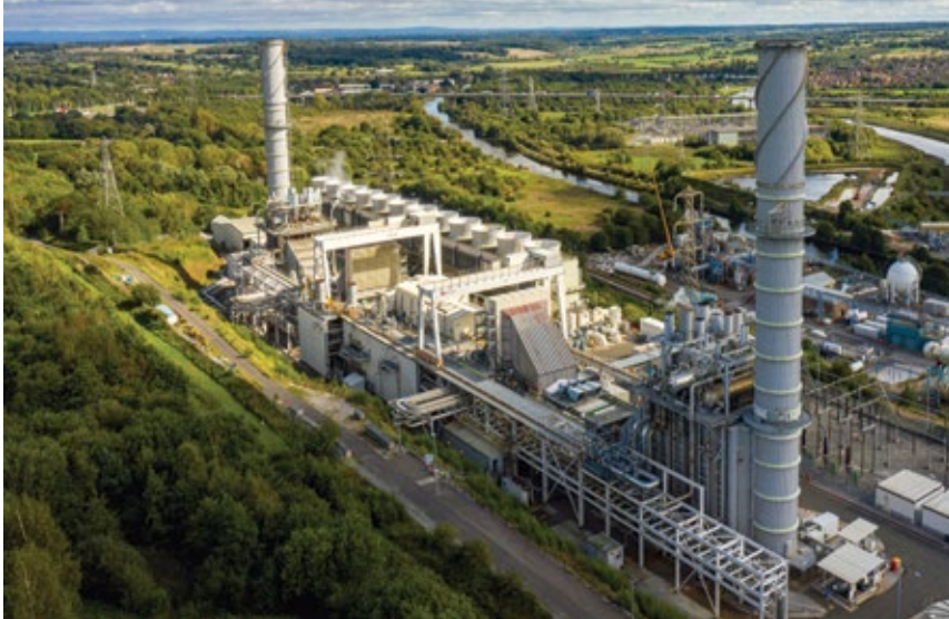
2. The UK's Rocksavage Power Station, near Liverpool, required a complete EV combustor rebuild on its GT26
