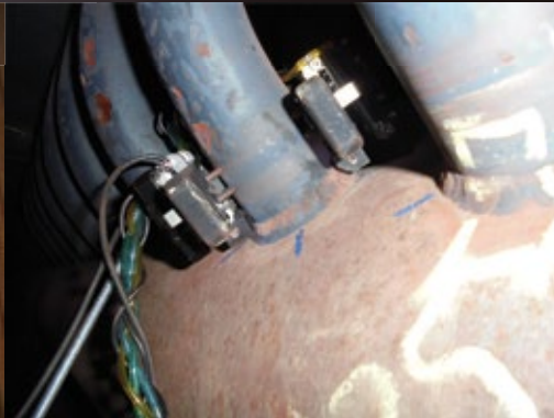
Tube to Header Weld Examination for Cracking
