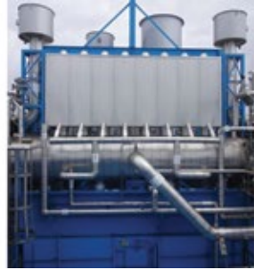
Secondary steam separation in bottles outside drum
