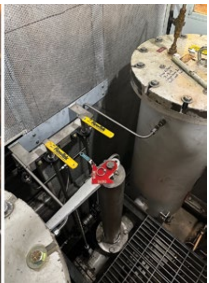
3. Newington’s duplex fuel filters, at left as installed, were modified to improve O&M access and safety (right)
