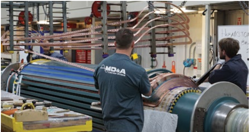
9. Hermiston's 7A6 generator-field rewind in progress at MD&A's repair facility
