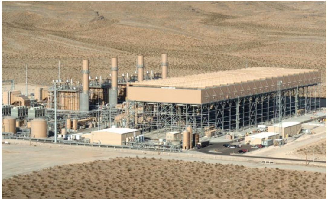
Lenzie was one of the largest combined cycles in the nation when completed in spring 2006. Its two 2 × 1 7FA-equipped power blocks share a common 100-cell air-cooled condenser, believed to be the largest in North America at the time
