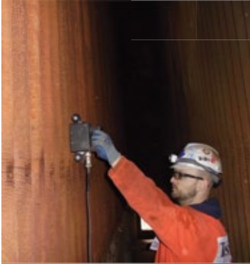
Through Fin Tube Scanning for Wall Thinning
