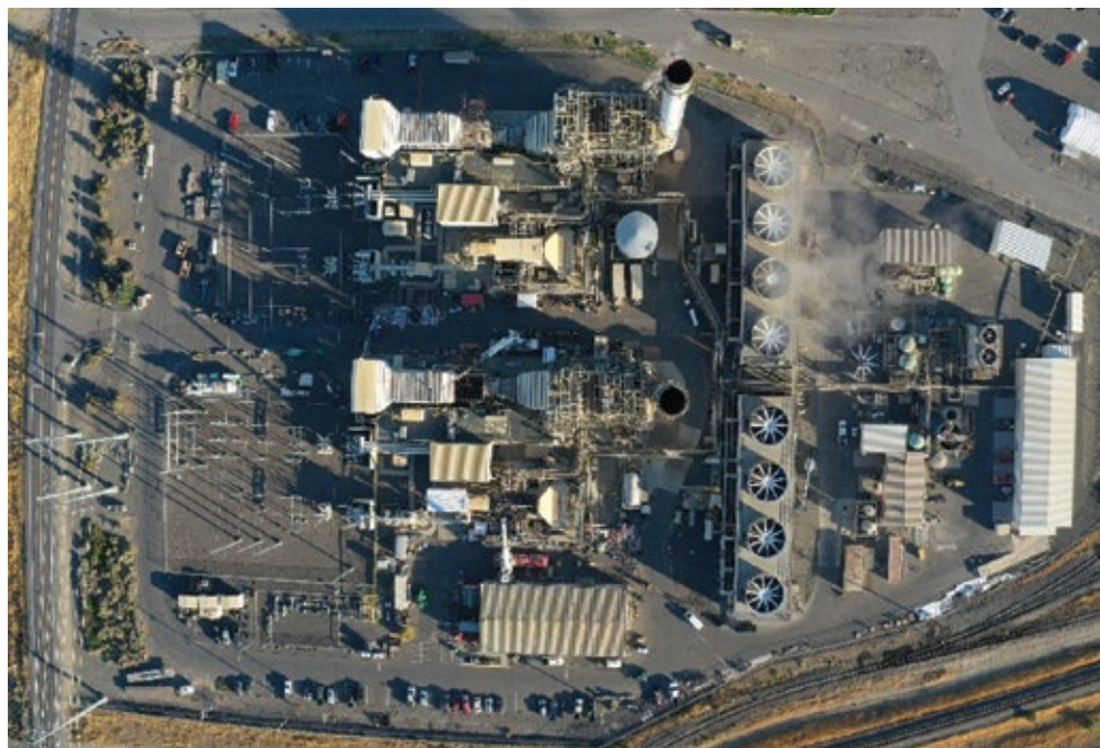
2. Limited space for contractors and equipment laydown was an added challenge in performing multiple majors
