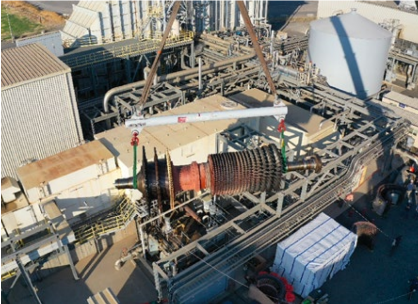
3. Team MD&A removes the 7FA gas-turbine rotor
