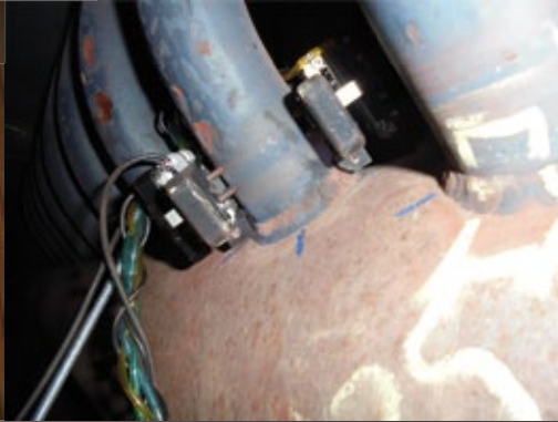
Tube to Header Weld Examination for Cracking
