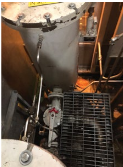
3. Newington’s duplex fuel filters, at left as installed, were modified to improve O&M access and safety (right)
