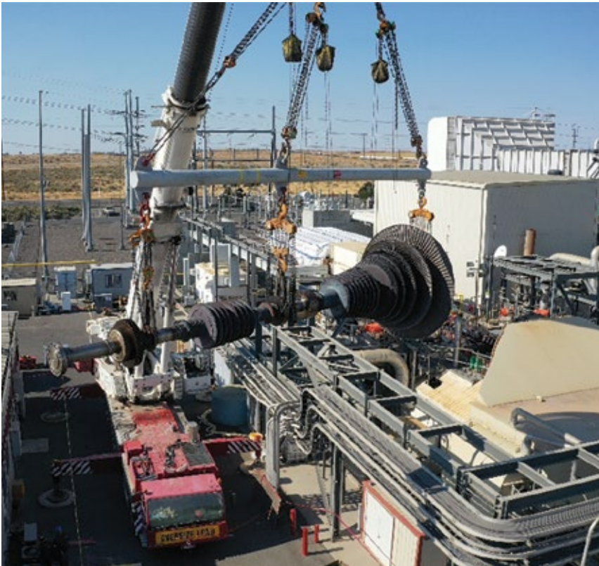
5. A10 steam-turbine rotor is removed for inspection and repairs
