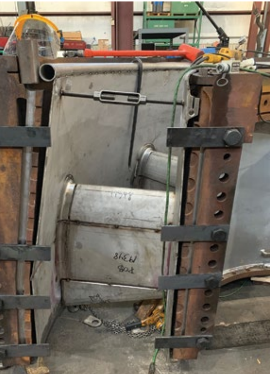
Exhaust refurbishment in the field
