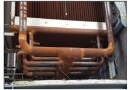
Multiple inside downcomers, expansion loops in evap feeder, and bundle spring support
