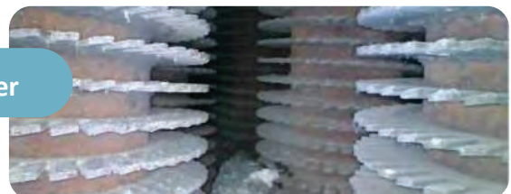
After cleaning 8th row of tubes
