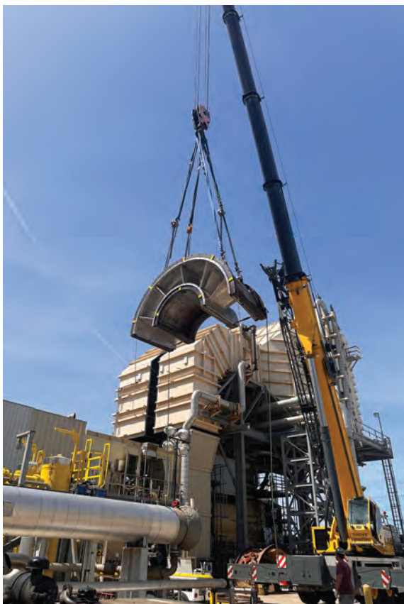
3. IPS field refurbishment was performed in less than 40 days and with the rotor in place
