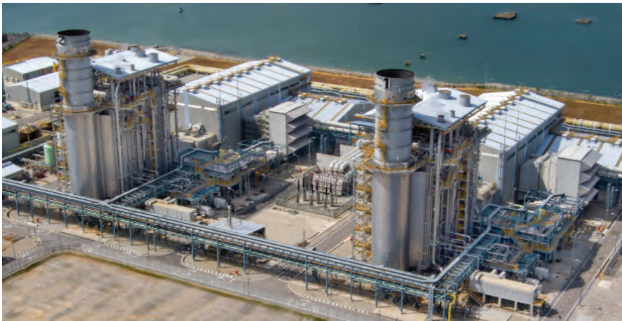
Track 4A in Malaysia, a 9HA.02, 2x1 CCGT with GE Vernova OT HRSGs
