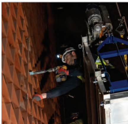
T3. Core sampling requires ladder or scaffolding for access
