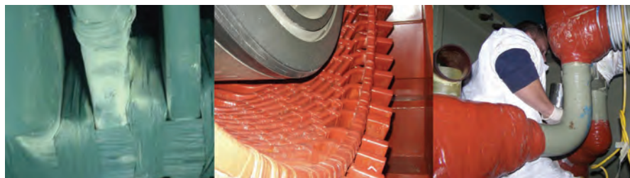
AGT Services: When robotic inspection is not feasible, borescope-aided visual inspection through simple end cover removal enables cost-effective access to critical generator components, including endwindings, main leads, and turn insulation
