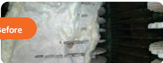
Before cleaning 8th row of tubes
