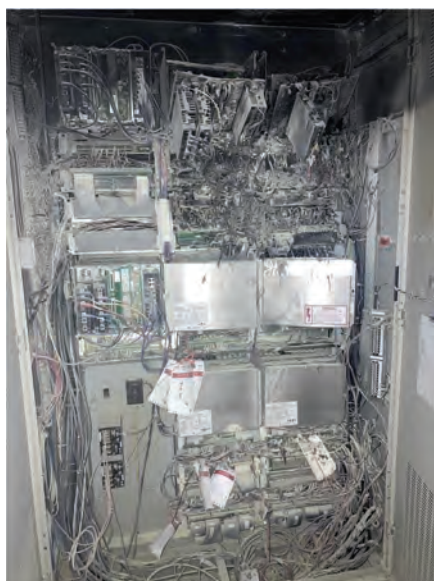
1. Recovery from fire in the charger cabinet, originating in the battery pack, was accomplished in two months
