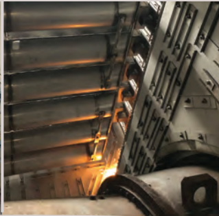
Exhaust Silencer Upgrades
