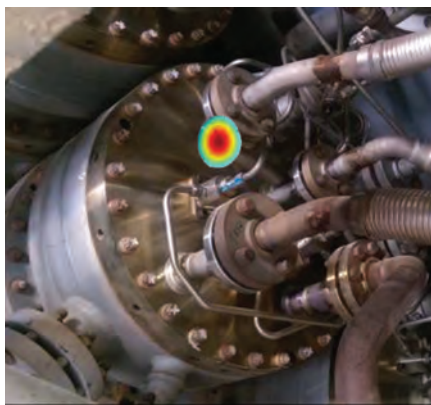
Detection of a fuel-gas leak is challenging after a major outage, given the scores of hoses and flanges to check (photo indicates a leak in the PM2 hose of one combustor). There are at least five ways to detect a fuel leak that you might consider
