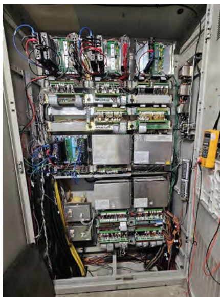
1. Recovery from fire in the charger cabinet, originating in the battery pack, was accomplished in two months
