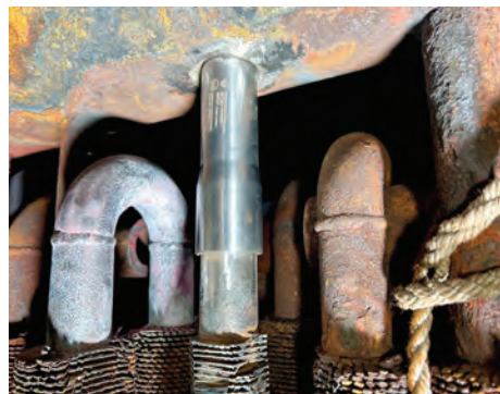
GS8. TTHC connection on location
