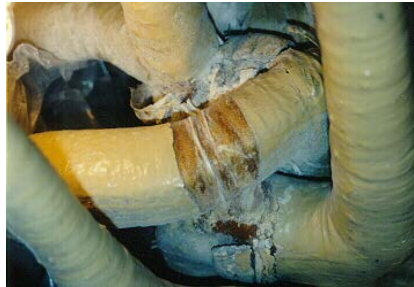
Figure 8-15. Replacing Individual Tie on Stator End Winding
