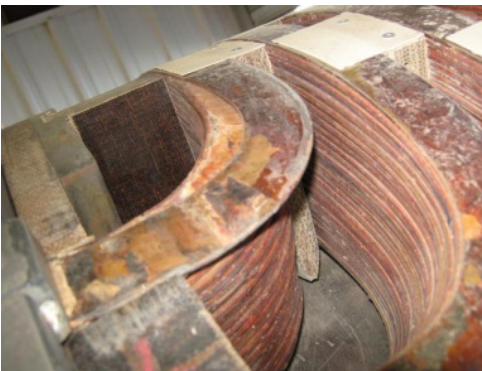
Photo 29. Badly distorted top turn on smallest coil.
