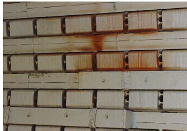
Figure 6-14. Dust Generated by Vibrating Wedges
