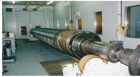
Figure 8-47. Closed Room with Controlled Atmosphere for Field Rewind
