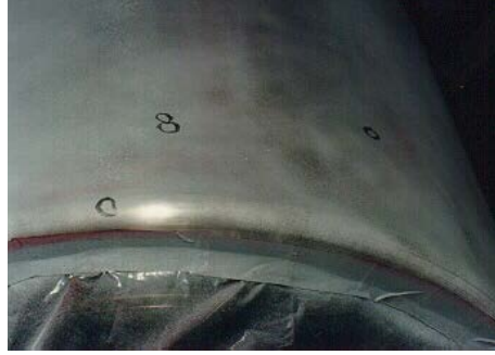
Figure 6-64. Retaining Ring with Minor Pitting Detected
