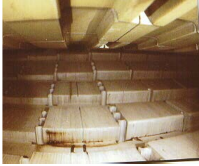
Figure 6-8 & Figure 6-9. Robot Camera View of Stator Bar Vibration and Core
