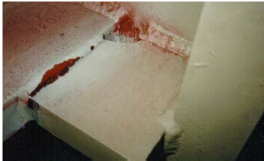
Figure 6-37. Inspection for Cracks in Generator Frame Structure
