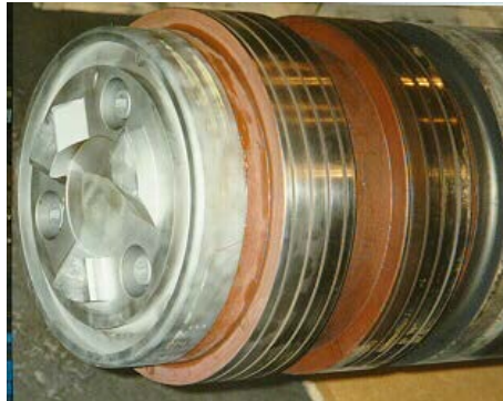
Figure 4-17. Contaminated and Rusted Collector
