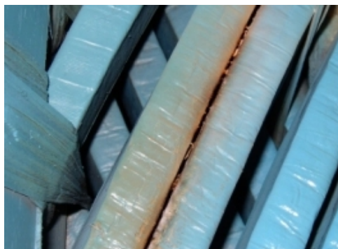
Photo 3. Significant surface partial discharge indication in the endwinding.
