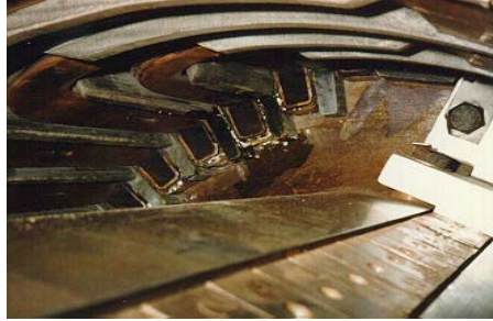
Figure 6-49. Inspection of Underside of Coils of Assembled Field
