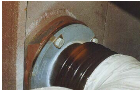
Figure 6-40. Standoff Insulator with Unbonded Flange
