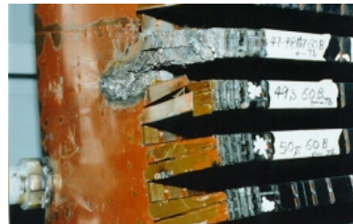
Figure 4-53. Extensive damage seen after partial disassembly of core
