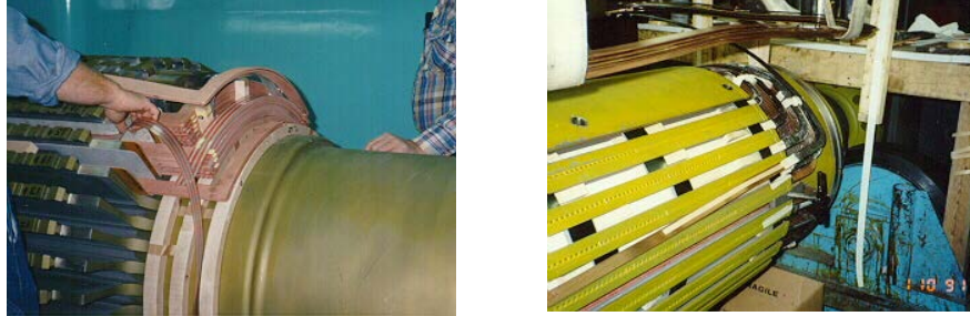
Figure 8-49 & Figure 8-50. Full Field Rewind in Progress
