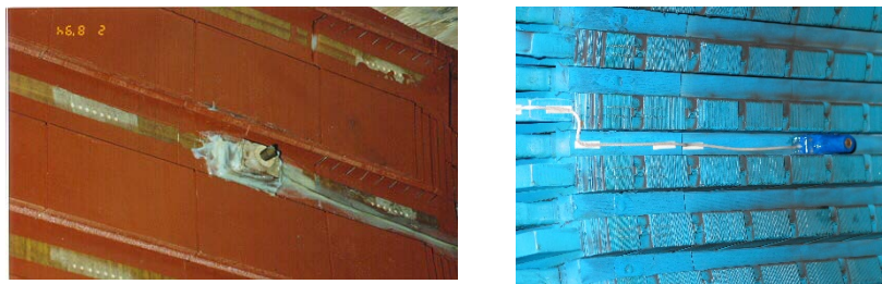
Figure 5-10 & Figure 5-11. Two Applications of Field Air Gap Flux Probes
