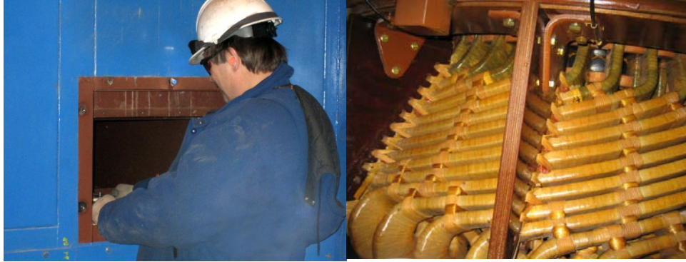
Figures 6-6a&b. Inspection Man-way in Frame Behind Stator Endwinding. Access to Winding through Man-way.
