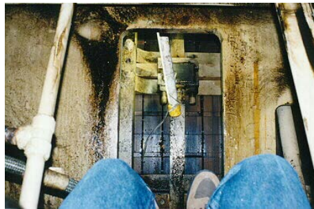
Figure 2-42. Opening Cut in Frame Wrapper Plate for Access
