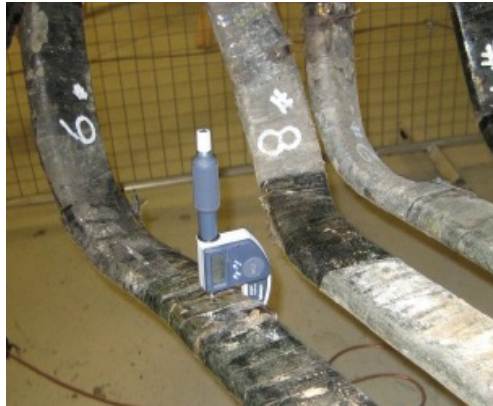
Figure 4-5b. Tape migration on a newer smaller generator.
