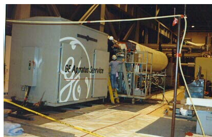
Figure 8-33 & Figure 8-34. Equipment for Removing Large 4-Pole Coupling
