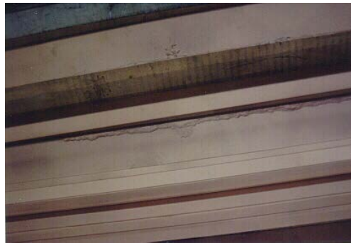
Figure 8-40. Field Forging Damage Due to Broken Field Turn
