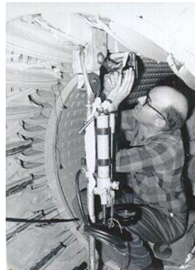
Figure 6-17 & Figure 6-18. Inspection for Stator Bar Slot Vibration by Borescope and Flashlight
