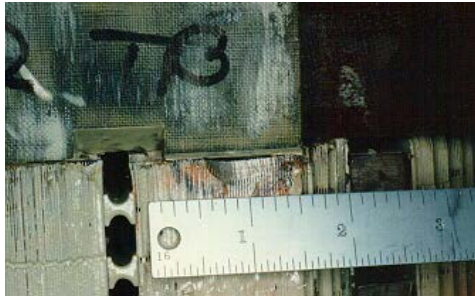
Figure 8-30. Repair of Minor Core Damage through Careful Grinding
