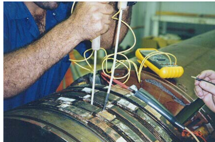
Figure 7-18. Checking Pole/Coil Voltages with Retaining Ring Removed
