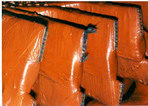
Figure 2-30. Westinghouse Taped Insulation on Gas Cooled Stator (after Service Failure and Insulation Damage)
