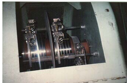
Figure 6-48. Collected Opened for Inspection
