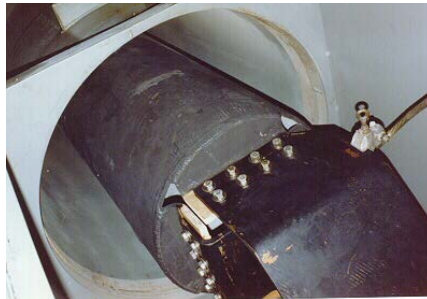
Figure 6-42 & Figure 6-43. Bolted Accessible Isophase Electrical Connection and Bolted Insulated High Voltage Bushing Connection
