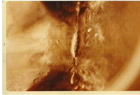
Figure 6-54. Distorted Borescope View of Crack in Main Lead Under Retaining Ring
