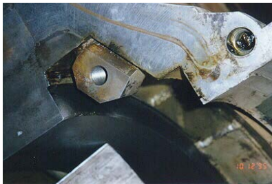
Figure 8-53. Addition Bolting on End Shield Horizontal Joint
