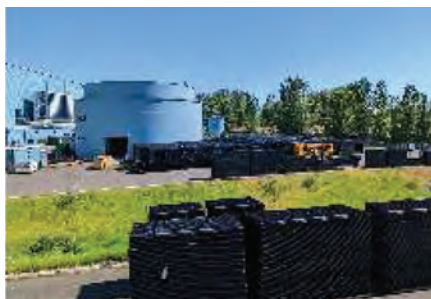
5. Media was replaced throughout the five-cell cooling tower
