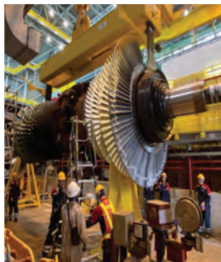
2. Trial lifts of critical components (GT rotor at left; exhaust casing at right) are an important part of pre-outage training
