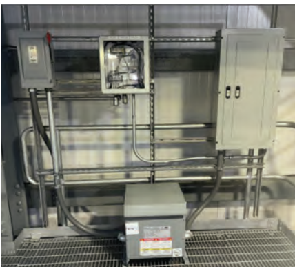
5. Electrical equipment to enable freeze protection included disconnect, step-down transformer, sub panel, and control panel
