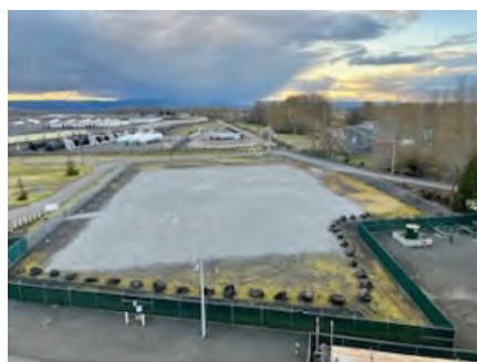
9. Unused lot next to the plant was converted to a parking area. One of the first steps was to compact its soft gravel surface
