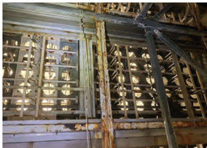
1. Evaporative cooler downstream framing before (left) and after (right) repair
