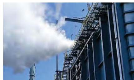
2. HP steam drum leak posed safety and reliability issues for a baseload 1x1 CCGT facility. Solution involved design and operating revisions
