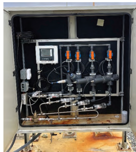
2. Upgraded influent sample panel provides better insight into water quality
