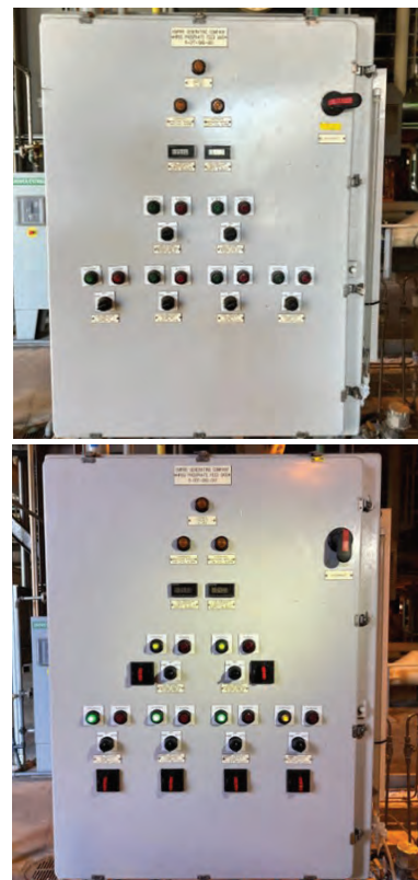
2. Original non-lockable, hand-off-auto switches at left, lockable disconnects alongside hand-off-auto switches at right
