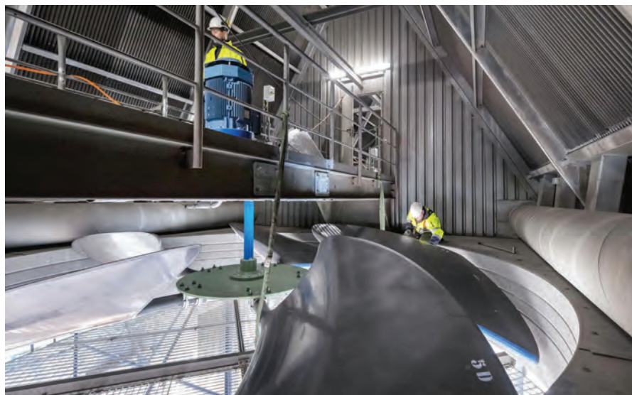
8. Completed installation Howden 6116SXT5
