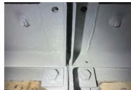
1. Evaporative cooler downstream framing before (left) and after (right) repair
