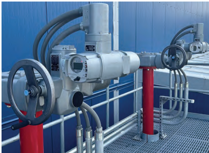
4, 5. Vibrations that compromised operation of valve actuators were mitigated by remote mounting of electronic controls (before/after are at the left/right, respectively)
