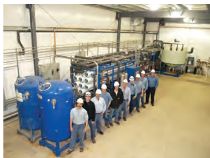
2. Trailers with ion-exchange vessels were replaced by a compact skid incorporating ultrafiltration and two-pass reverse osmosis systems
