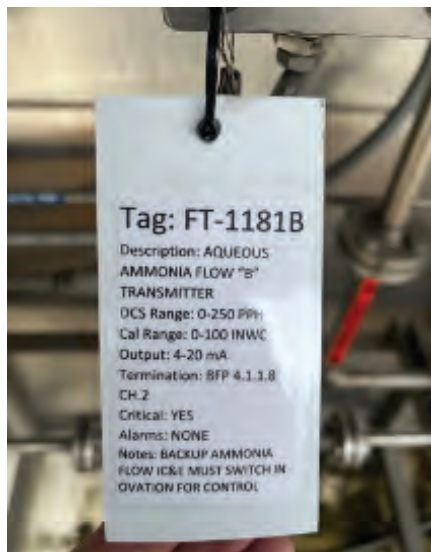
7. Pertinent information for a given instrument is displayed on its unique identification tag
