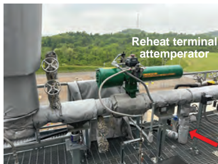
1. Attemperator systems are located in the upper-most pipe rack and exposed to low temperatures and high winds
