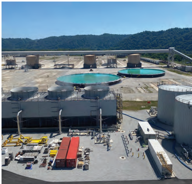
2, 3. Cooling water for Long Ridge is pulled from the Ohio River, treated, and retained in two ponds that serve the cooling tower
