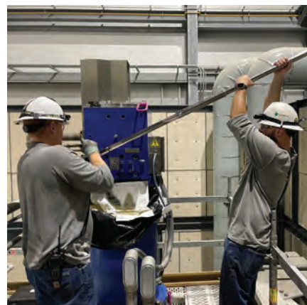
3. Plant personnel remove and clean the trip-oil poppet valve
