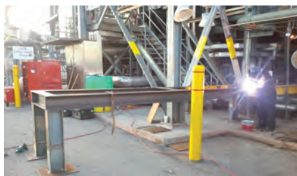
4. Steel support and trolley system had to be installed to slide reheater attemperator out from under the HRSG
