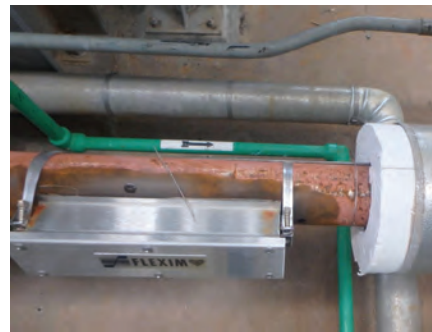
6. Ultrasonic flowmeter, clamped onto an attemperator spray water line, was able to detect leakage and avoid boiler tube damage. Device is suitable for challenging plant locations when existing flow detection isn’t working well
