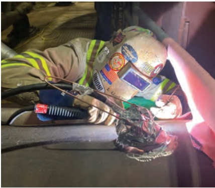
4. Welding of 2-in. P22 Latrolet fitting for tie-in to existing steam-turbine drains-tank line
