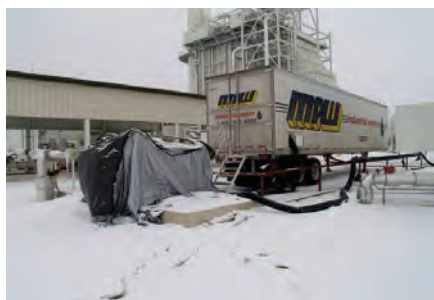
1. Ion-exchange trailers were specified for Faribault because of restrictions on the discharge of wastewater from an RO system. However, they posed operational challenges
