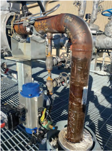
3. Installation of ½-in. leak-off line into attemperator supply line
