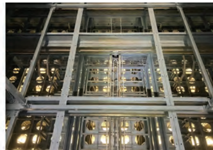
1. Evaporative cooler downstream framing before (left) and after (right) repair
