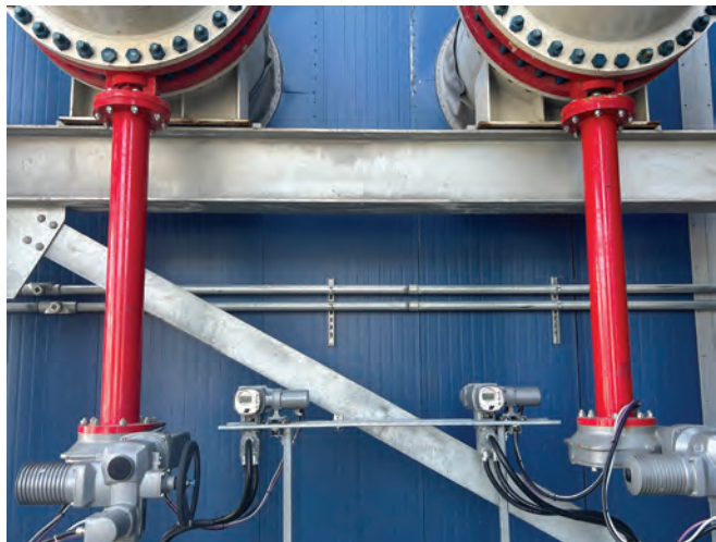
4, 5. Vibrations that compromised operation of valve actuators were mitigated by remote mounting of electronic controls (before/after are at the left/right, respectively)
