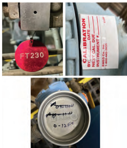
6. Multiple versions of RRGP instrument tags were converted to a standard format, enabling quick and concise bidirectional communication between the field and control room
