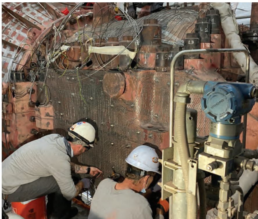
Heater cables installed along mapped grid to ensure uniform heat distribution before applying insulation screens and cladding
