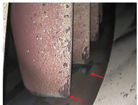
R2 blade damage prompted inclusion of spare components in project budget and proactive preparation for future parts fallout
