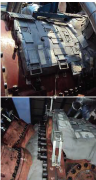
Arnold Group. Thoughtfully designed insulation blankets enable partial removal, allowing 60–80% to remain installed during outages, cutting reinstallation time
