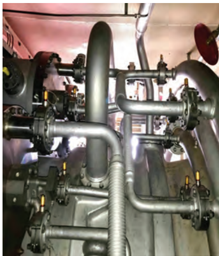
HP Leak Detection. Installed flange leak detection system uses pressure-activated flags to pinpoint flange leaks during operation, improving safety and minimizing downtime
