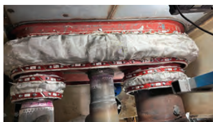
8. Combination side wall penetration seal for cyclic duty
