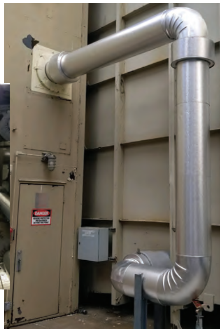
Single-piece exhaust section lowered into place using swing set hangers to improve alignment and ease of installation
