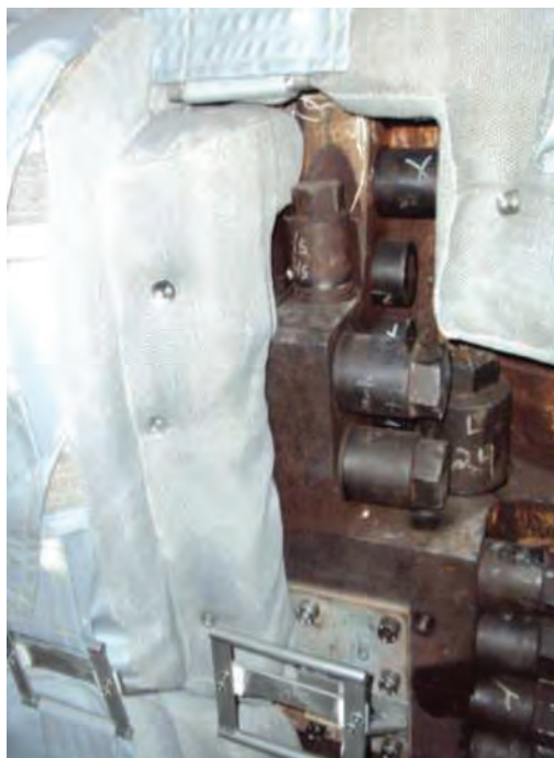
Arnold Group. Thoughtfully designed insulation blankets enable partial removal, allowing 60–80% to remain installed during outages, cutting reinstallation time
