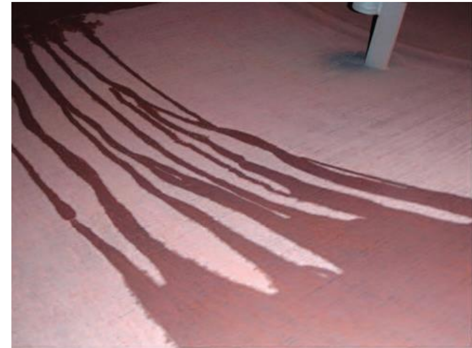
Feedwater tank of a CHP Plant during shutdown inspection (Systems treated with FFA and emptied)
