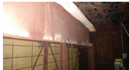
3. Pillow seals can help prevent bypass around SCR catalyst frame
