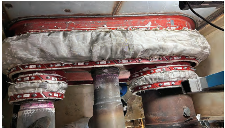
6. DEKOMTE combination seal
