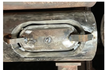
8. Final repair method Unit 12
