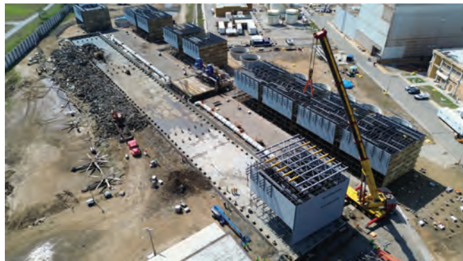
3. Cooling tower replacement progresses (right) after demolition of the original wood structure (left)
