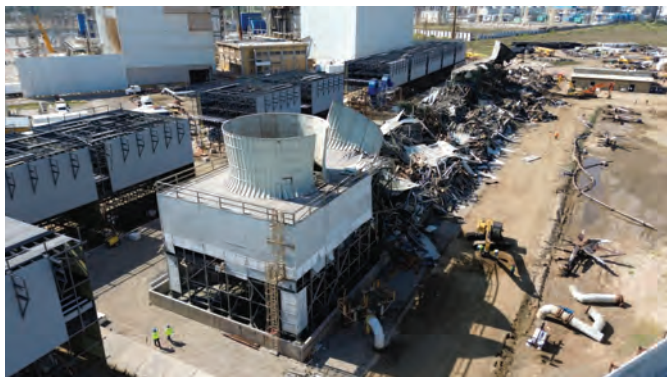
3. Cooling tower replacement progresses (right) after demolition of the original wood structure (left)
