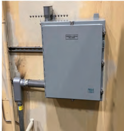
2. Cabinet photos show the transition from bulky dual purge boxes to a cleaner CDMS kit that consolidates signal conditioning and simplifies installation
