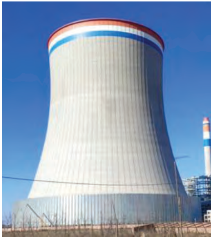
2. Dry cooling tower at GaoHe 1320 MW thermal power plant
