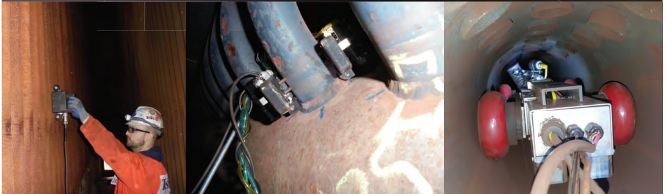
Through Fin Tube Scanning for Wall Thinning
