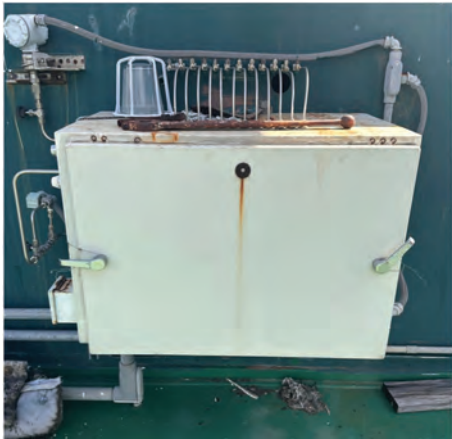
2. Cabinet photos show the transition from bulky dual purge boxes to a cleaner CDMS kit that consolidates signal conditioning and simplifies installation
