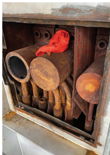
11. Penthouse sidewall removal for HP evaporator rear header inspection
