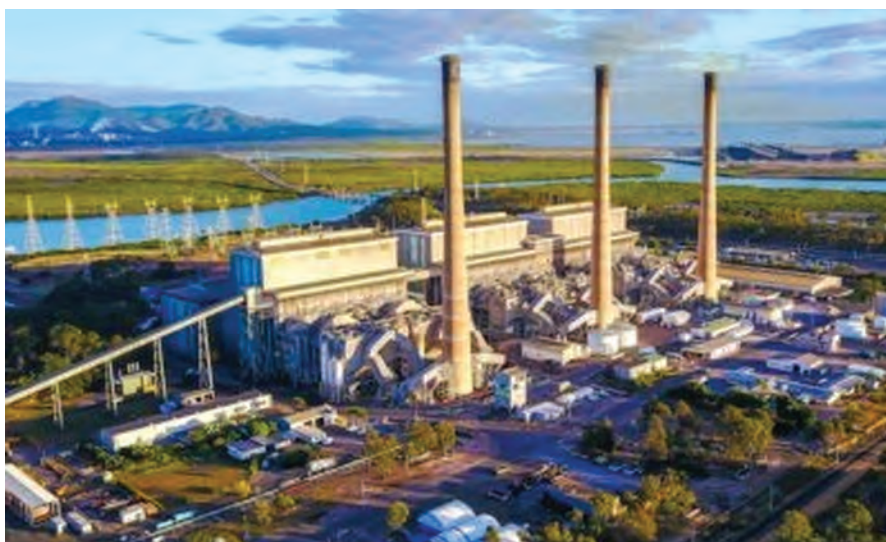
1. 1680 MW NRG Gladstone Power Station, Queensland
