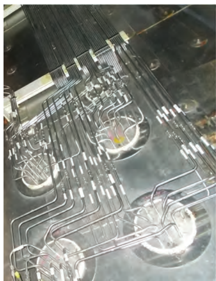
4. Data from sampling/tuning grid installed on the downstream side of the SCR catalyst in horizontal HRSGs is used to create heat maps for adjusting AIG balancing valves, reduce ammonia consumption, and minimize outlet NOx based on average and localized values
