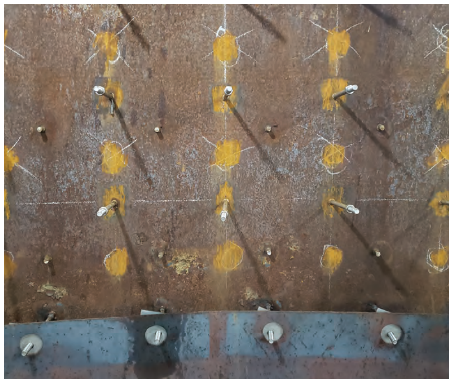
1. Exhaust-casing wall prepared for liner repair
