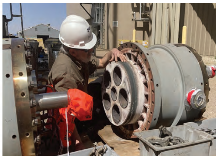
1. White powder discovered on combustion-system components during the outage was identified by laboratory analysis as sodium sulfate, providing the first clue to the source of the turbine’s hot-corrosion problem
