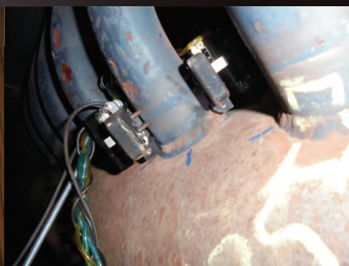
Tube to Header Weld Examination for Cracking
