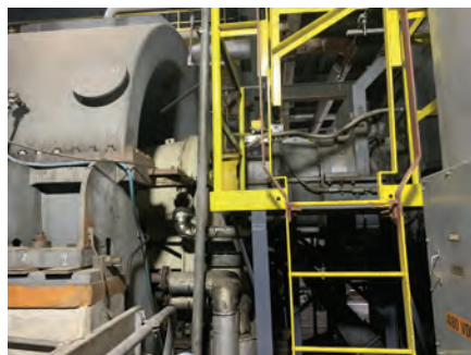
7. The SSS Clutch is the cream casing on the left, with a Brush generator on the right
